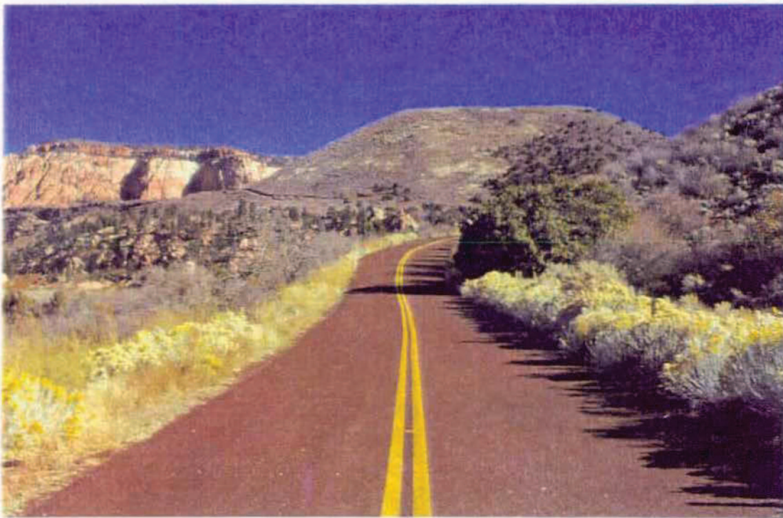
Photo #400 - MP 0.00 - Begin North Section, Typical Pavement Section
