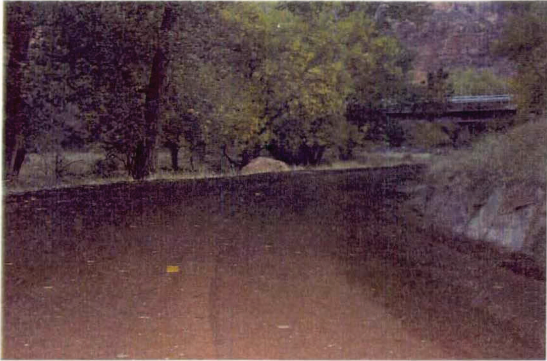
Photo #53 - MP 0.00 - Typical Pavement Section
