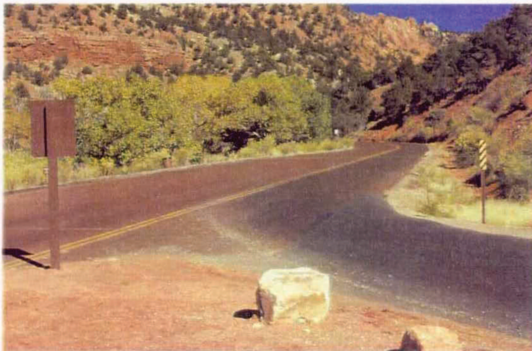
Photo #31 - MP 0.04 - Typical Pavement Change
