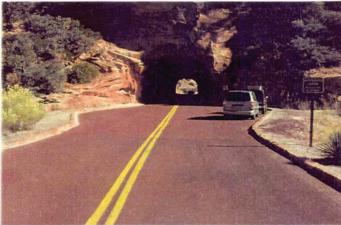
Photo #22 - MP 7.35 - Tunnel entrance
