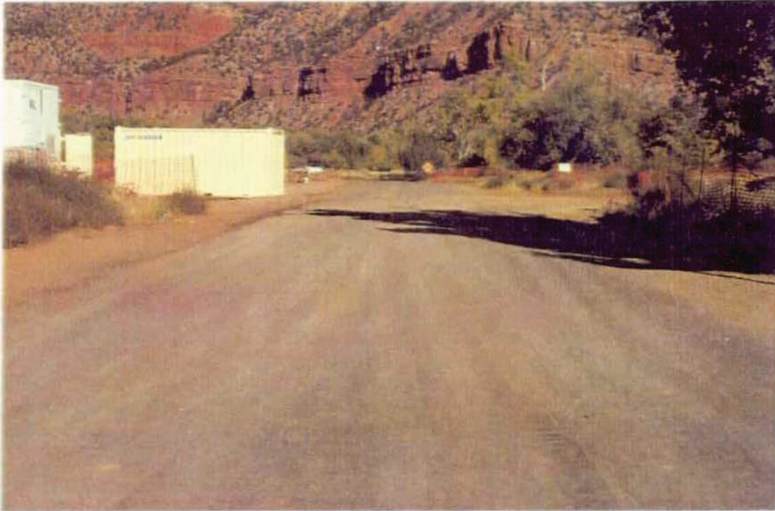
Photo #36 - MP 0.00 - Typical Pavement Section
