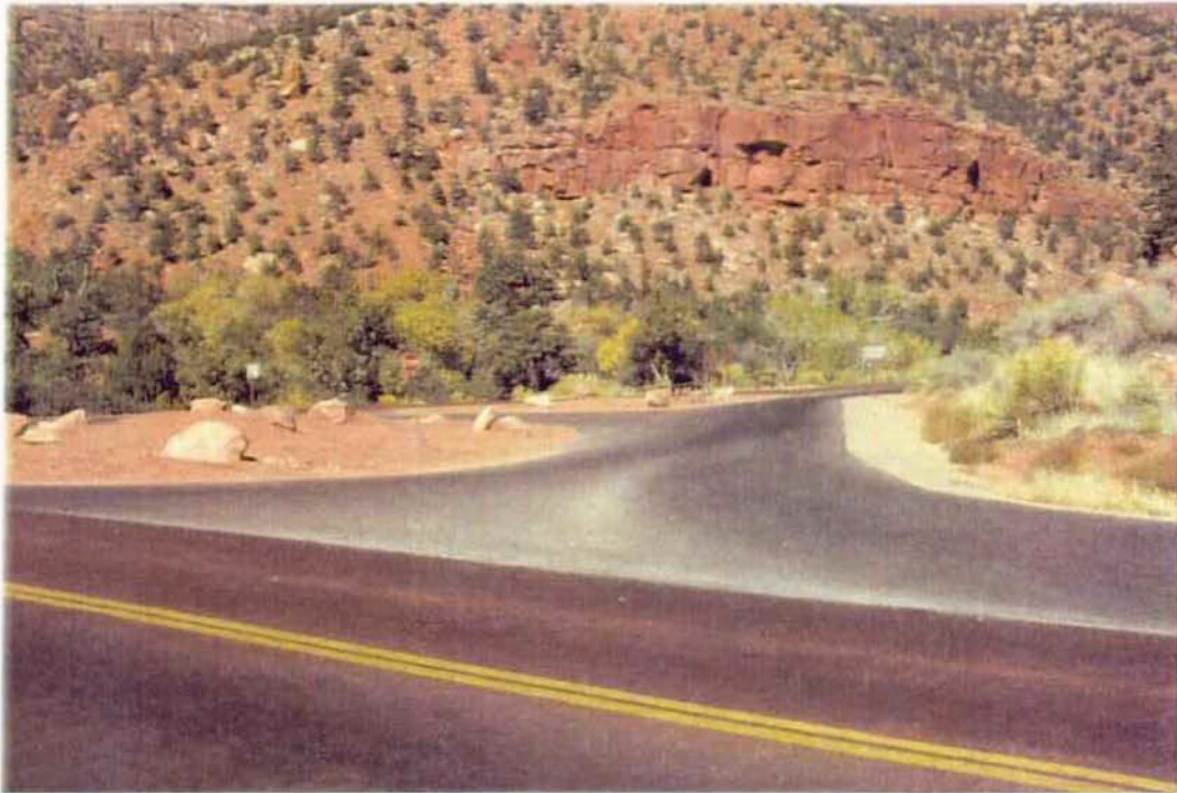
Photo #30 - MP 0.00 - Begin at Rte 010, Typical Pavement Section
