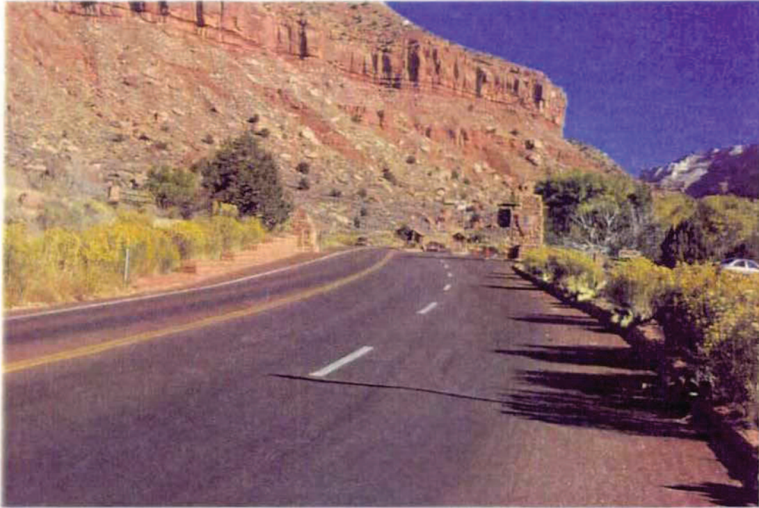
Photo #14 - MP 0.00 South Entrance - Typical Pavement Section
