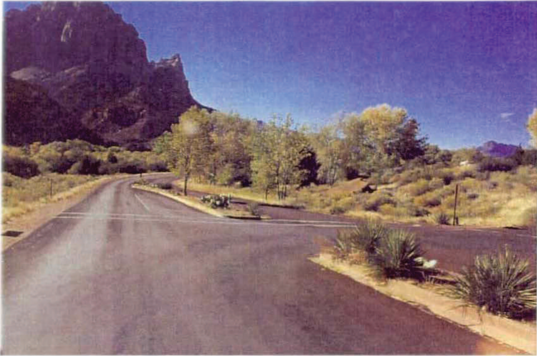
Photo #16 - MP 0.89 - Typical Pavement Section
