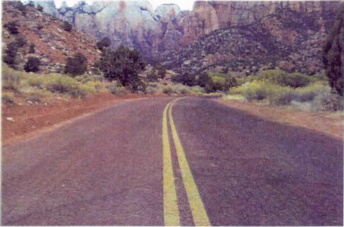
Photo #50 - MP 0.05 - Typical Pavement Section
