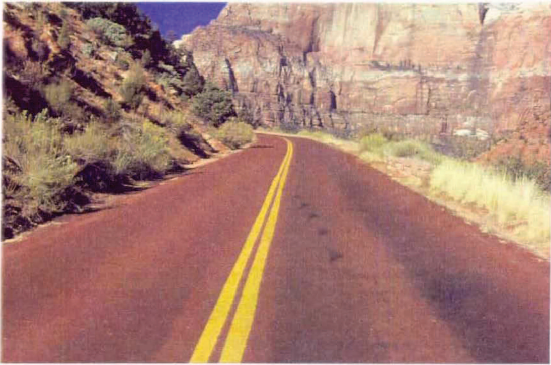
Photo #18 - MP 3.30 - Pavement Change
