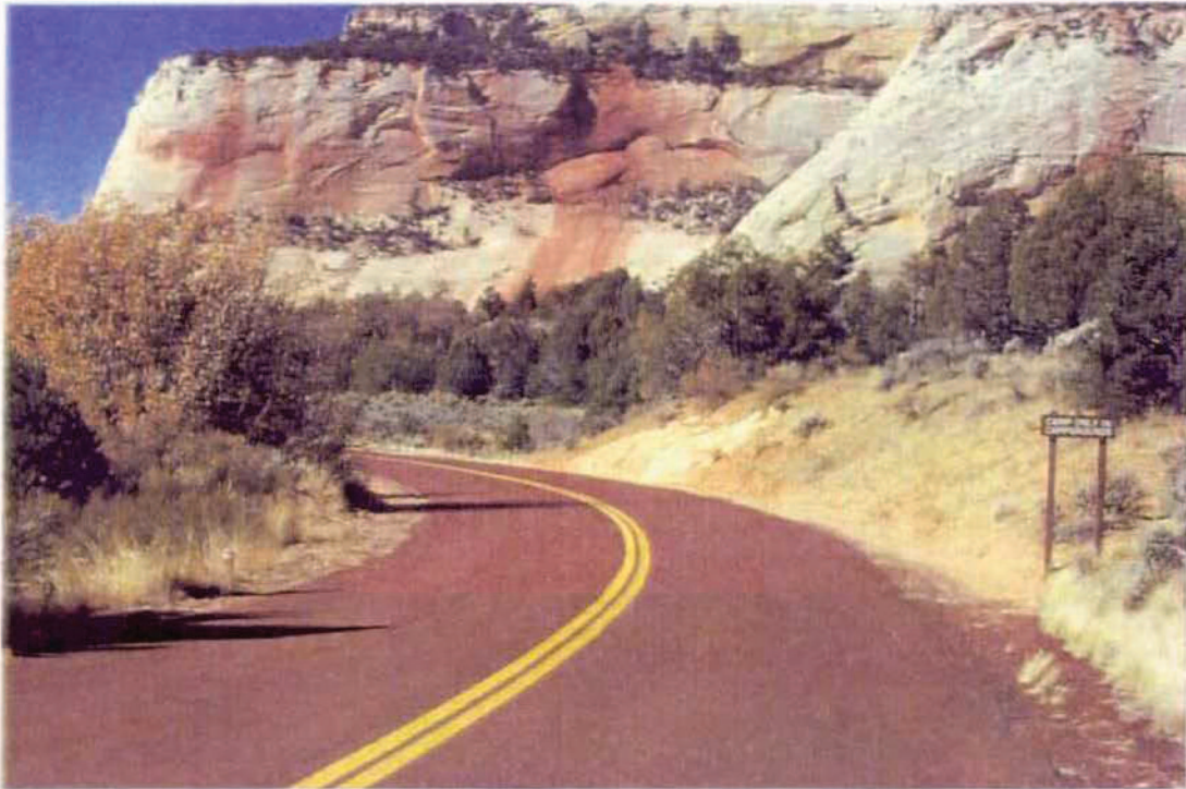
Photo #24 - MP 11.55 - Typical Pavement Section, looking back
