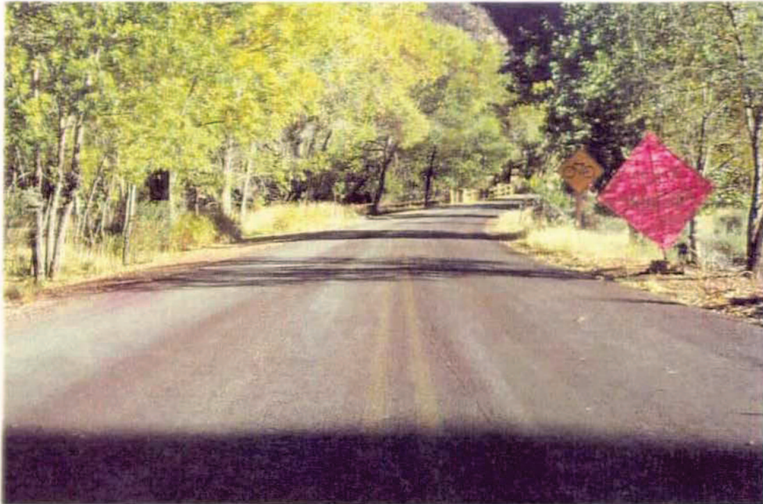
Photo #42 - MP 0.00 - Typical Pavement Section
