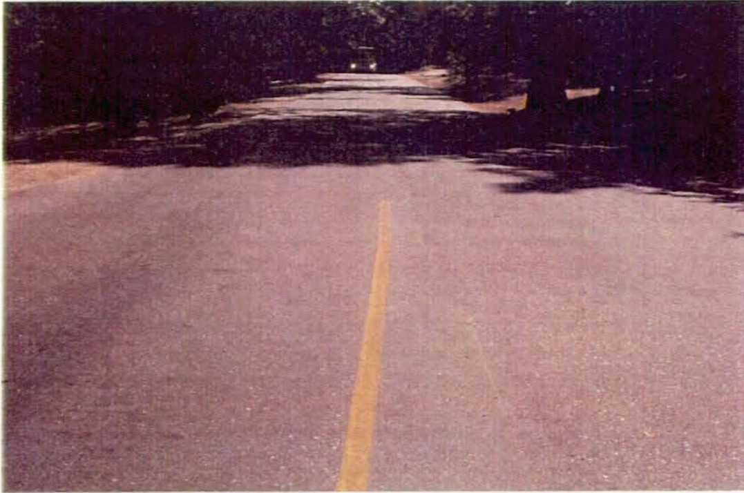
Photo #3465 - MP 0.00 - Begin at Rte 206, Typical Pavement Section
