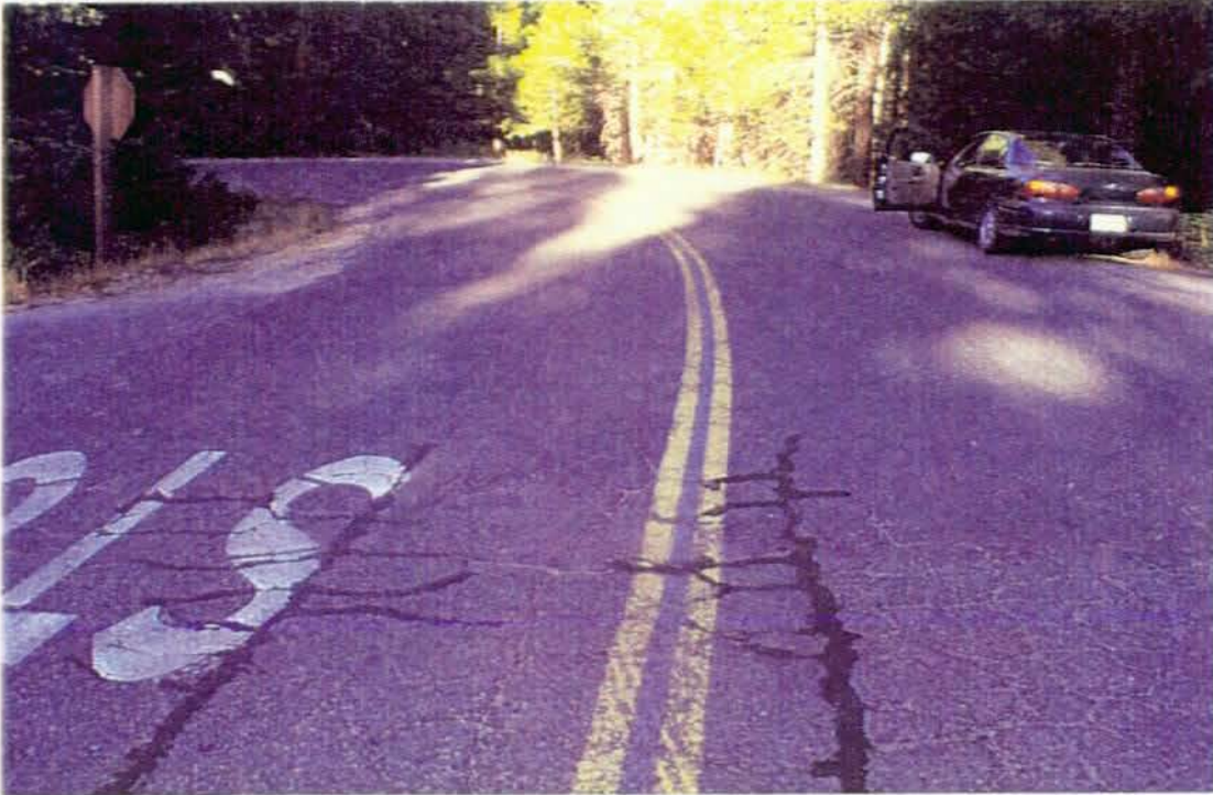
Photo # 3459 - MP 0.00 - Begin at Rte 013, Typical Pavement Section
