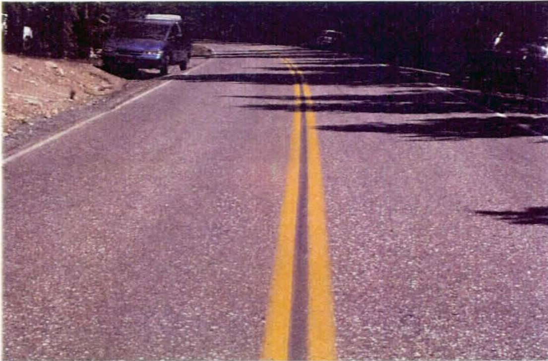
Photo #3472 - MP 35.86 - Typical Pavement Section
