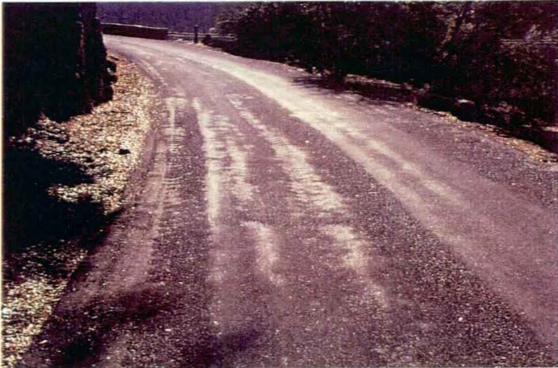
Photo #3458 - MP 0.10 - Typical Pavement Section
