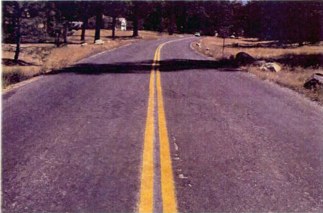
Photo #3441 - MP 0.00 - Begin at Rte 014, Typical Pavement Section
