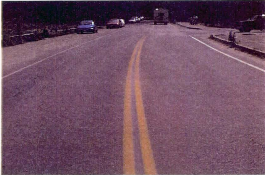
Photo #3464 - MP 0.10 - Typical Pavement Section
