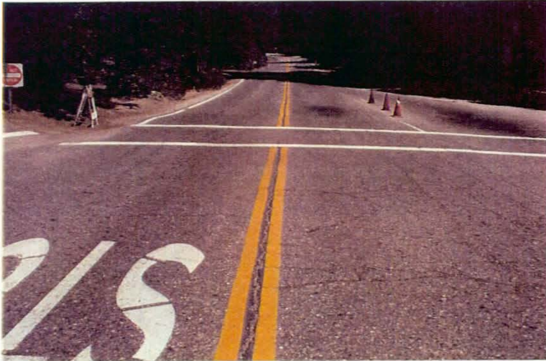
Photo #3448 - MP 0.03 - Typical Pavement Section.
