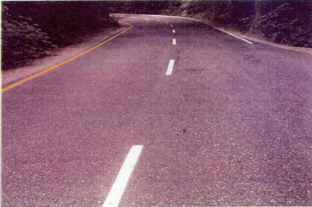
Photo #3460 - MP 0.12 - Typical Pavement Section
