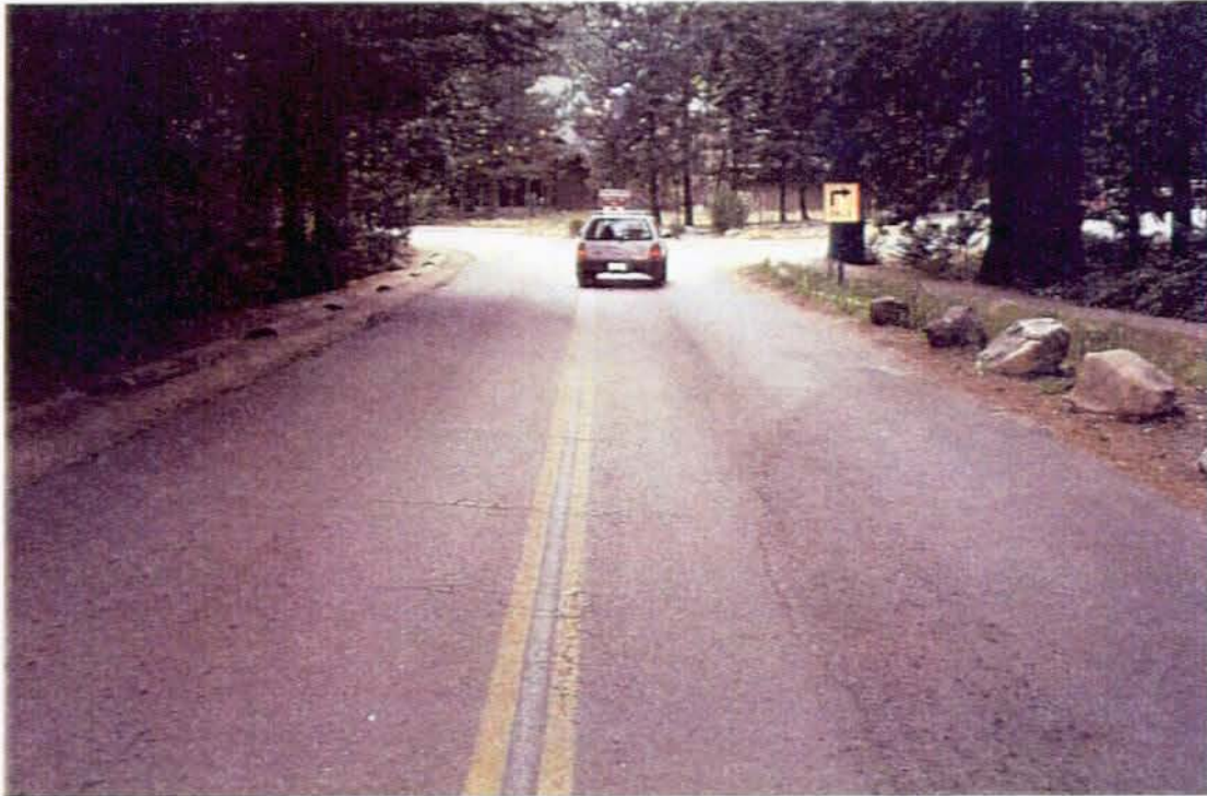
Photo #3479 - MP 0.02 - Typical Pavement Section
