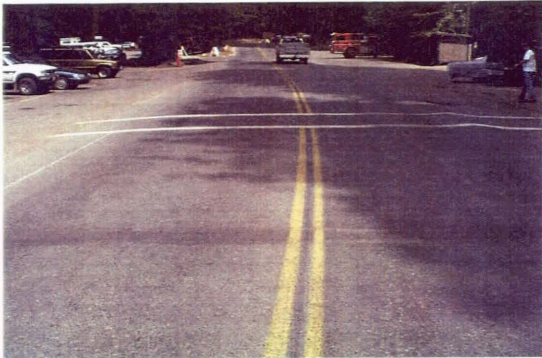
Photo #3469 - MP 0.07 - Typical Pavement Section
