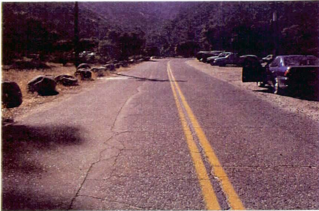
Photo #3438 - MP 0.15 - Typical Pavement Section
