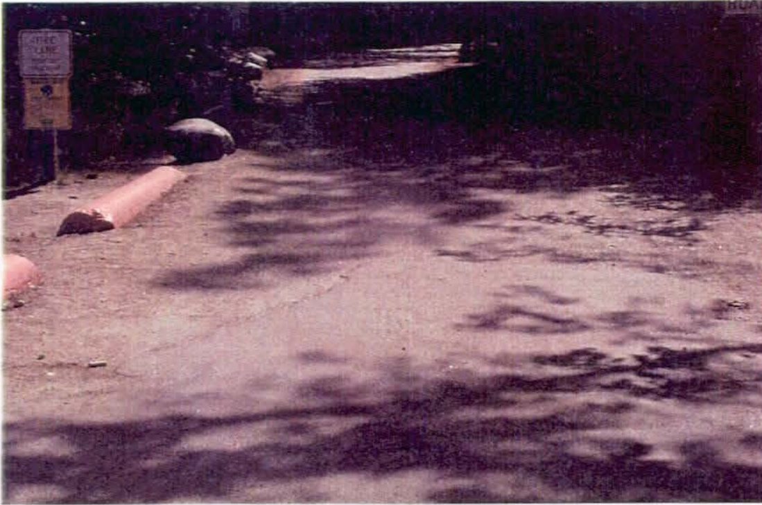
Photo #3462 - MP 0.00 - Begin at Rte 954
