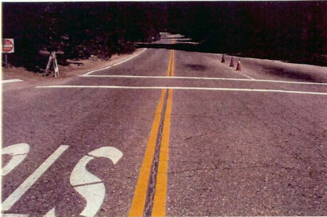
Photo #3448 - MP 0.03 - Typical Pavement Section.
