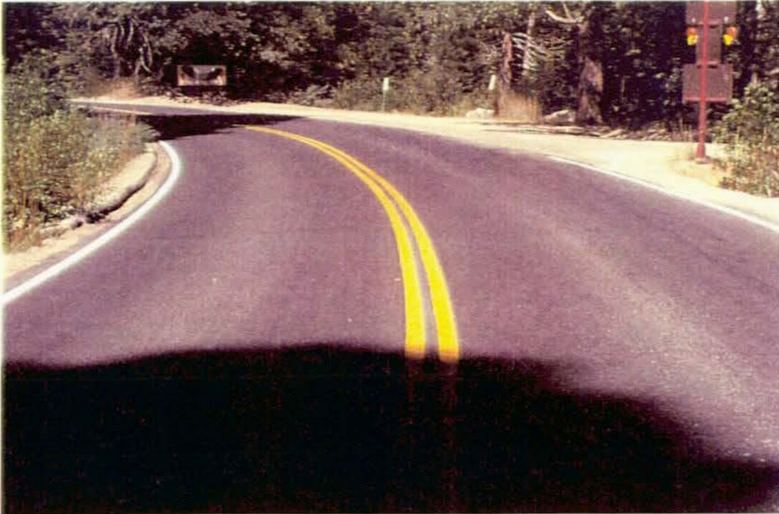
Photo #3449 - MP 0.03 - Typical Pavement Section
