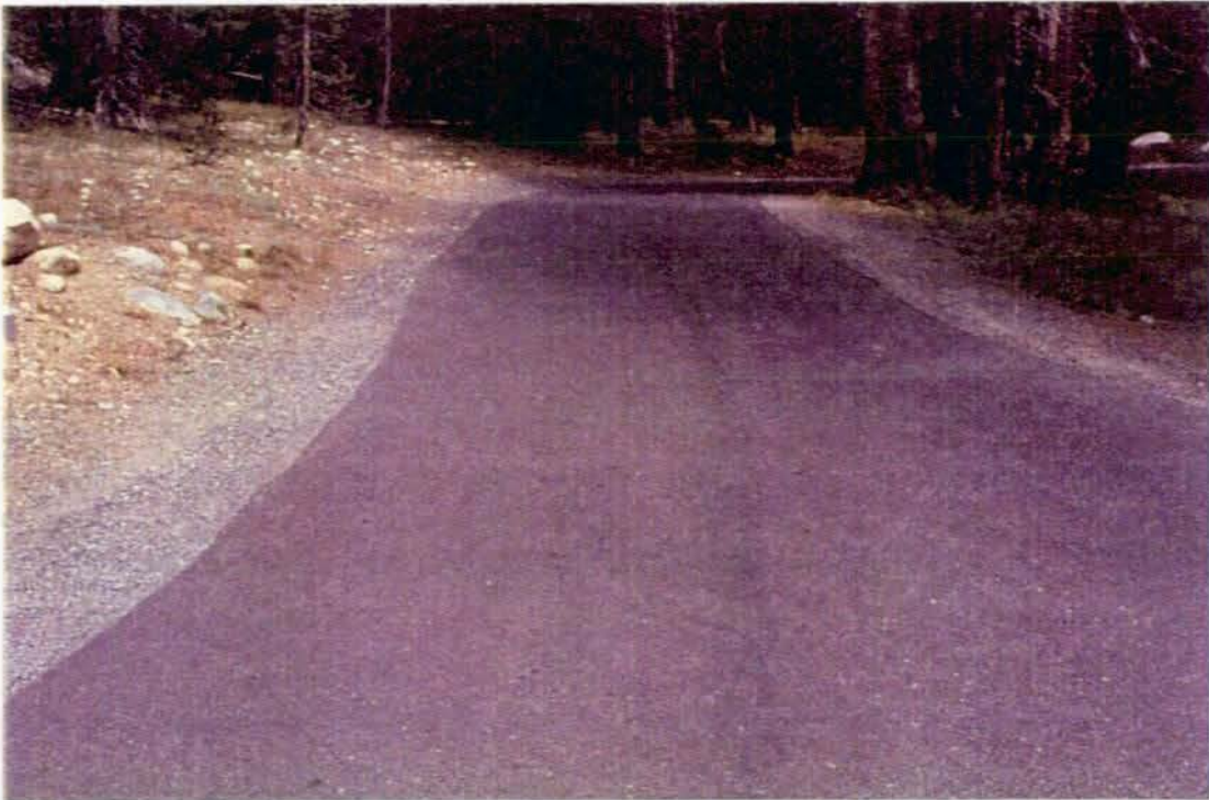
Photo #3475 - MP 0.50 - Pavement Change
