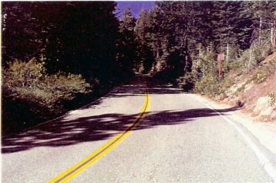
Photo #3434- MP 0.02 - Typical Pavement Section
