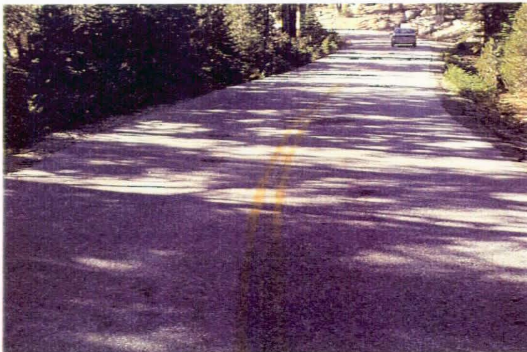
Photo #3476 - MP 0.00 - Begin at Rte 017
