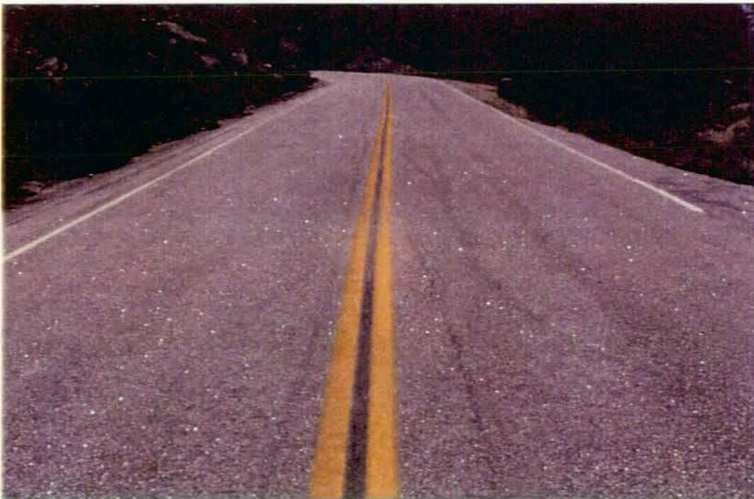
Photo #3471 - MP 20.30 - Typical Pavement Section
