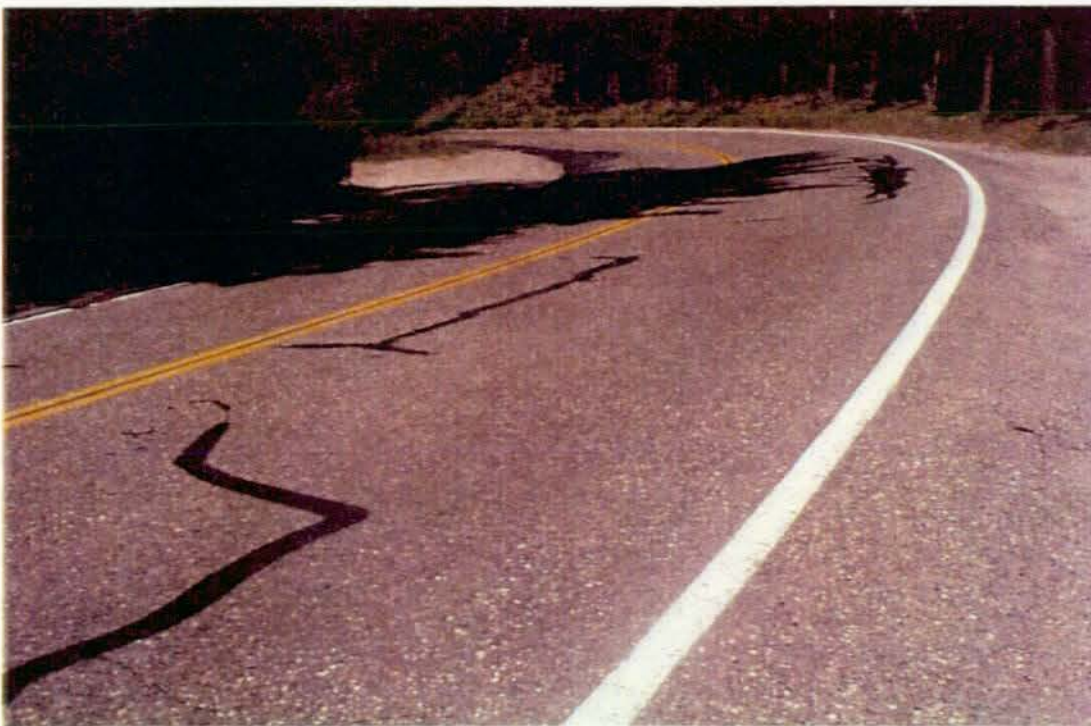
Photo #3450 - MP 17.80 - Typical Pavement Section, with sealed cracks.
