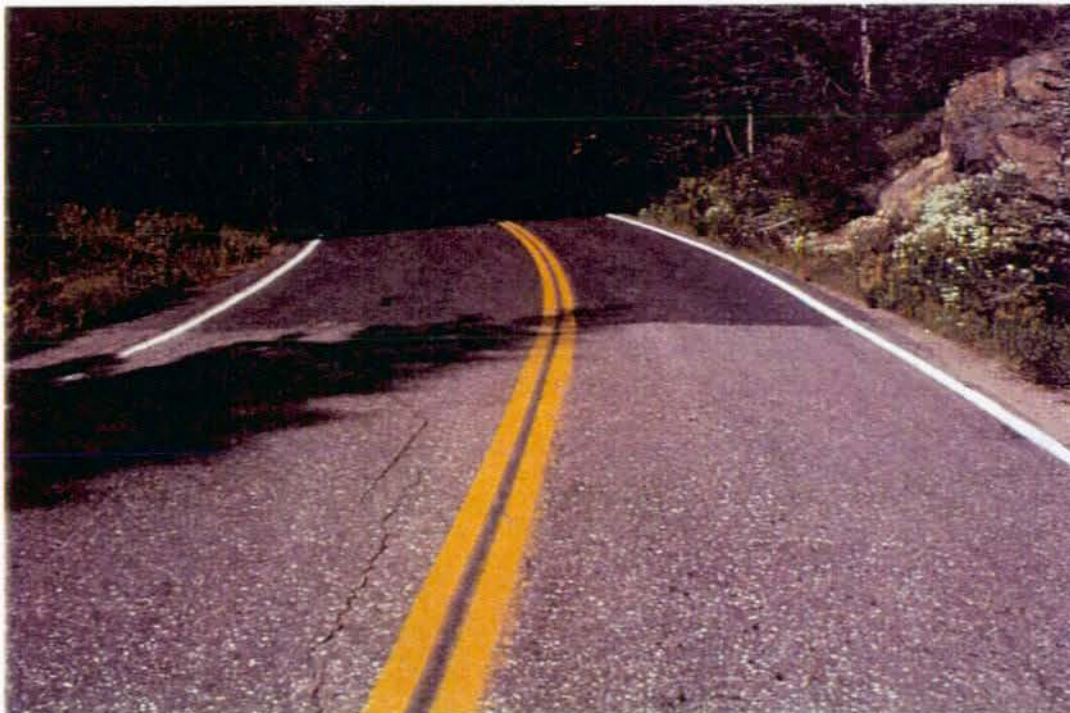
Photo #3450 - MP 5.02 - Pavement Change to new asphalt
