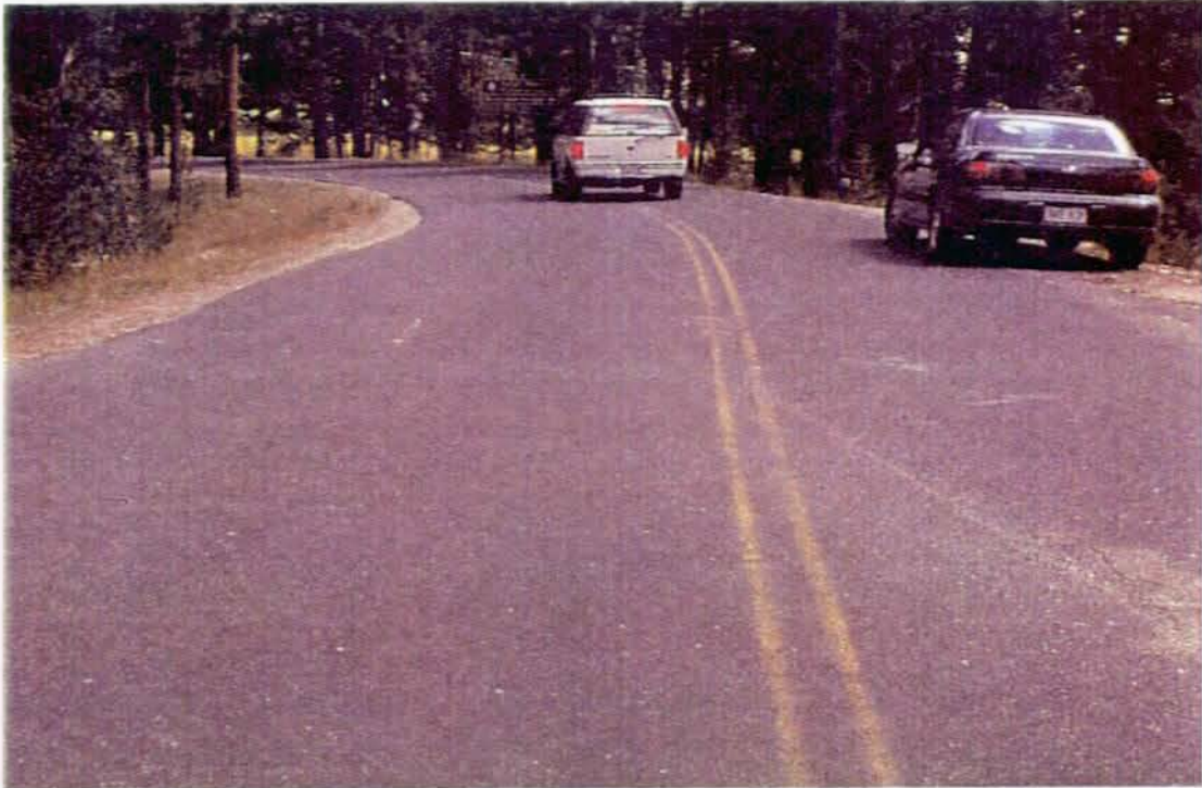
Photo #3474 - MP 0.02 - Typical Pavement Section
