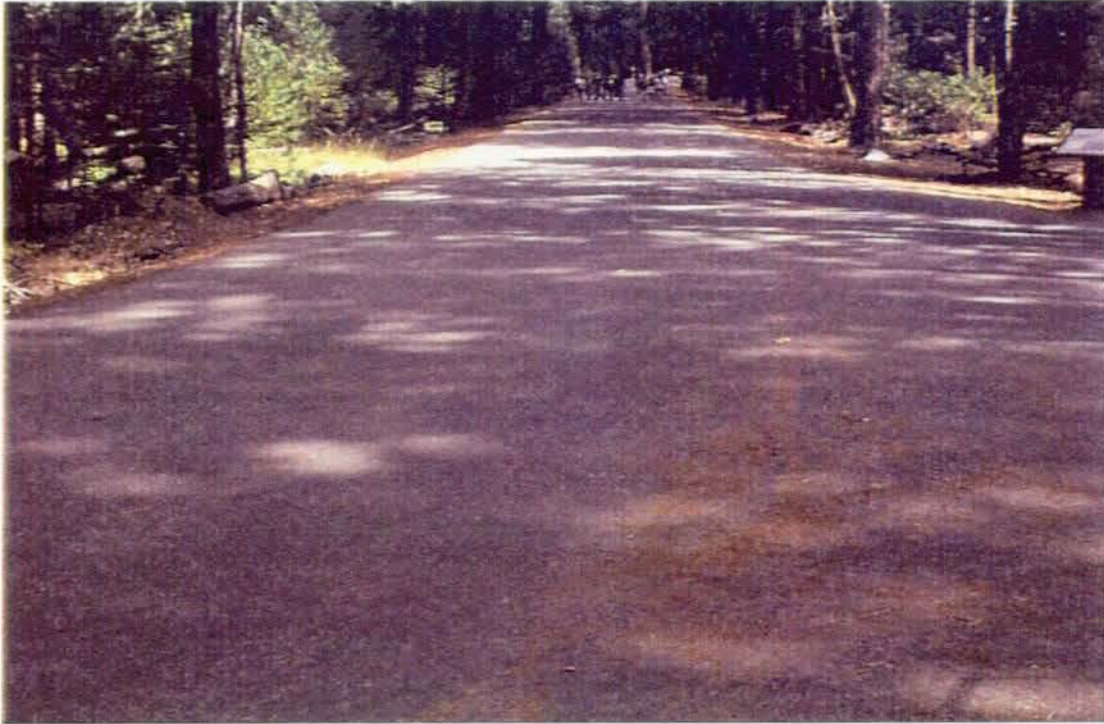
Photo #3468 - MP 0.00 - Begin at Rte 408, Typical Pavement Section
