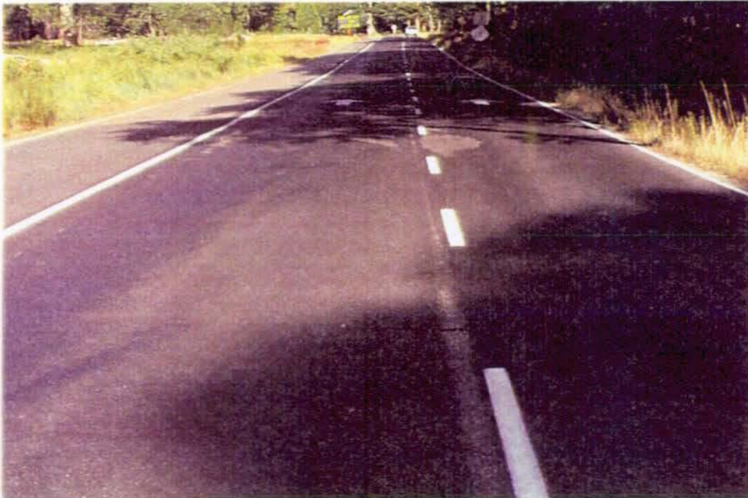
Photo #3461 - MP 10.64 - Typical Pavement Section
