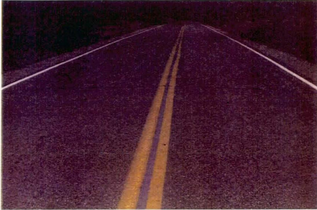
Photo #3480 - MP 0.08 - Typical Pavement Section
