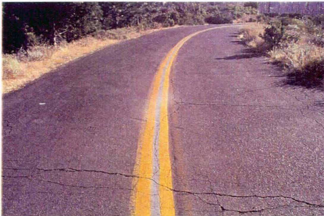
Photo #3477 - MP 0.00 - Begin at Rte 013, Typical Pavement Section
