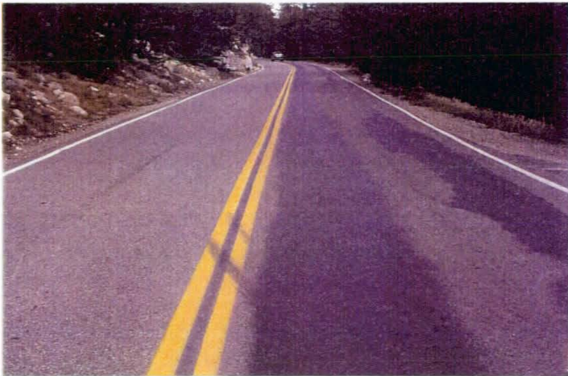
Photo #3473 - MP 40.11 - Typical Pavement Section
