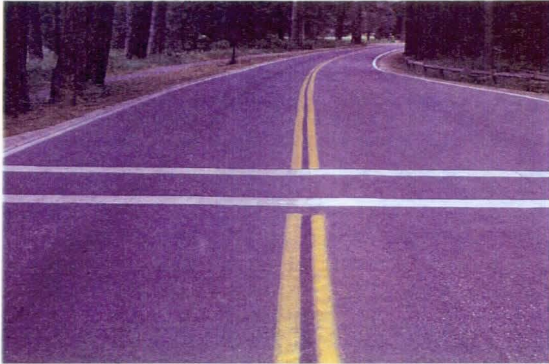
Photo #3478 - MP 0.08 - Typical Pavement Section
