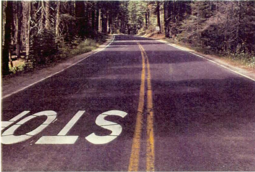
Photo #3470 - MP 0.04 - Typical Pavement Section
