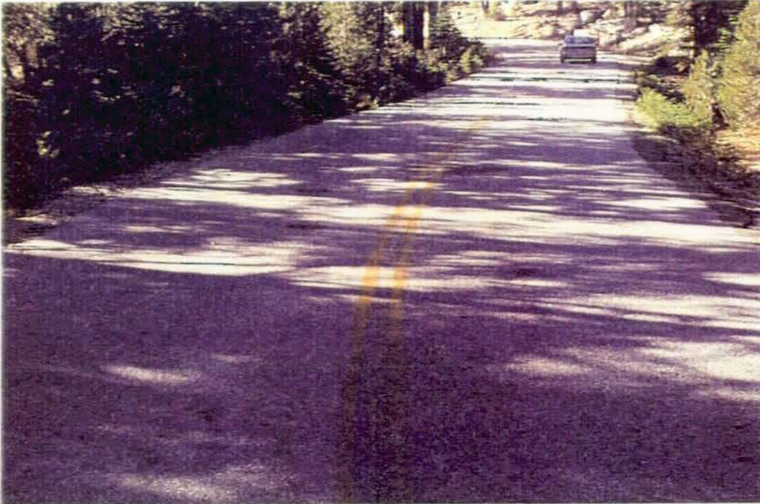
Photo #3476 - MP 0.00 - Begin at Rte 017
