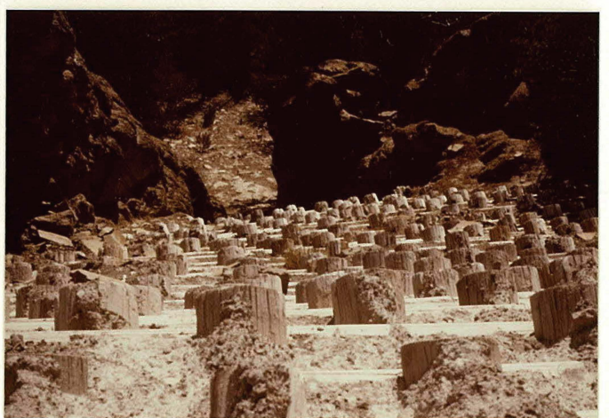
MP 0.86 Exposed Face of Cribwall From Edge of Roadway
