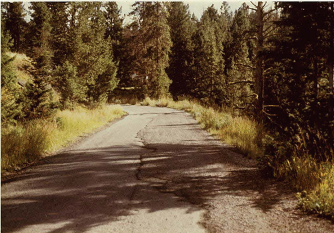
MP 0.29 Patched Roadway
