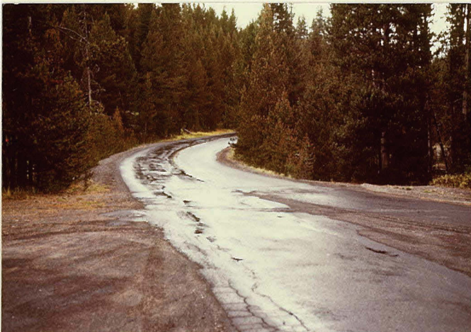
MP 0.15 Typical Road Condition
