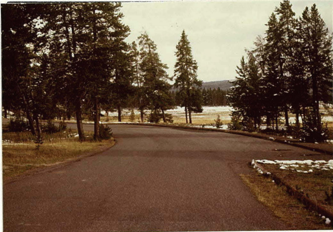
MP 0.28 Entrance Parking Area
