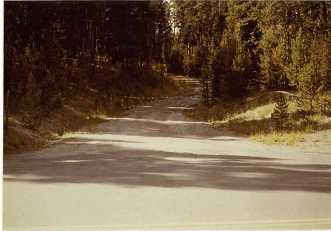
MP 0.00 Gated Approach to Route 10
