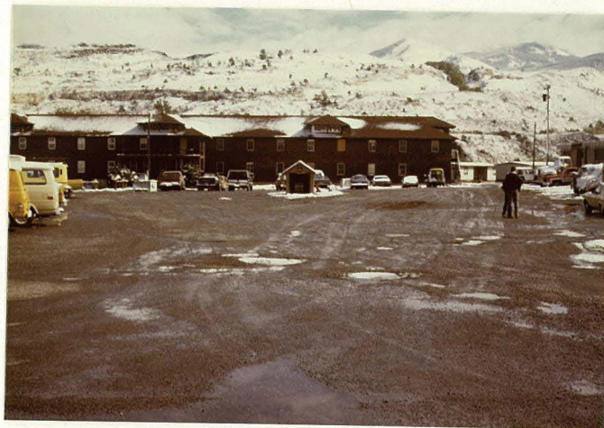
MP 0.25 Unpaved Parking Area
