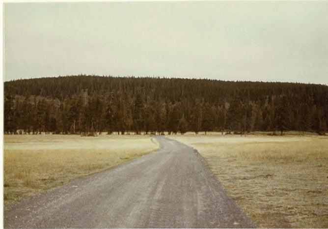
MP 0.23 Typical Roadway Condition
