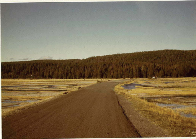
MP 1.24 Typical Road Condition
