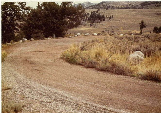
MP 0.33 Parking Area at Road End
