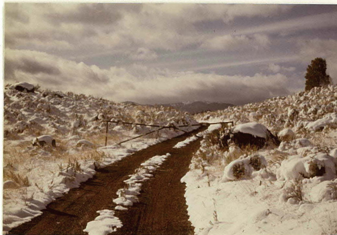
MP 0.15 Gated Service Road
