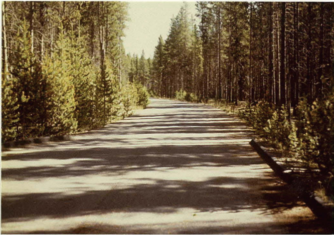
MP 0.24 Typical Road Condition
