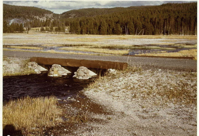
MP 1.29 Low Profile Culvert
