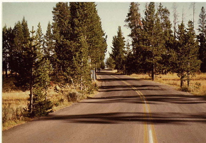
MP 0.66 Entrance Road
