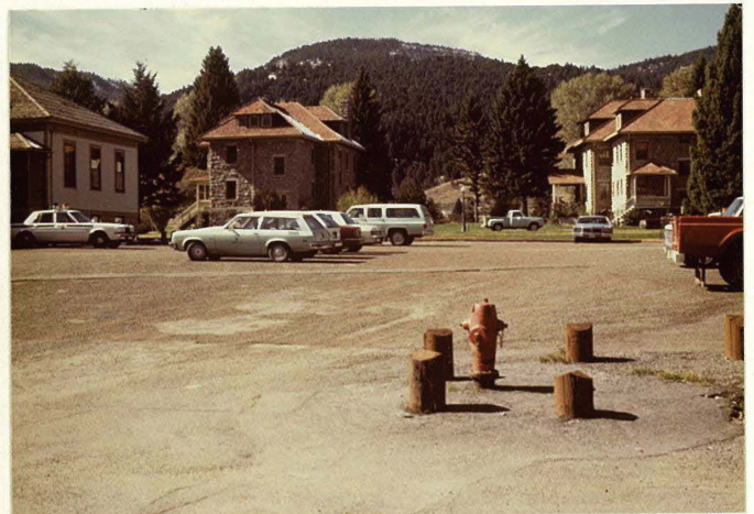
Administrative Parking Area
