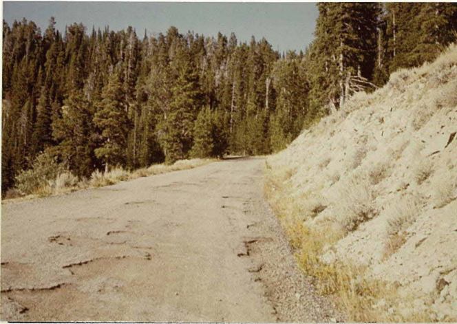
MP 0.46 Potholed Roadway ROUTE 260
