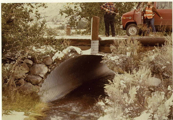
MP 4.47 Reese Creek Culvert
