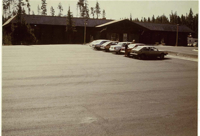
MP 0.99 Hamilton Store Parking Area
