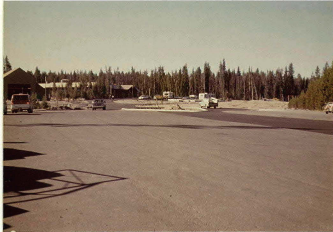
Parking Area at Post Office (Under Construction)
