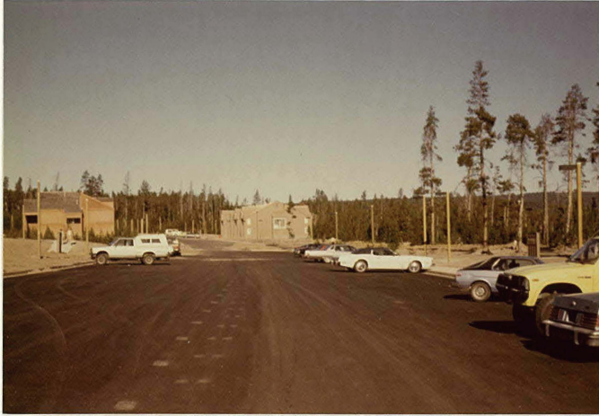
MP 0.38 Lodging Parking Area (Under Construction)
