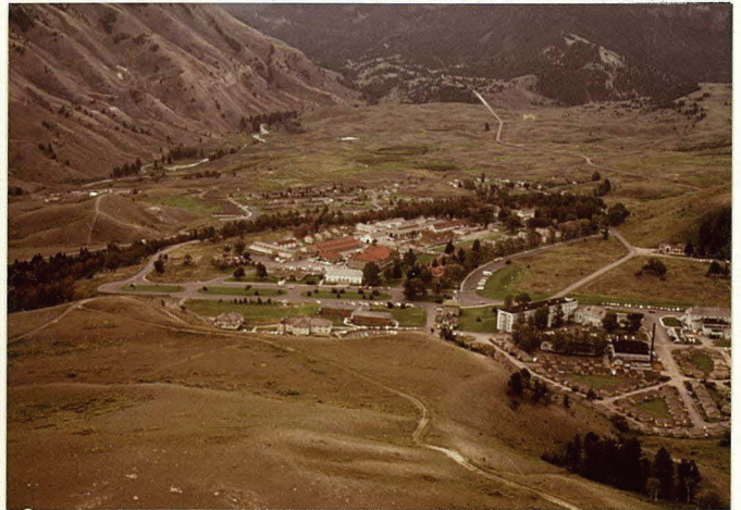
Aerial View Park Headquarters (Upper Center)
