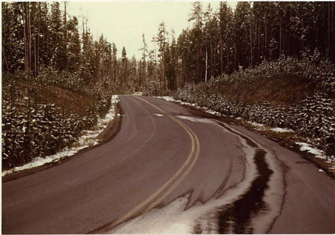
MP 0.06 Entrance Road
