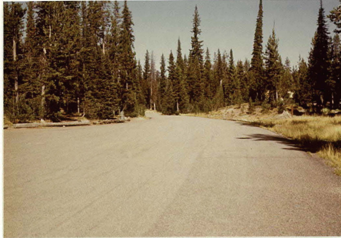
MP 0.21 Lewis Lake Campground Walk-In Parking Area
