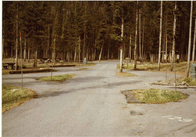
Typical Campground Loop Road
