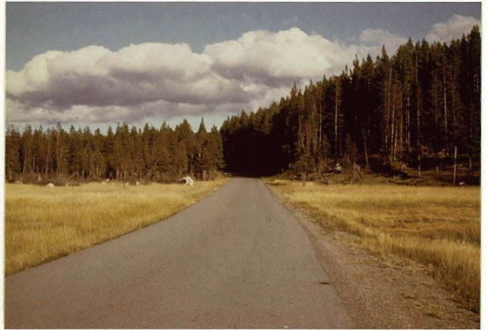
MP 0.13 Typical Road Condition
