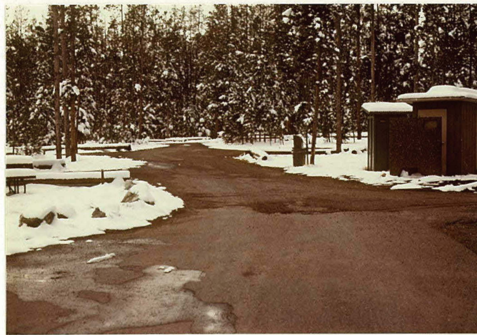
MP 0.58 Typical Campground Loop Road
