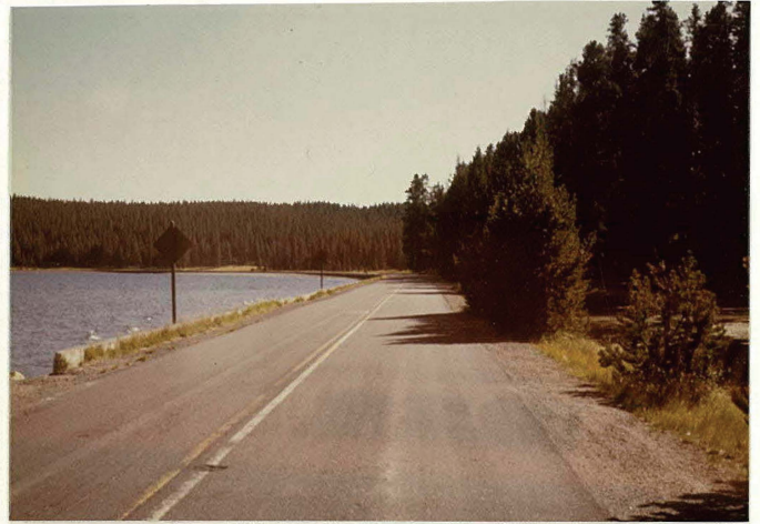
MP 0.15 Retaining Wall Along Yellowstone Lake
