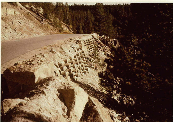
MP 0.84 Timber Cribwalls
