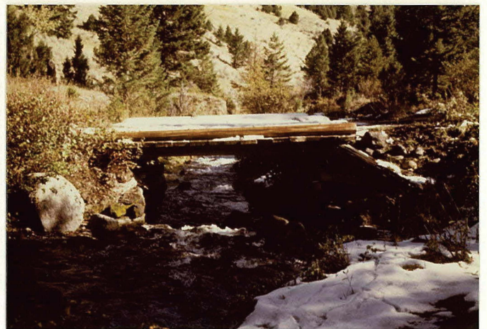
MP 5.23 Glen Creek Bridge
