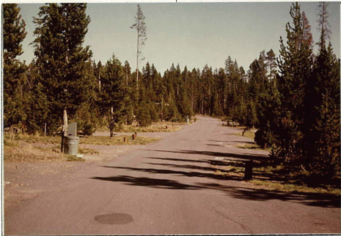
MP 0.86 Typical Road, Bridge Bay Campground
