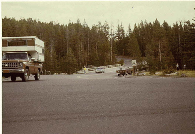
MP 0.00 South Rim Drive and Chittenden Memorial Bridge
