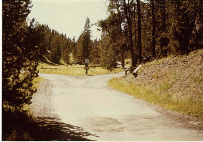
MP 0.88 Loop at Road End, Natural Bridge Vicinity
