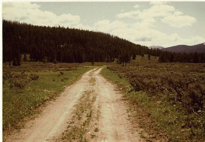
MP 0.15 Eastbound, Typical Primitive Road Condition
