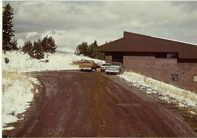
MP 0.81 Mammoth Water Treatment Plant Parking Area
