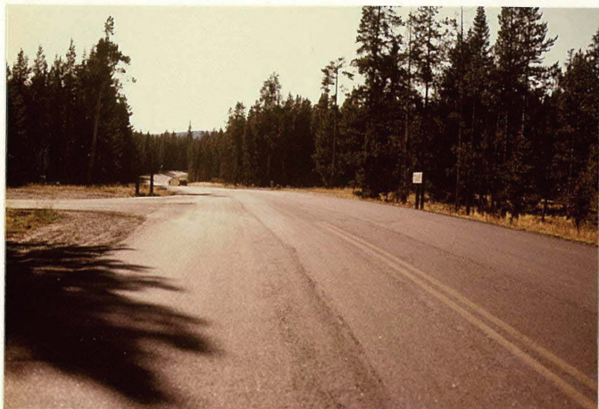
MP 0.35 Entrance Road
