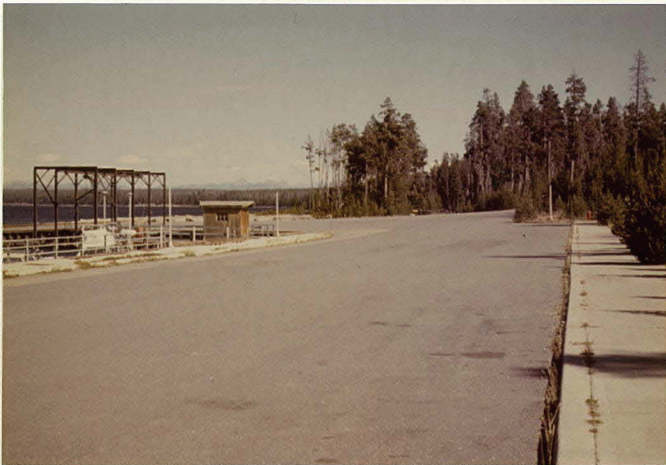
MP 1.12 Grant Marina Parking Area
