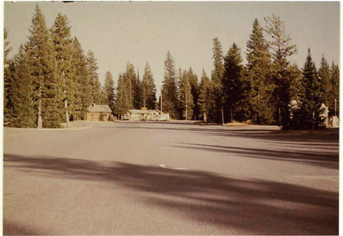
MP 0.25 Parking Area (Facing East)
