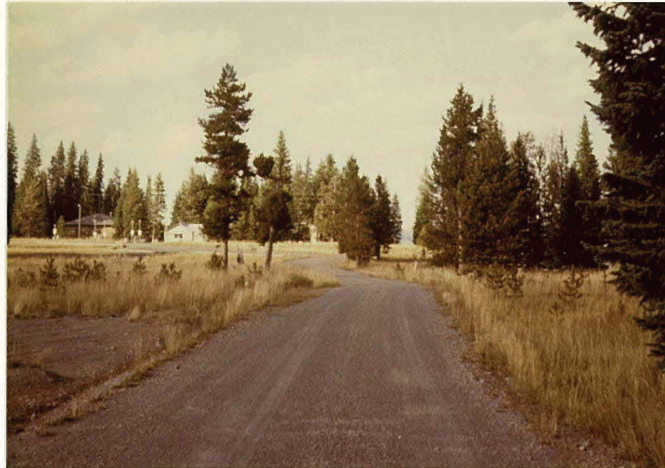
Typical Roadway Condition, West Thumb Service Road
