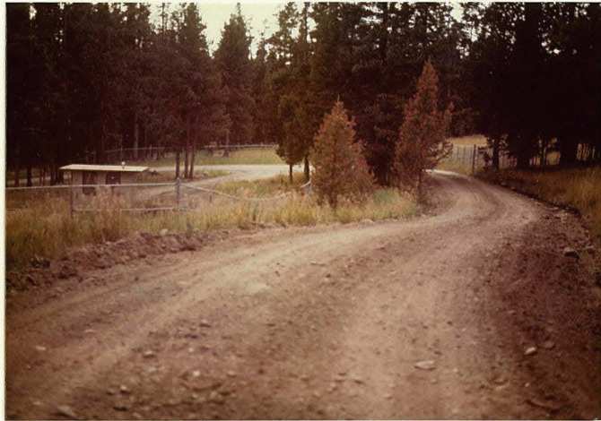
Approach to Sewage Treatment Plant
