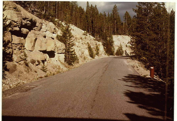
MP 0.63 Typical Roadway, Cascade Gorge Area
