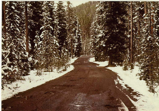
MP 0.18 Typical Road Condition
