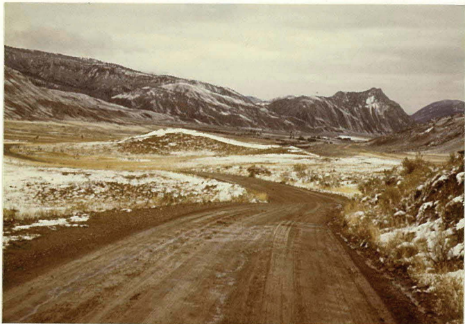
MP 1.52 Typical Condition Reese Creek Road Facing West
