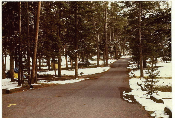
MP 0.32 Typical Road Condition
