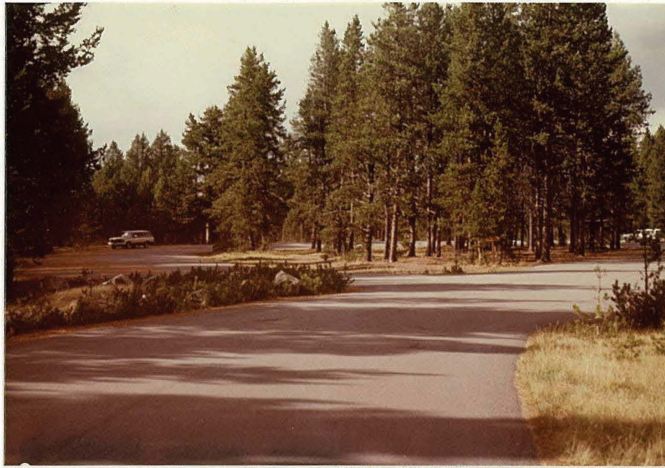
MP 0.28 Typical Road Condition
