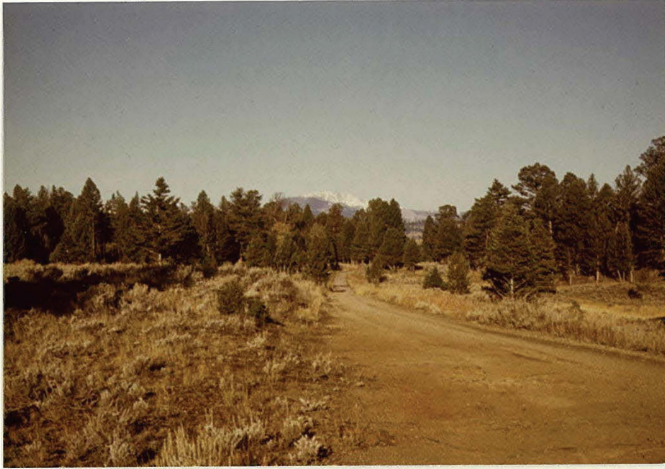
MP 0.51 Typical Unsurfaced Roadway
