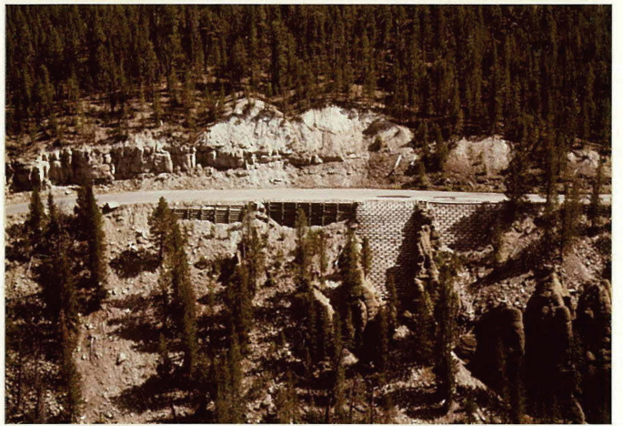
Aerial View, MP 0.80 to MP 0.90 Vicinity, Timber Cribwalls
