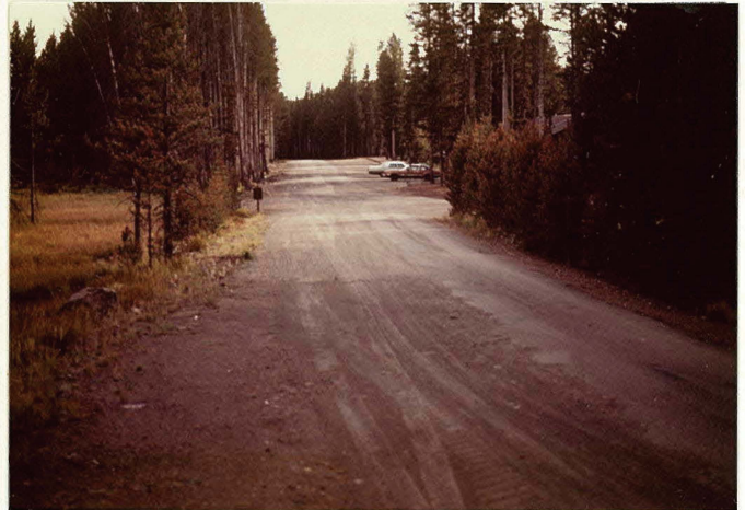
MP 0.92 Facing South, Canyon Residence Area
