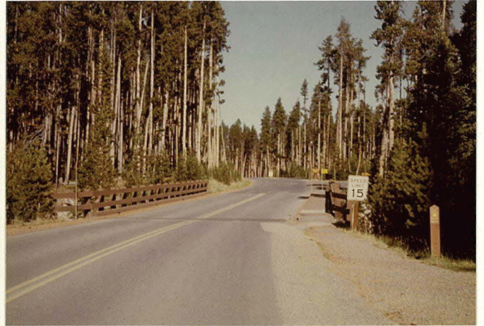
MP 1.39 Bridge and Campground Entrance
