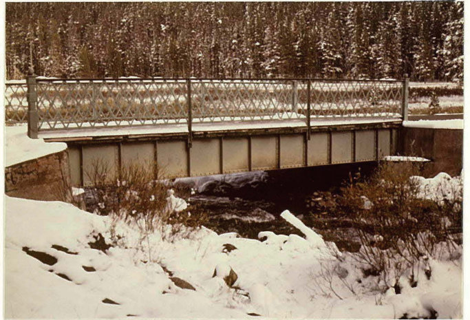
MP 0.11 Obsidian Creek Bridge
