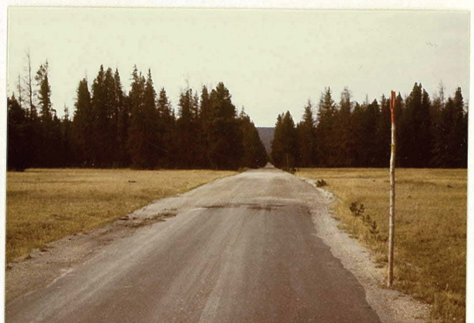
MP 1.82 Facing South, End of Pavement
