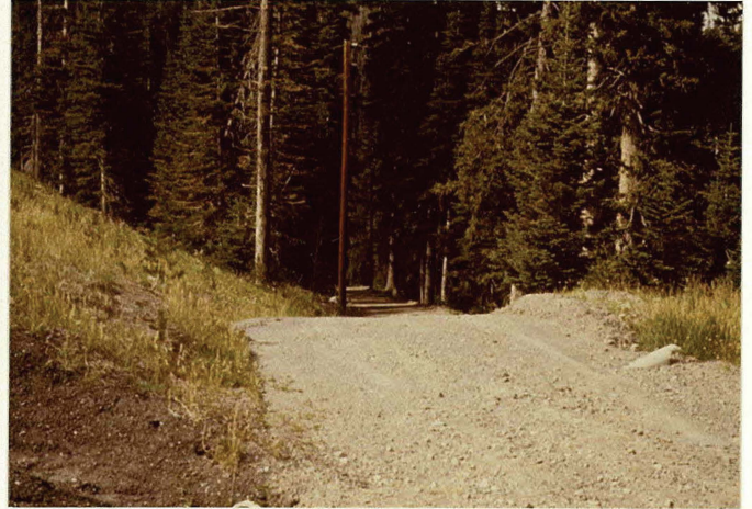
MP 0.02 Road Entrance
