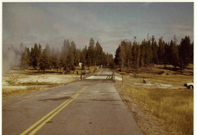
MP 1.23 Facing North New Firehole River Bridge
