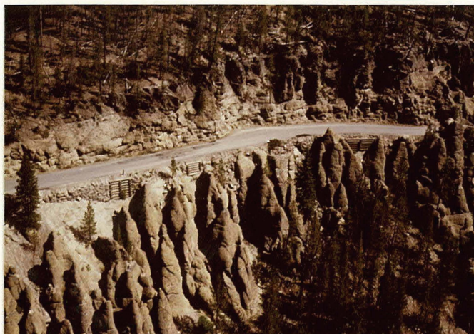
Aerial View, MP 0.93 to MP 1.00 Vicinity of Rubble Walls and Cribwalls
