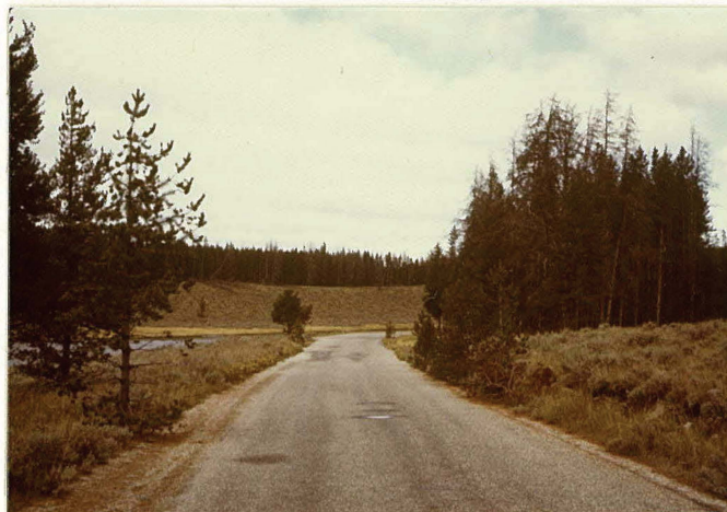
MP 0.13 Typical Road Condition
