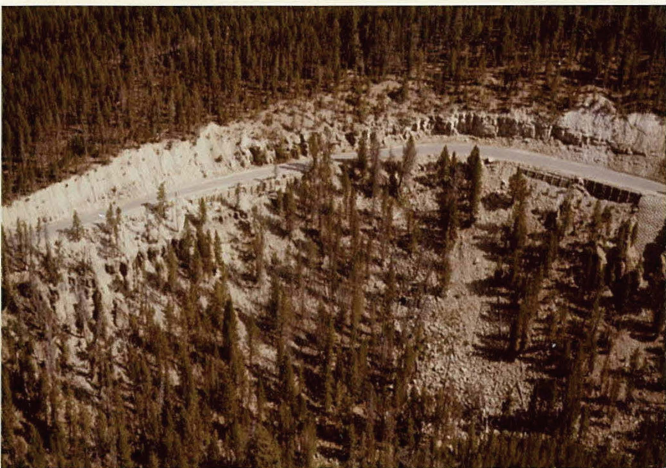
MP 0.70 to MP 0.85 Vicinity, View of Roadway and Cribwalls
