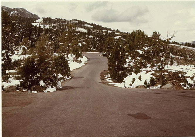
MP 0.24 Typical Road Condition
