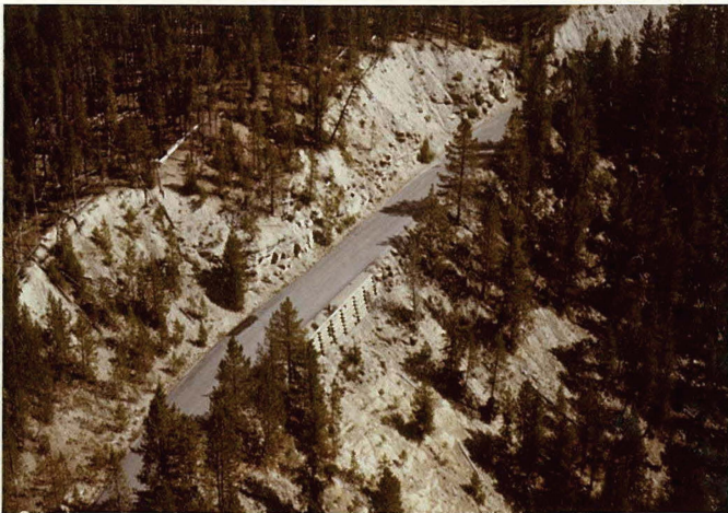
MP 0.60 Vicinity, Timber Cribwall
