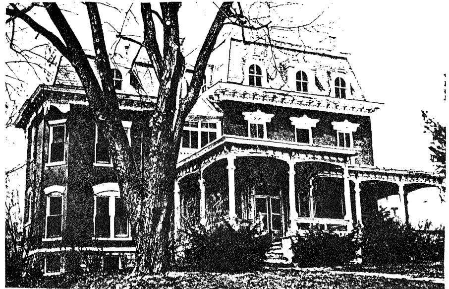
The Armitage, demolished to make room for former Seneca Falls Hospital. Photo courtesy of Seneca Falls Historical Society, Lost & Found: Nineteenth Century Architecture in Seneca Falls, 1981, p. 2. Demolished in 1975. This building was part of what was once called "Terrace Row."
