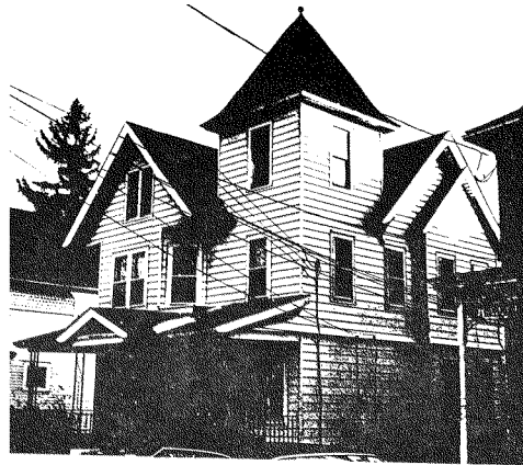
1981 Photo by Cornell Univ. before removal of aluminum siding.
