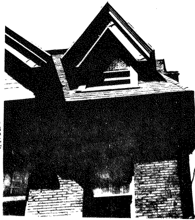
Detail of dormer over main entry
