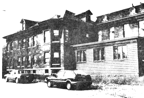
View of side (south) façade
