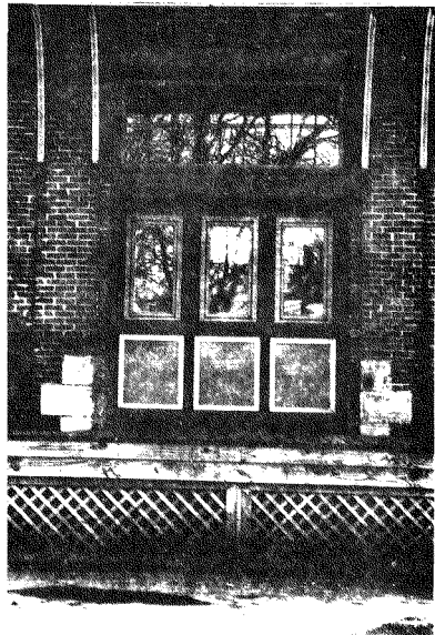
Detail of Loading Door
