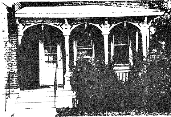
Front Porch Detail in the ell
