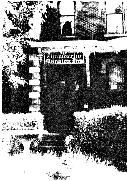
Detail of Main (West) Entry
