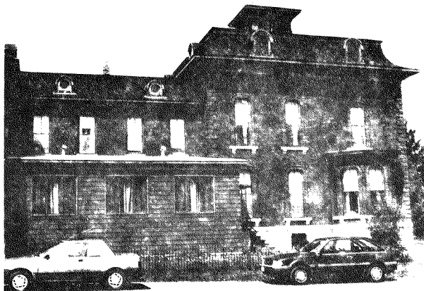
View of side (south) façade
