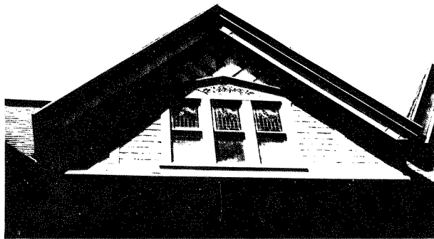
Detail of dormer on main (east) façade
