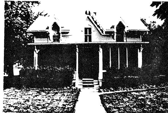
Front View of 62 Cayuga Street
