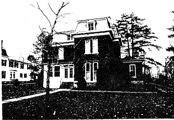
December 1980 Photo by Cornell Univ. Preservation Planning Shows porch before remodelling
