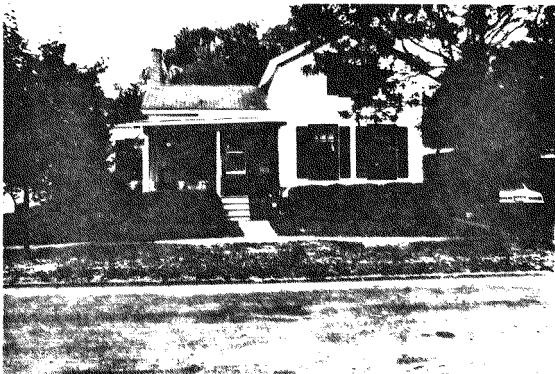
View from Johnston Street of Main (South) Façade
