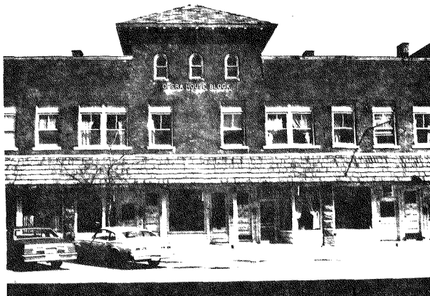
View of West Façade
