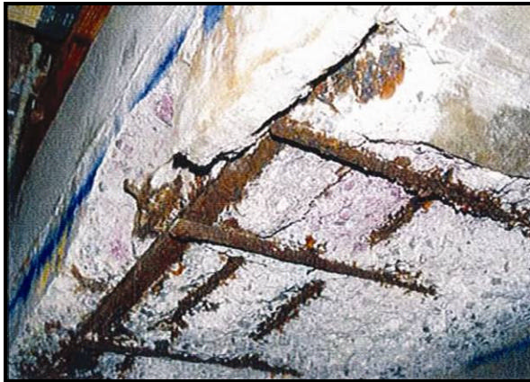
FIGURE 2. STRUCTURAL DETERIORATION AT USS ARIZONA MEMORIAL VISITOR CENTER
