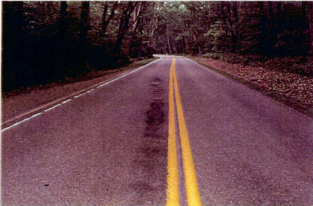
Photo #2967 - MP 58.92 - Localized pavement distress
