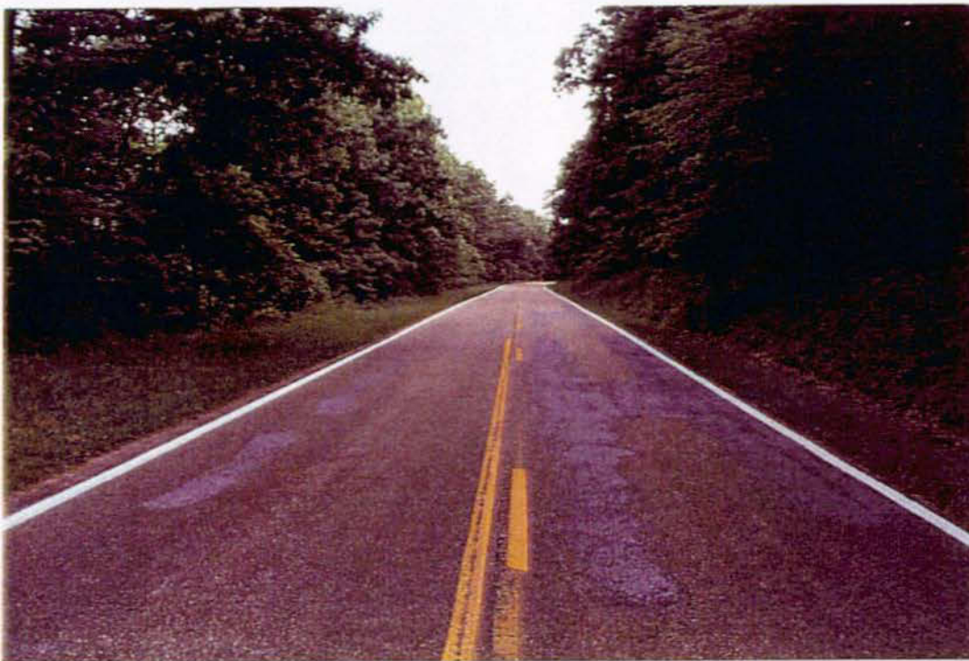
Photo #2971 - MP 101.00 - Pavement Patching Distress
