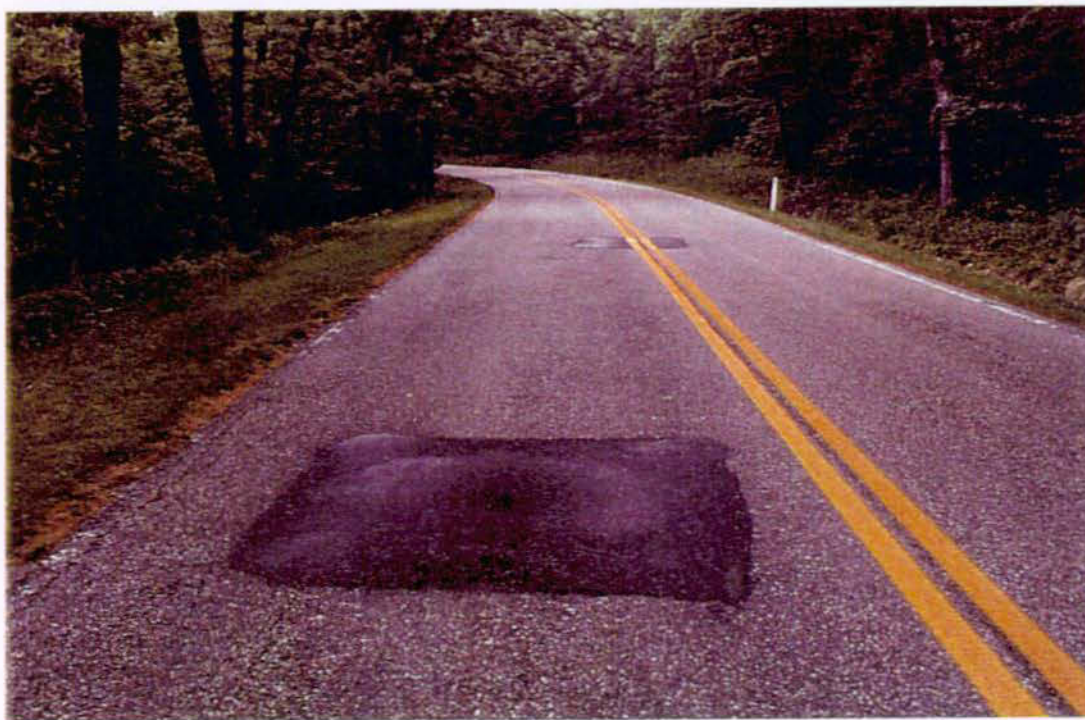
Photo #2963 - MP 42.08 - Pavement Patch
