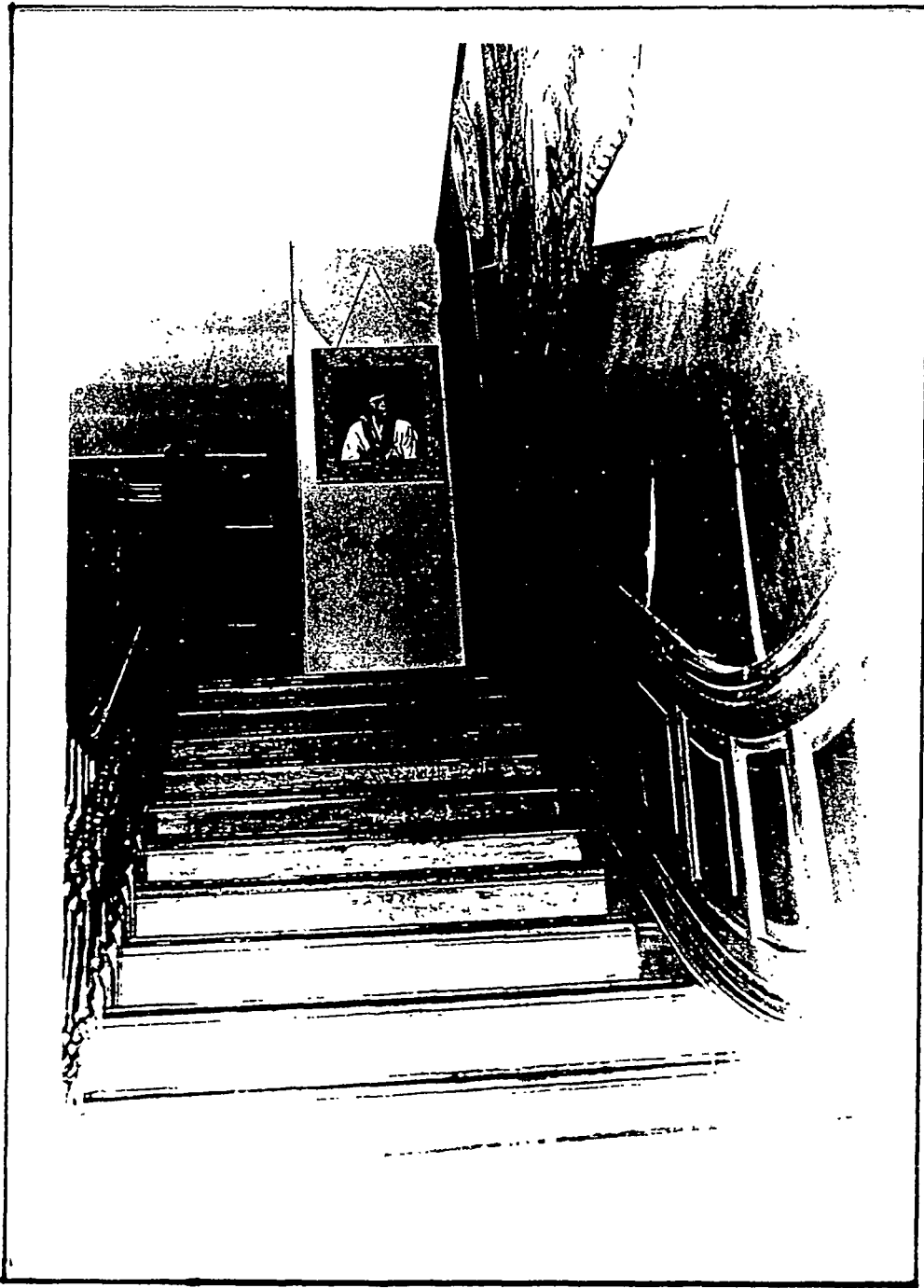
Fig. 1. Main staircase; Front Hall (Room 101) looking east, 1948. Photographic collection, SAHI NHS. After 1948, the rectangular wall at the top of the stairs was changed to an arch.
