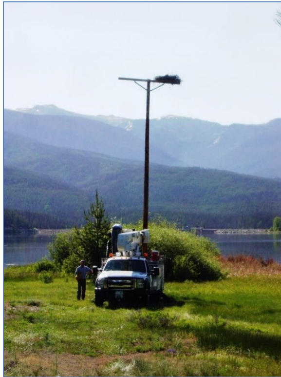
Figure 2. Bucket truck at Shadow Mountain Reservoir osprey Nest near Rocky Mountain NP.
