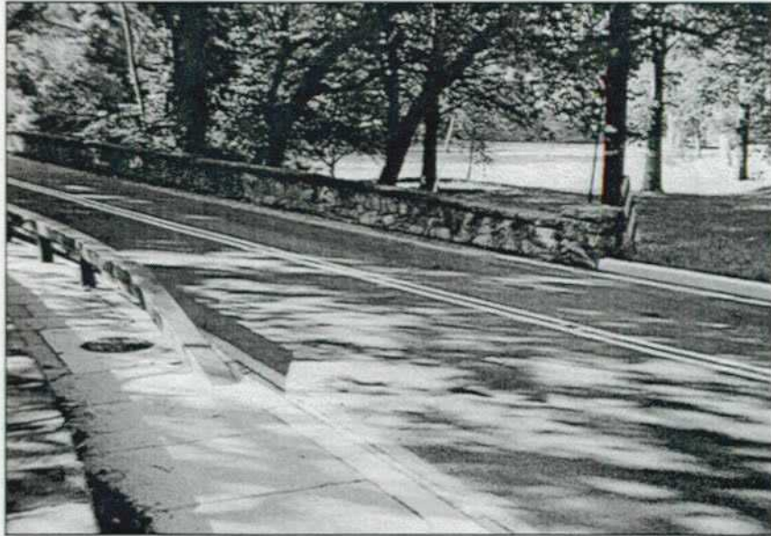
This photo of the west end of the bridge on Tilden Street shows two bridge end treatments used in the Park. The stone guidewall on the far side of the street is vertical and appropriately accompanied by a black and yellow object marker. The steel guardrail on the near side of this street is rolled down. Tilden Street and this bridge are under the jurisdiction of the DC DPW.
