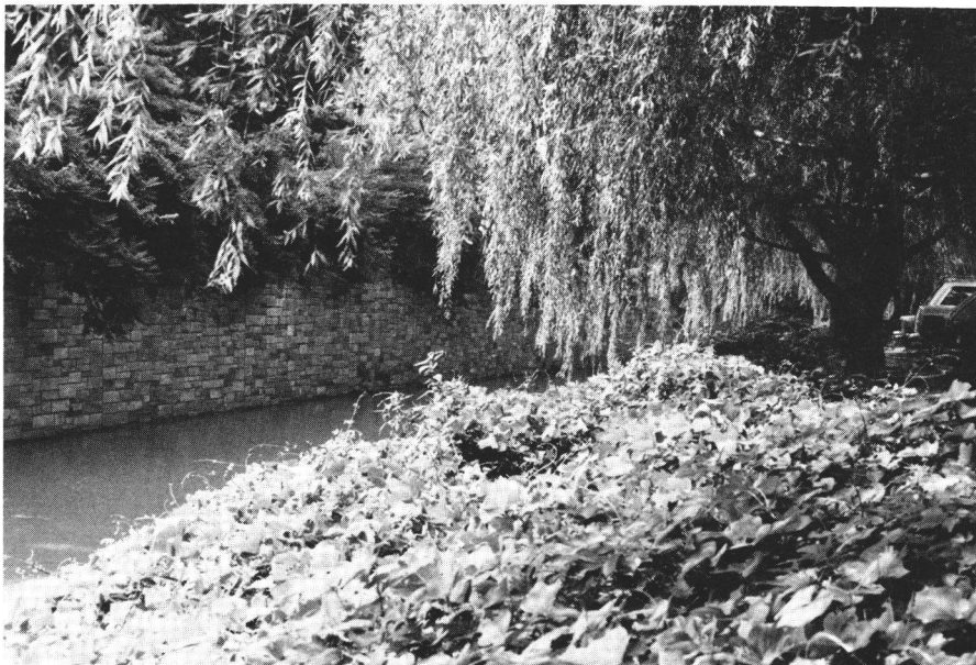
Figure 6-6 Retaining Wall Along Rock Creek at the National Zoo
