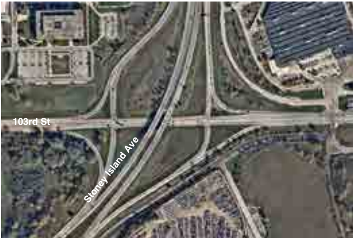
Cyclists crossing the 103rd Street interchange east-west, even on a sidepath, would be required to cross 4 potential points of conflict in each direction as they pass vehicle on/off ramps.
