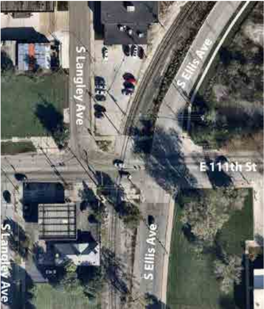
Complex intersection at Langley Ave, Ellis Ave, and 111th Street.
