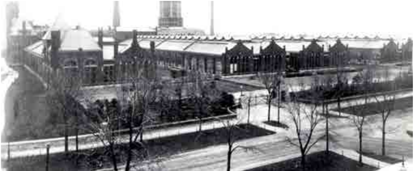
Photo showing historic midblock crossing at St. Lawrence
