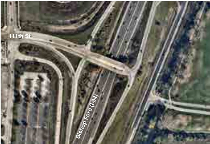
111th Street overpass poses the fewest potential conflicts for cyclists in its current form, and presents the widest contiguous bridge section to install a protected bike facility.
