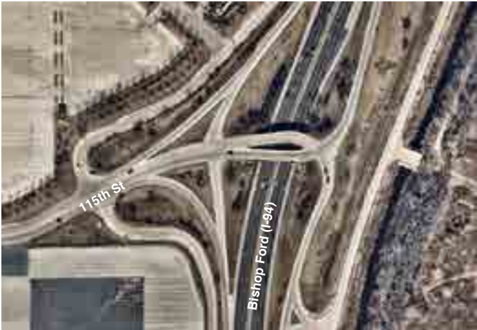
Although similar to 111th Street, the central opening in the 115th Street overpass limits the negotiable width for a protected bike facility in both directions.
