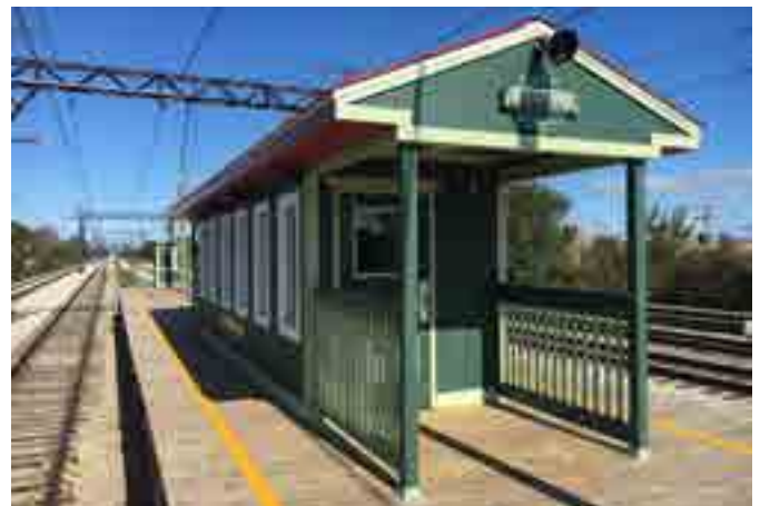
Metra 111th Street station
