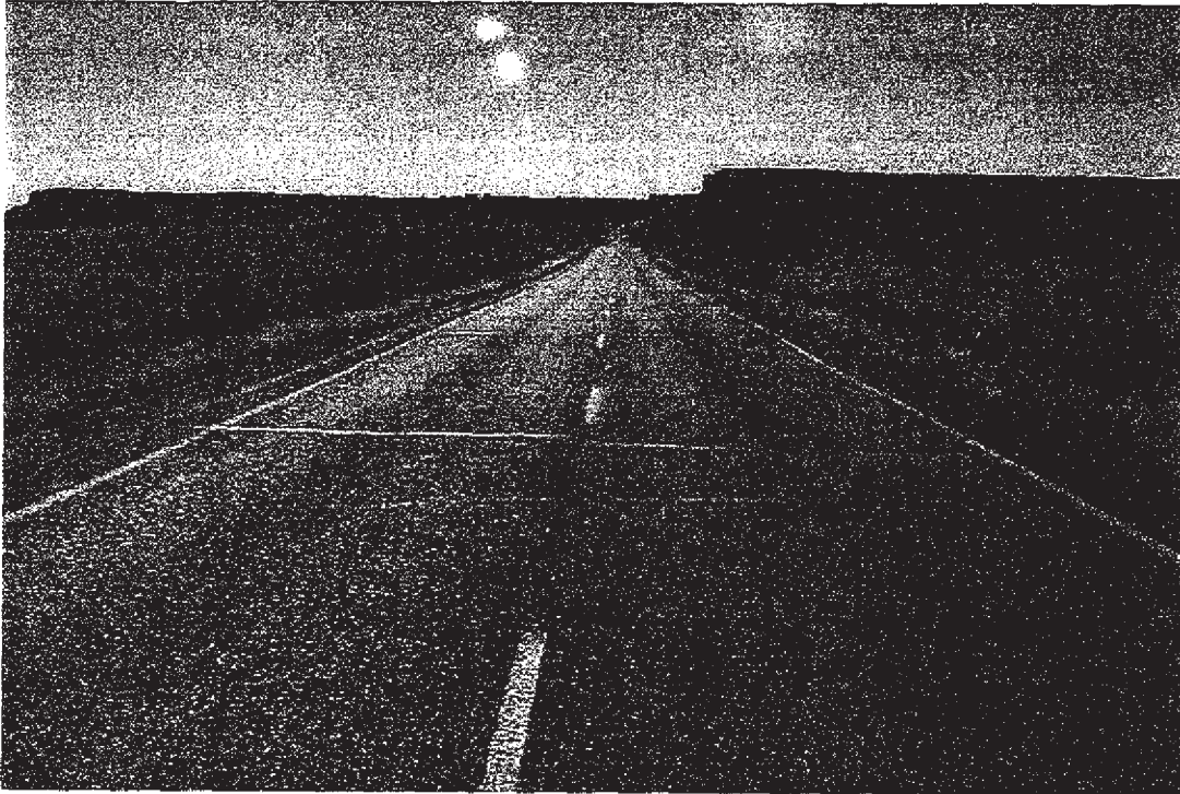
Photo #1828 - MP 17.10 - Typical Pavement Section, Note Transverse Cracking
