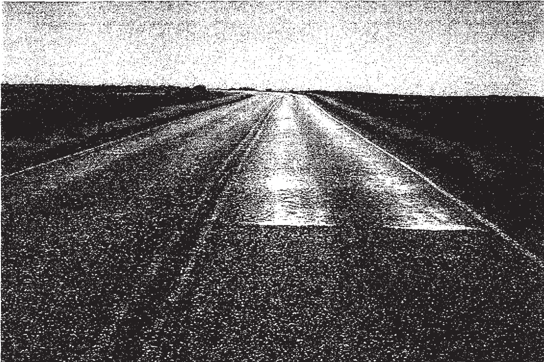
Photo #1824 MP 11.40 Typical Pavement Section, Note Raveling and Bleeding
