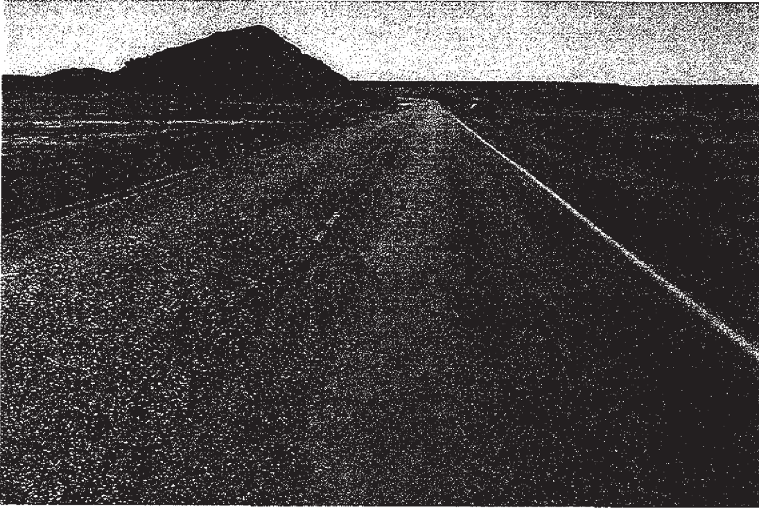
Photo #1826 MP 14.10 Typical Pavement Section, Note Bleeding
