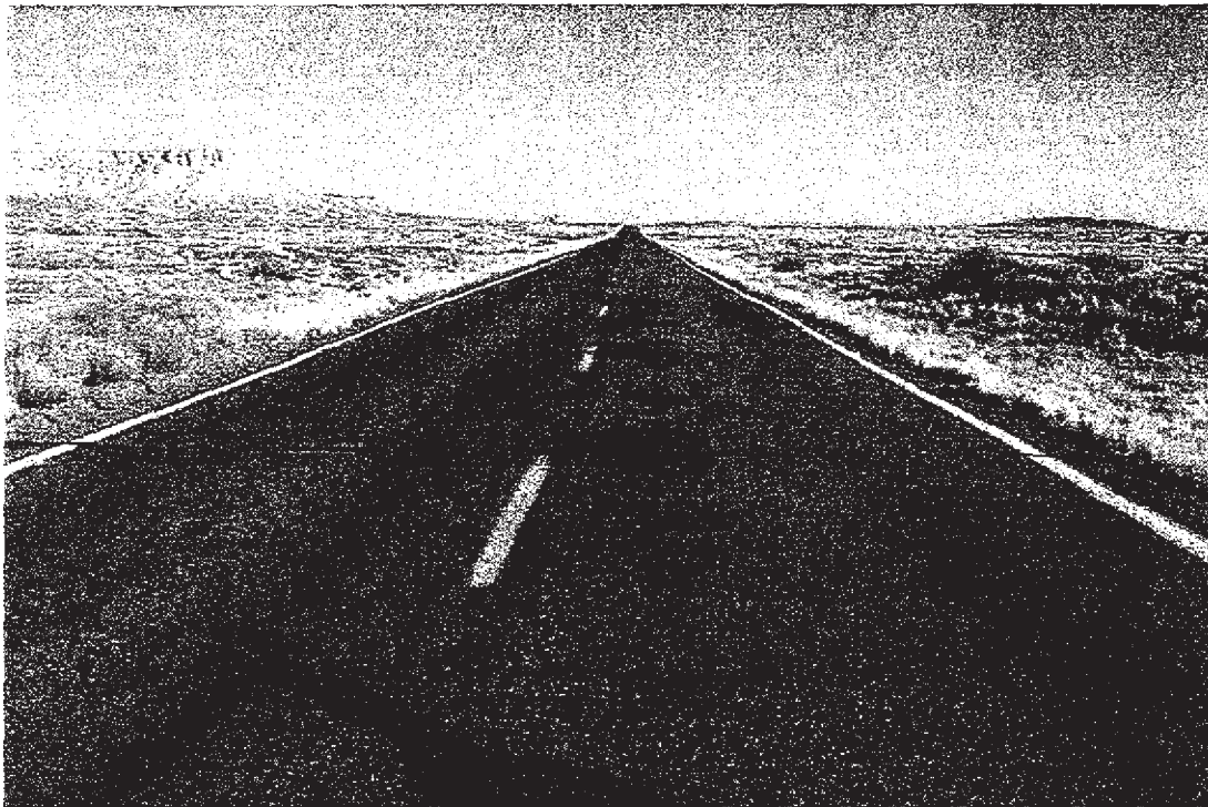
Photo #1844 - MP 0.40 - Typical Pavement Section, Note Full width Transverse Cracks
