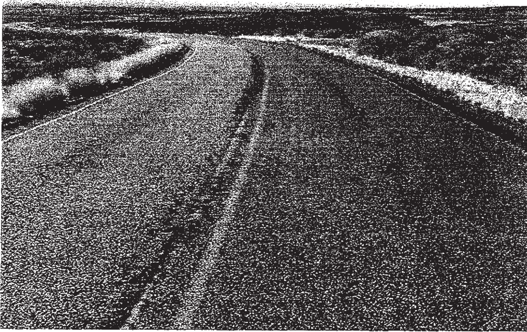
Photo #1822 - MP 4.18 - Typical Pavement Section, Note Raveling of Chipseal
