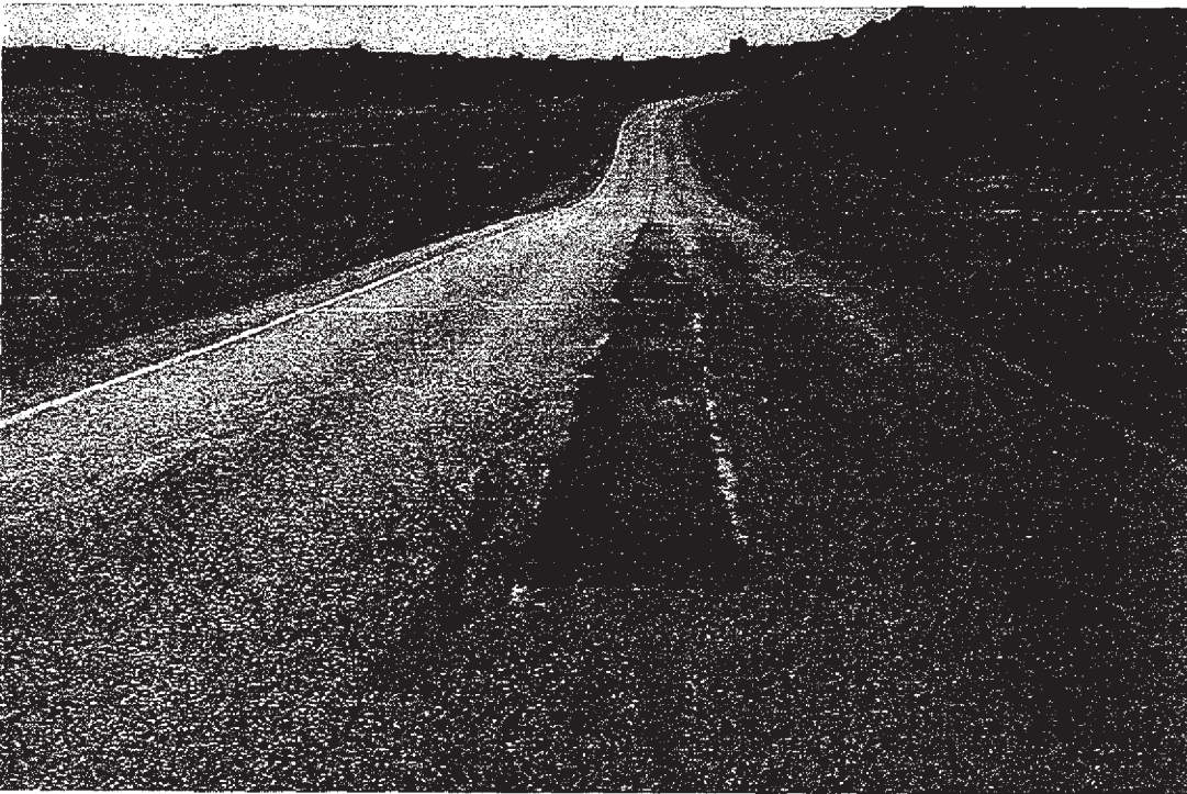
Photo #1829 - MP 17.42 - Typical Pavement Section, Note Patching
