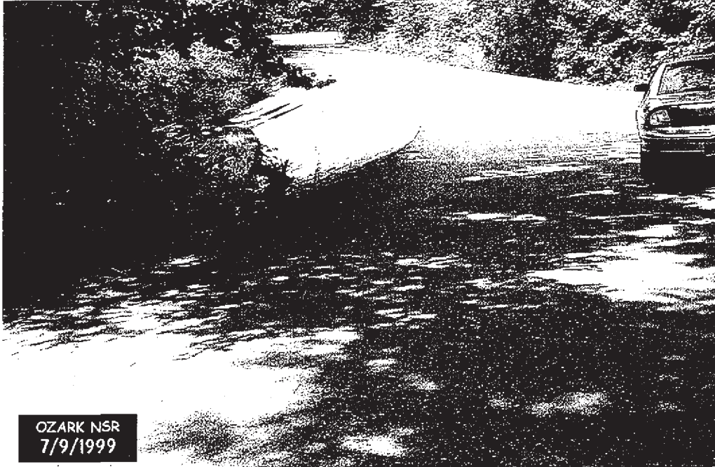
Photo # 09 - Route 112, Longitudinal and Transverse Cracking.
