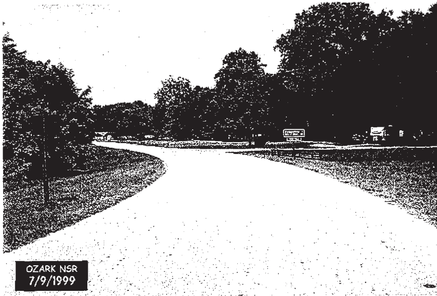
Photo # 21 – Route 227, Typical Pavement Section.
