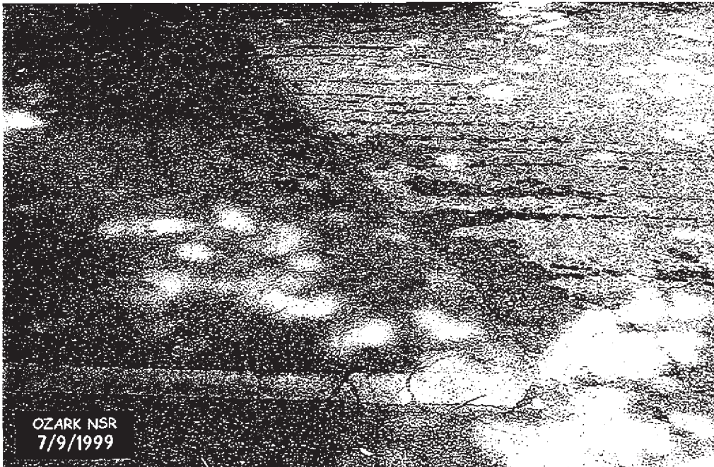
Photo # 10 - Route 112, Detail of Improved Wash and Alligator Cracking.
