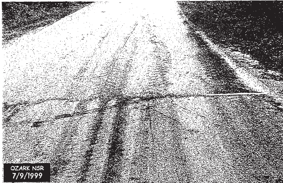
Photo # 02 – Route 015, Section Change and Pavement Change.
