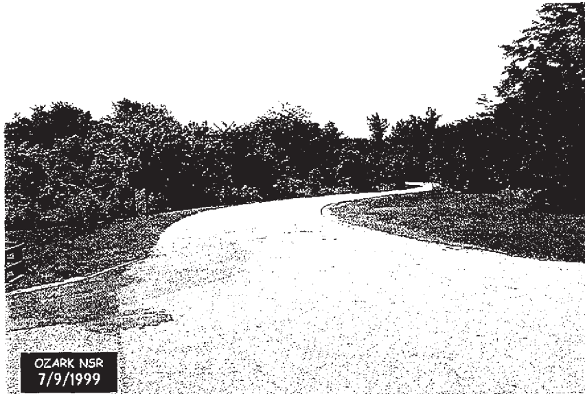
Photo # 22 – Route 227, Pavement at Intersection with Route 228.
