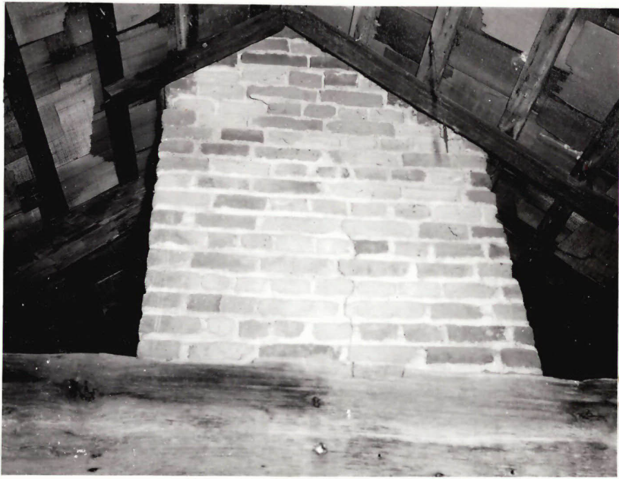
2. Chimney in attic, showing crack in brickwork.
