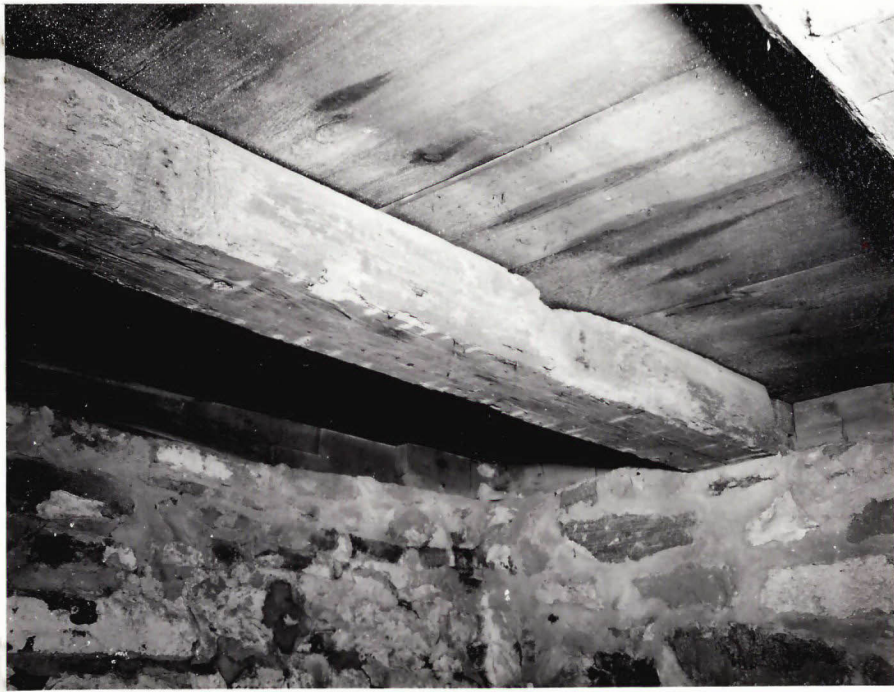
4. Condition of floor joists in cellar.
