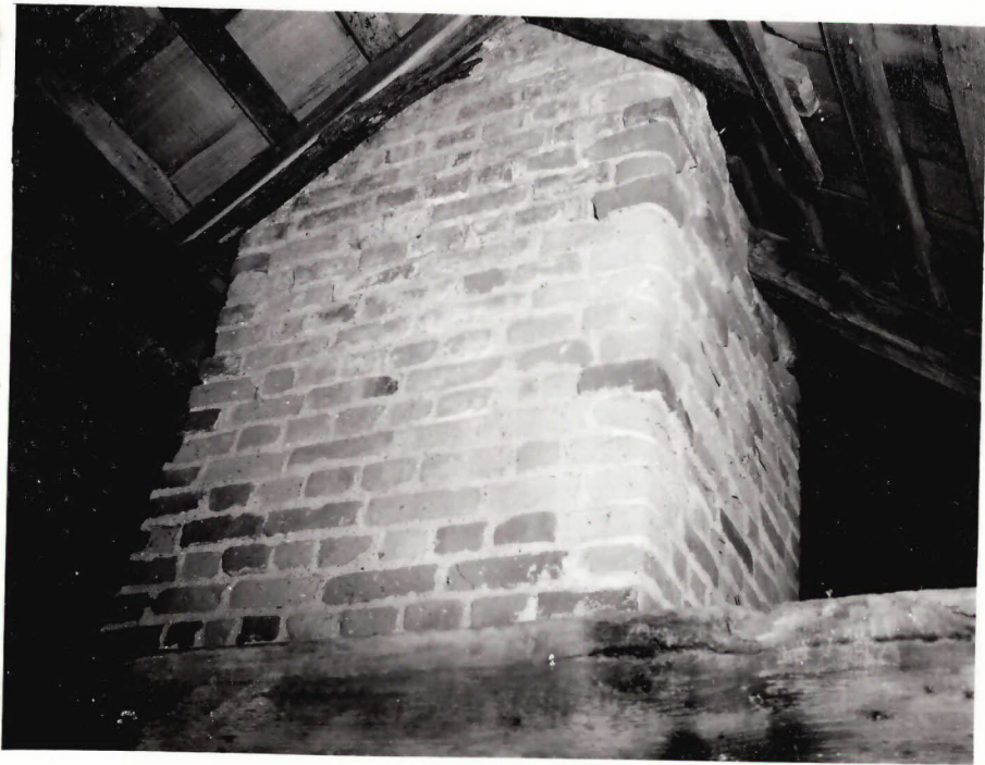
3. Chimney in attic, showing missing brick.
