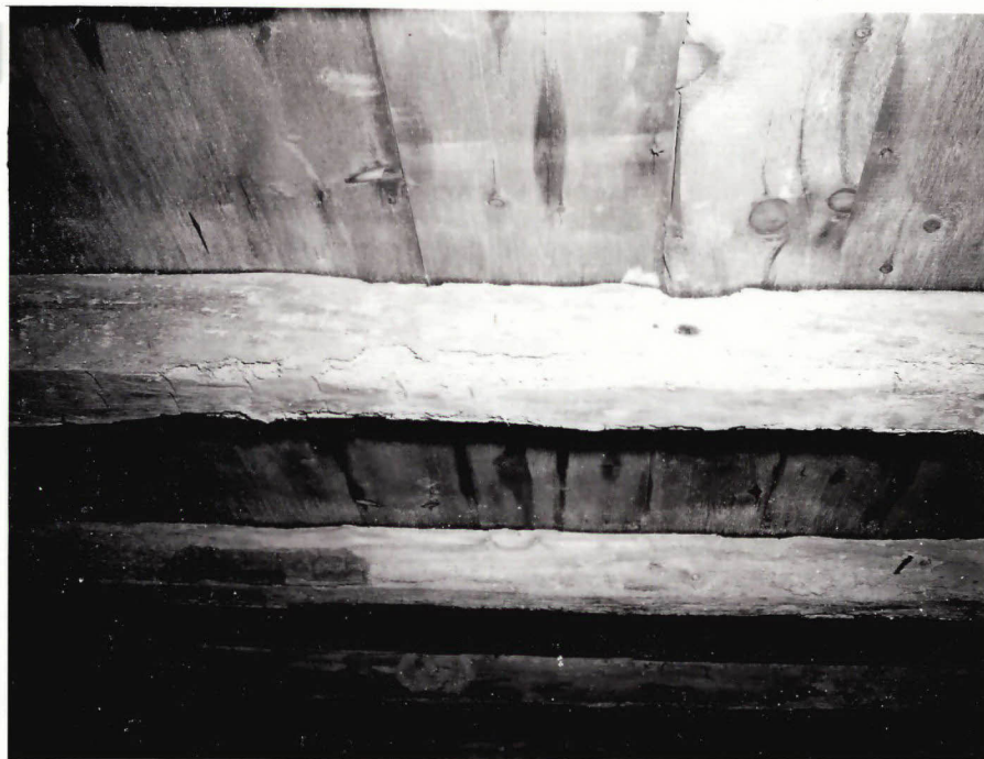
5. Another view of floor joists.
