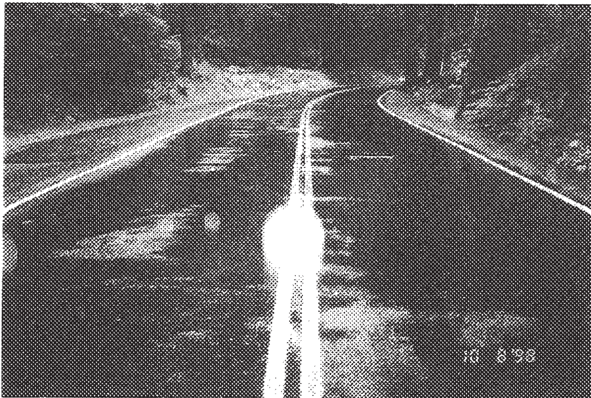
Photo R1-04 - MP 4.00 - New overlay
