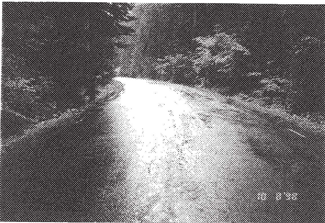
Photo R2-15: - MP 5.90 - Typical blade patch
