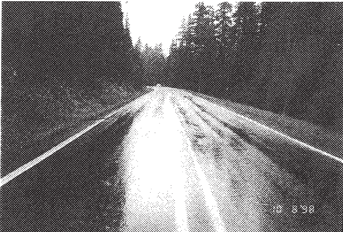
Photo R2-18 - MP 11.10 Typical pavement section, looking back
