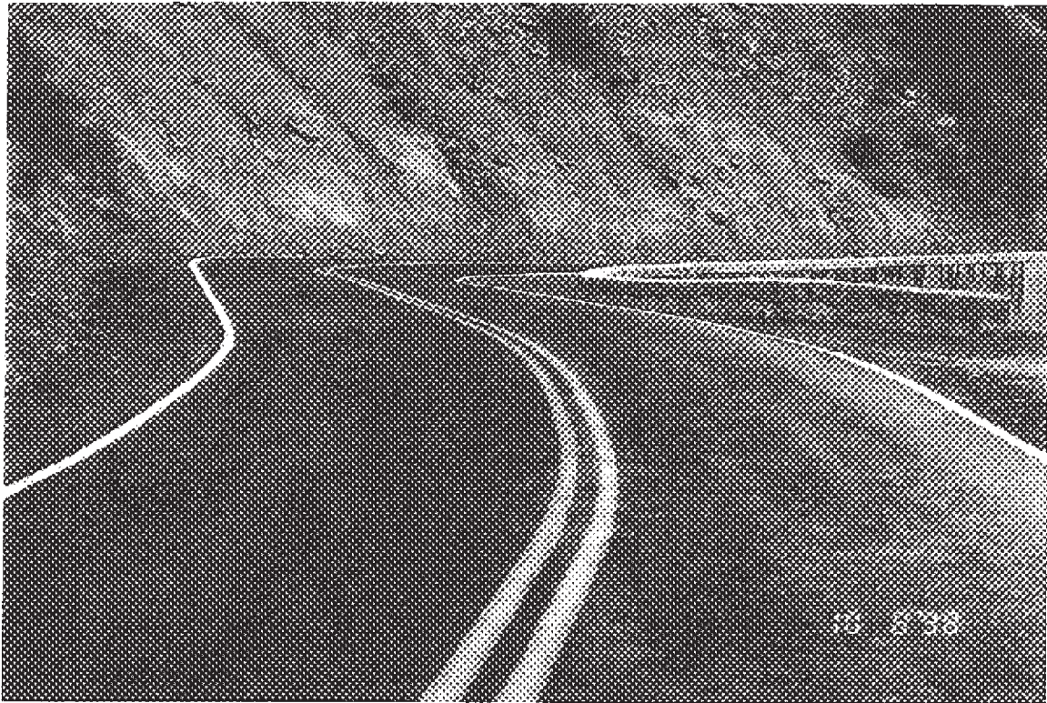
Photo R3-14 - MP 7.30 - Start new pavement
