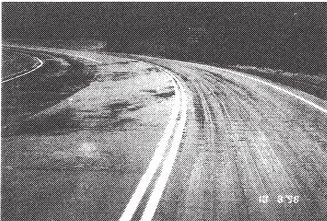
Photo R1-10 - MP 15.50 - Mill section
