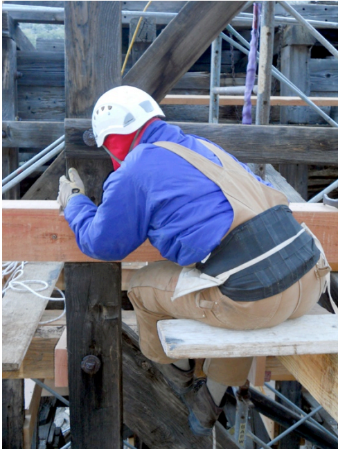
Figure 53: The upper posts were moved into position on top of the replacement sill, correcting the buckle in the bent.
