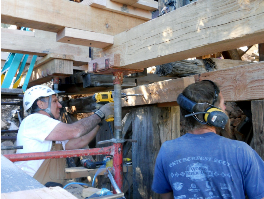
Figure 32: The eastern half of the subframe's cap beam was damaged and replaced in kind. The members strengthening the joint between the two cap beam halves were also replaced in kind (both sides of the beam). Here, holes are drilled into the replacement members so hardware can be reinstalled.
