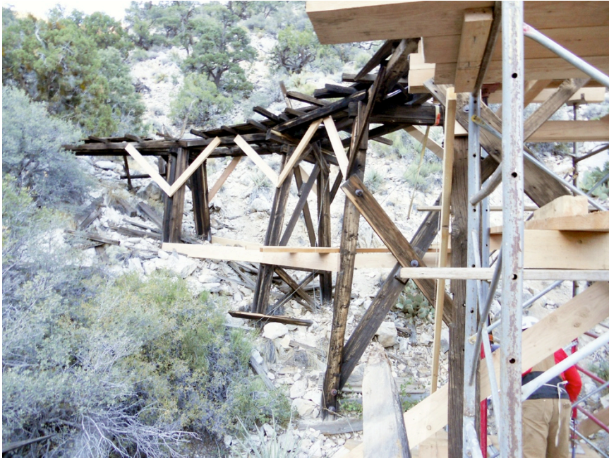
Figure 17: Much of the diagonal and longitudinal bracing between the trestle bents was damaged or missing. Braces were replaced in kind when they could not be salvaged or reattached securely.
