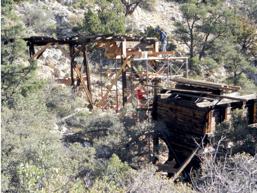
Figure 28: Structural staging and cribbing was also installed between the ore bin and bent 1 and bents 1 and 2.
