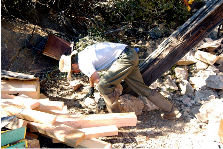
Figure 36: the bottoms of the braces had decayed from prolonged contact with the ground. Decayed portions were removed and the ends were reset in stone.
