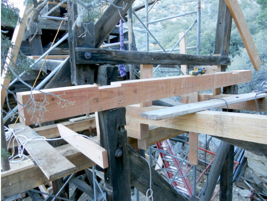
Figure 52: A new sill was cut using the old timber as a template and set on top of the lower posts.
