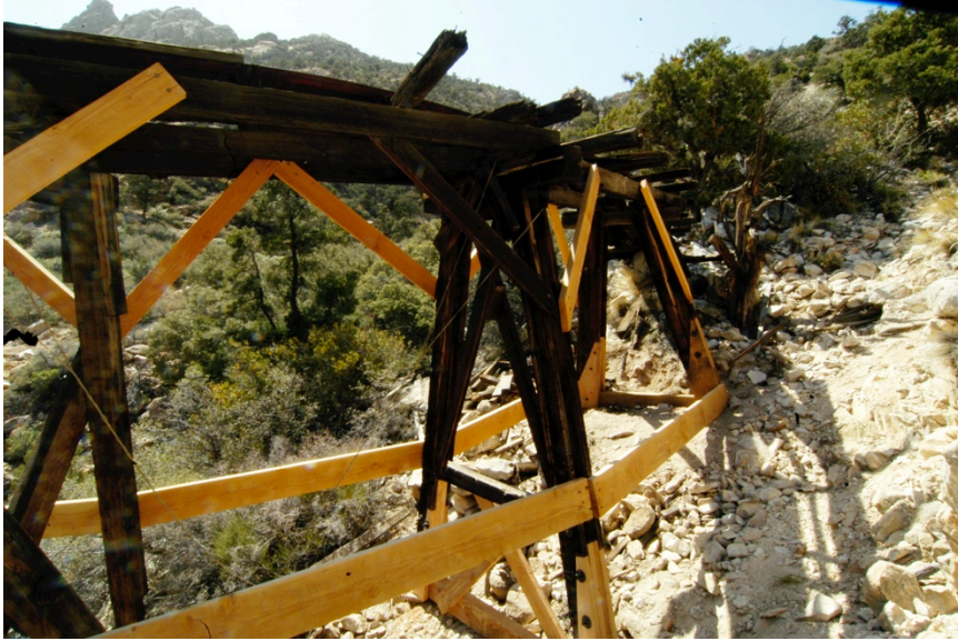
Figure 62: New wood was scarfed into the columns of bents 3 and 4 and their sills were replaced in kind. Spacers were placed between the repairs in the dimensional lumber posts and through-bolted. See Appendix B, sheet XXX for details of the repairs.
