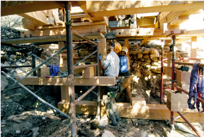
Figure 43: The two westernmost posts in the subframe were badly decayed and had lost significant portions of their length. The posts were replaced in kind after installation of the new sill. Here, the second post from the west is moved into position.
