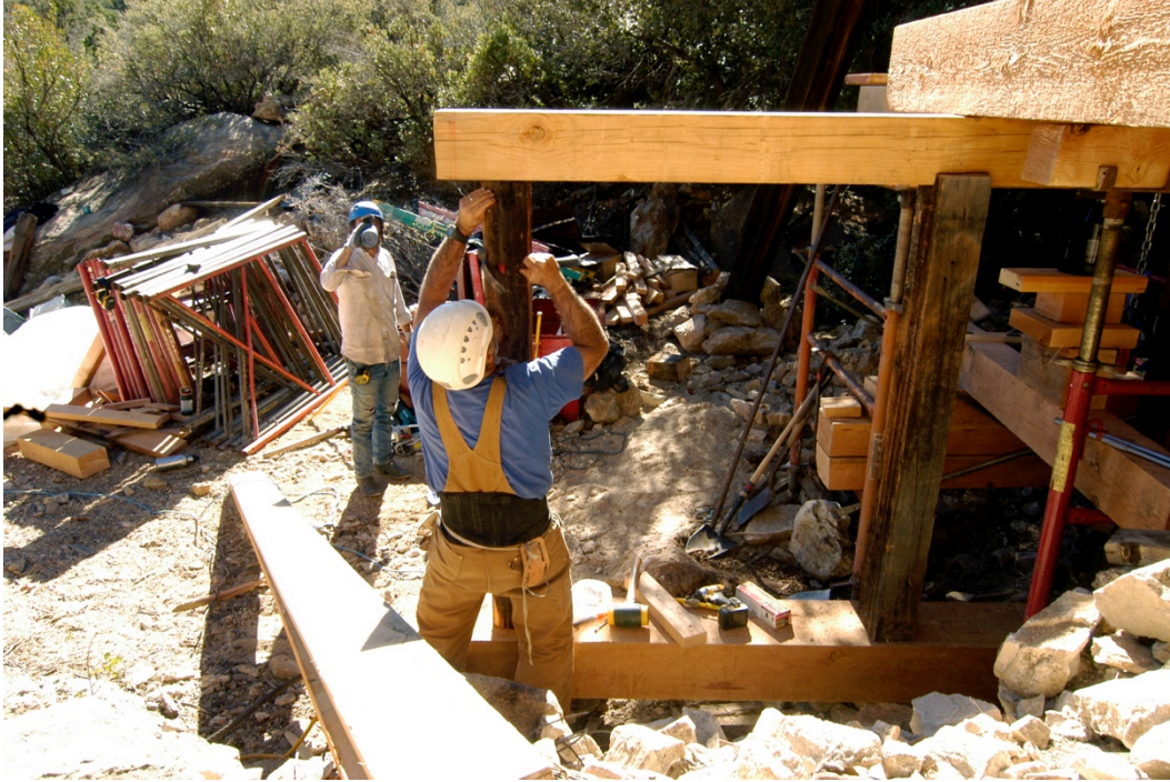
Figure 44: The three eastern posts in the subframe did not require repair and were reinstalled.
