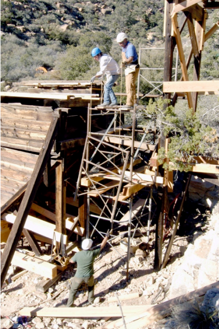
Figure 56: Taking down structural staging at the completion of work on bent 1 during the first repair visit.
