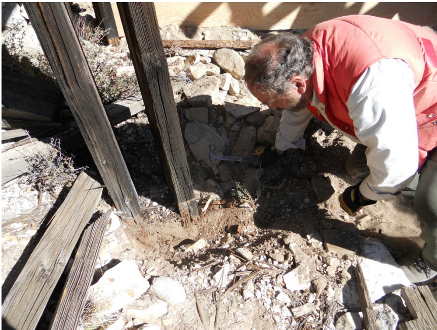
Figure 61: The sills at bents 3 and 4 had been largely lost to decay due to prolonged debris build-up
