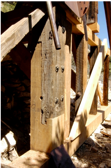
Figure 45: The center post was decayed at its bottom. The decayed material was removed and new wood was scarfed into the bottom of the post. A smaller post, just visible to the right of the scarfed repair, was installed to help support the end of the east half of the cap beam. This work was completed during the second repair visit.
