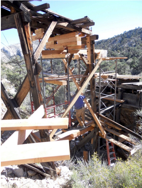
Figure 29: A view of the cribbing supporting the trestle roadway during repair work.
