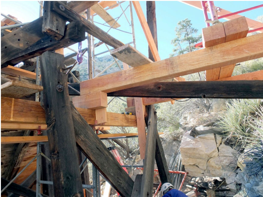
Figure 51: After the bent was stabilized, the intermediary sill could be removed.
