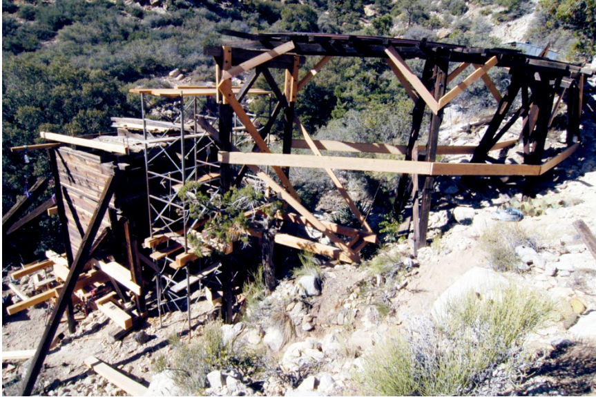
Figure 60: Replacement diagonal and longitudinal bracing installed between bents.
