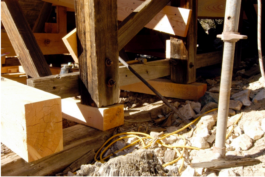
Figure 46: The two eastern hopper girders in the ore bin were decayed along their lengths and were replaced in kind.
