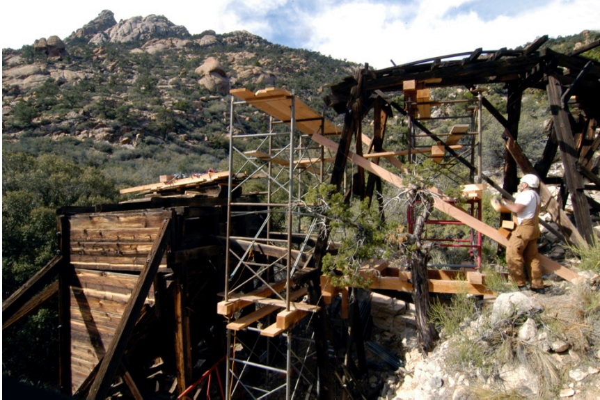
Figure 3: Structural staging was erected to support the structure.
