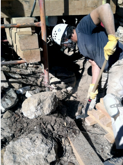
Figure 38: Digging out the remains of the subframe sill.
