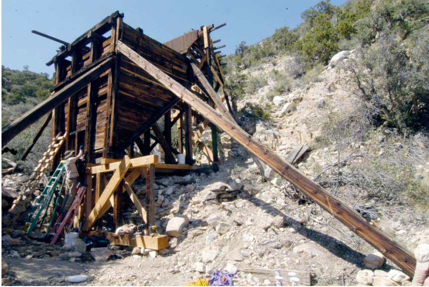
Figure 66: Once the repairs were completed, the hardware at the mouth of the ore bin, including a movable chute and lever, was reinstalled.
