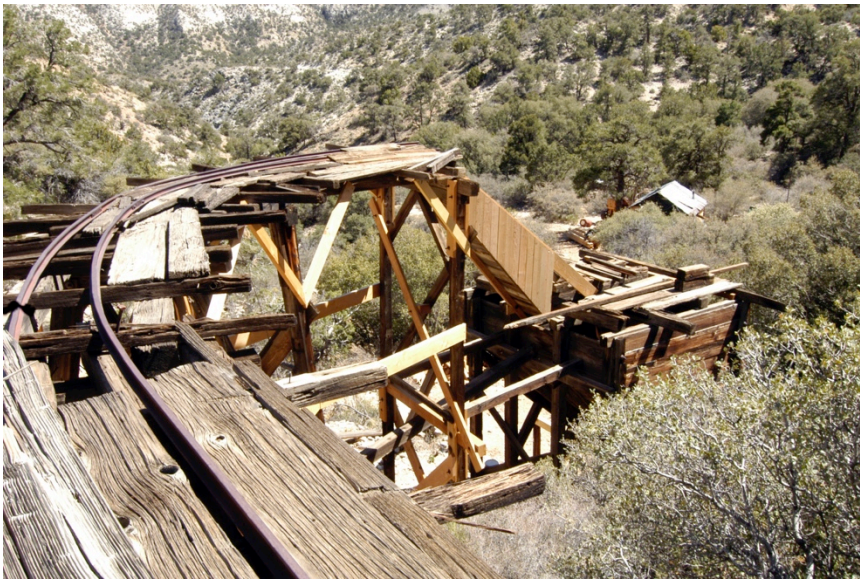
Figure 14: The completed ore chute. Enough of the ore chute was rebuilt to brace bent 1, and several members were in good enough condition to be reused. Surviving remnants were copied to sheath the sides.
