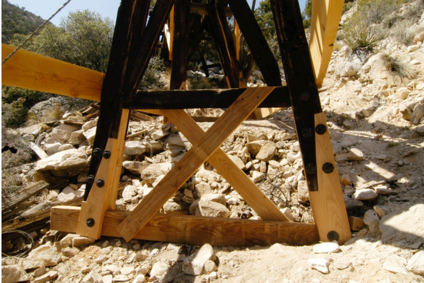
Figure 15: Scarfed repairs in bent 3. Lower cross bracing and the sill were replaced in kind. Spacers were added between the dimensional lumber posts between the scarfs to support the repairs.
