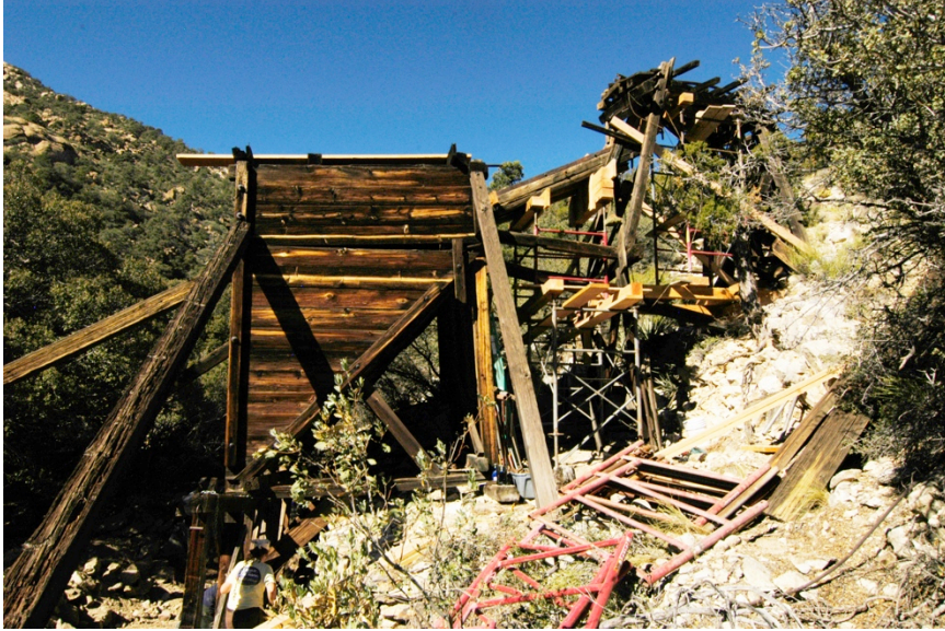
Figure 64: The ore chute, removed at the beginning of the repair work, was reinstalled during the second repair visit. The team was able to reuse several of the existing members to rebuild the base of the chute.
