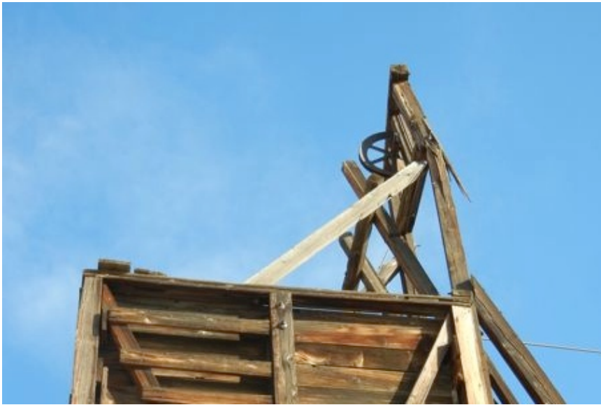
Figure 19: One of the columns supporting the sheave at the top of the structure has failed.
