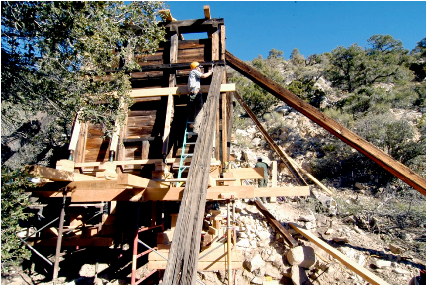
Figure 35: After the ore bin was repositioned, the long timber braces at the southeast and southwest corners were reset.
