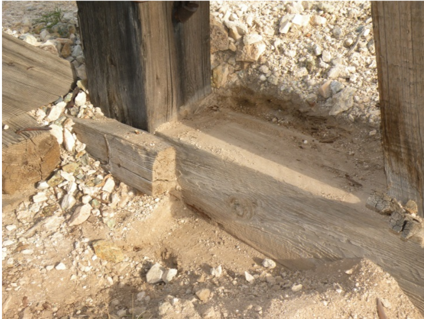
Figure 20: The interior of this sill has decayed, and leaves it providing little to no support for the columns and braces above.
