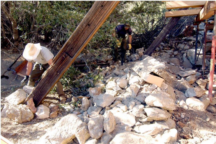
Figure 11: Resetting the ore bin braces after the bin was returned to a plumb condition.
