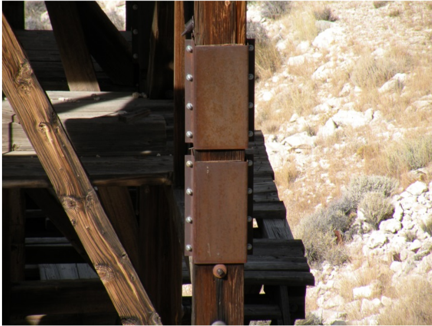
Figure 22: Steel plate clamps installed on columns will result in decay of the columns.
