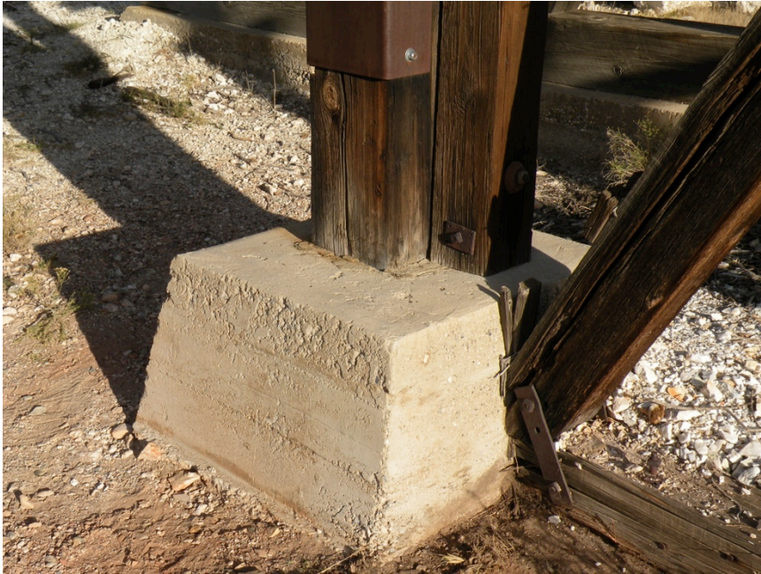
Figure 21: The base of the larger (12x12) column is decayed where it is embedded in the concrete pier. The diagonal brace terminating in the pier is deteriorated around its connection and has lost most or all of its original capacity.
