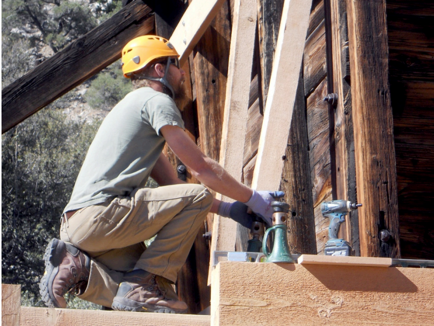
Figure 30: A temporary ledger was installed on the south side of the ore bin. Posts were set against the ledger and raised using screw jacks, lifting the south side of the ore bin. This allowed for repair work to the ore bin subframe and corrected the bin's out of plumb condition.
