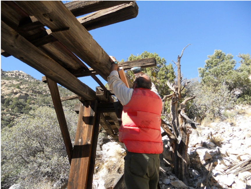
Figure 58: Diagonal and longitudinal bracing in the trestle provide stability in this portion of the mine structure. Many of the braces had partially or completely detached, and were damaged or decayed at their ends. Those braces that could not be securely reattached were replaced in kind.
