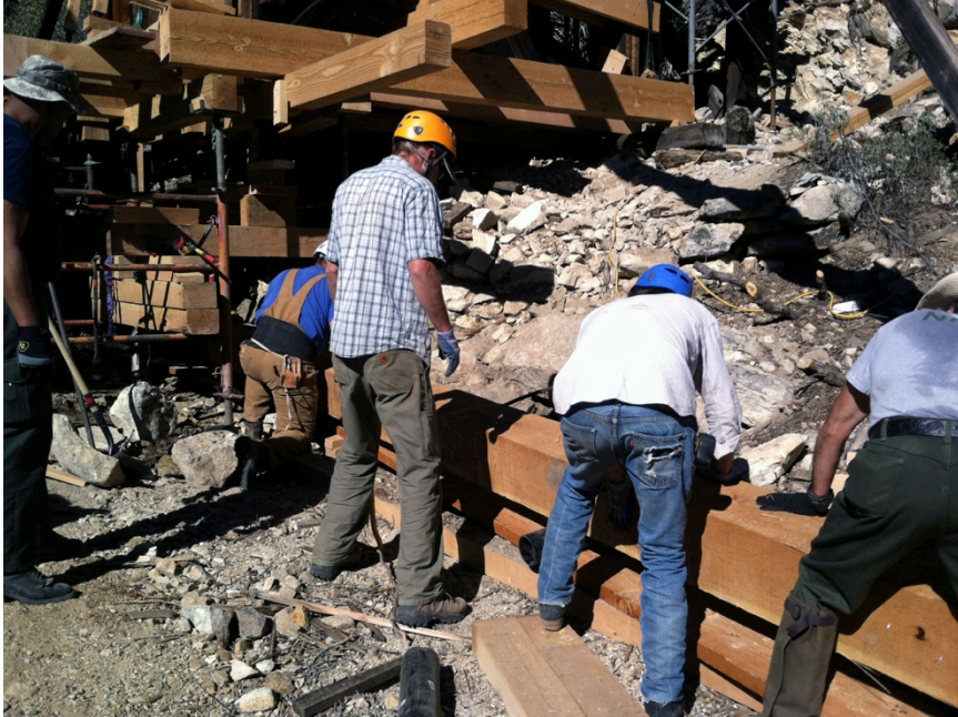
Figure 42: Positioning the replacement sill under the subframe.
