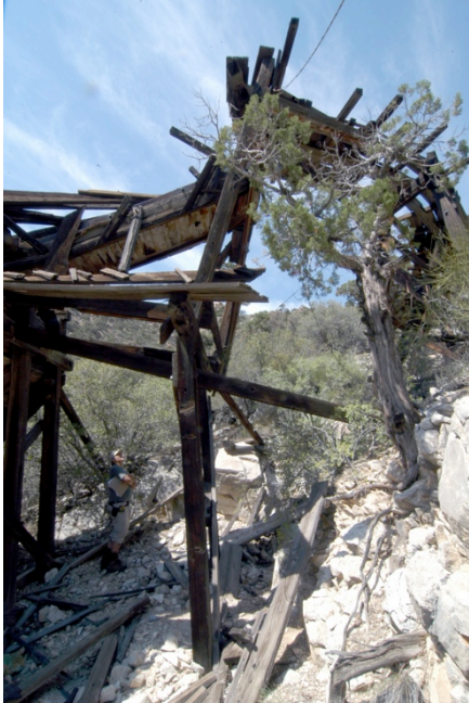
Figure 26: Rotation and subsidence in the ore bin had caused the tallest bent in the trestle, bent 1, to buckle at its intermediary sill.
