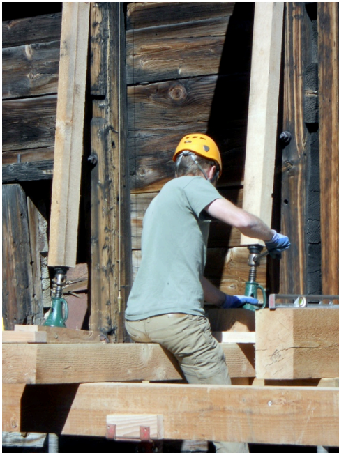
Figure 13: Using screw jacks to correct the alignment of the ore bin.
