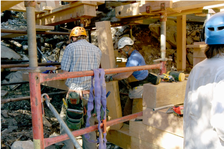
Figure 9: Setting the replacement post, second from the west, in the ore bin subframe. The first and second posts from the west were deteriorated along their lengths and were replaced in kind.
