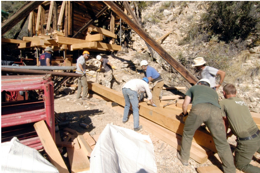
Figure 7: The replacement sill for the ore bin subframe was moved into place using ABS plastic pipe rollers
