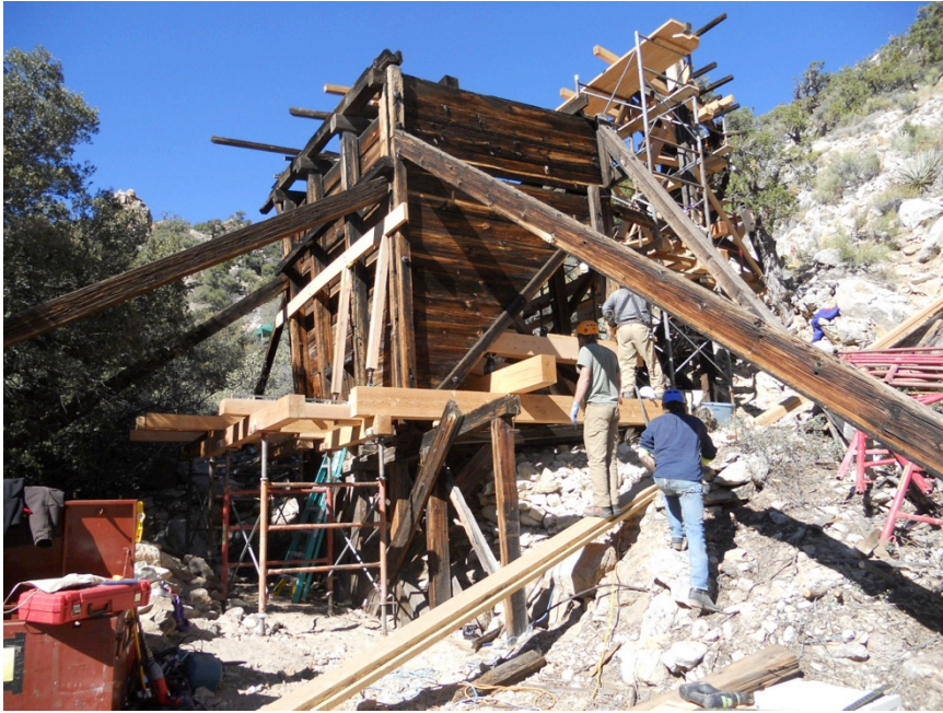
Figure 5: The south end of the ore bin was lifted using a combination of structural staging, cribbing, and screw jacks, allowing for repairs and plumbing of the subframe
