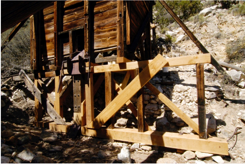
Figure 10: The completed subframe. The east half of the cap timber was replaced in kind, as were the two westernmost posts, and diagonal braces. New wood was scarfed into the end of the center post, and a column was added to the right to help support the end of the replacement cap timber.
