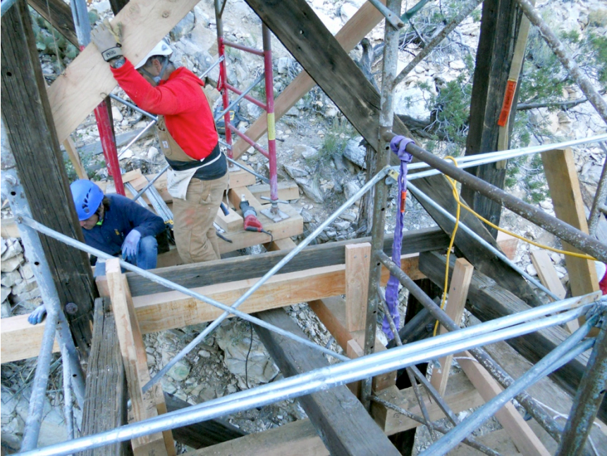
Figure 144 Once the replacement intermediary sill was installed, braces could be reset or replaced when damaged.
