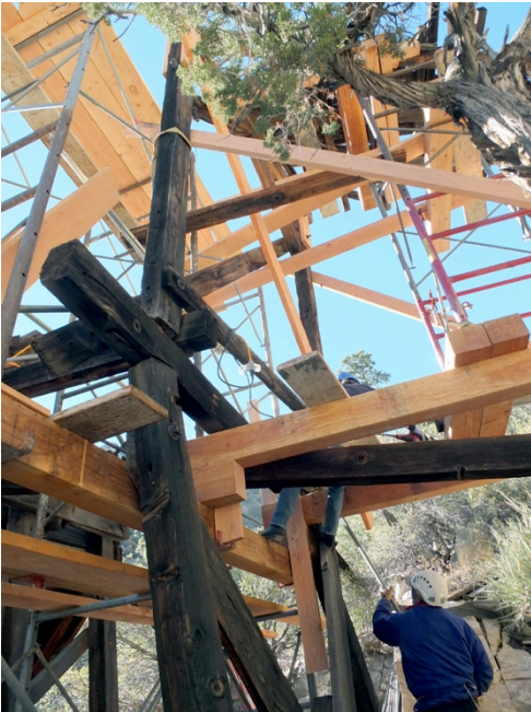
Figure 49: Subsidence and rotation in the ore bin had caused bent 1 to buckle. Structural staging and cribbing stabilized it so repair work could be completed.
