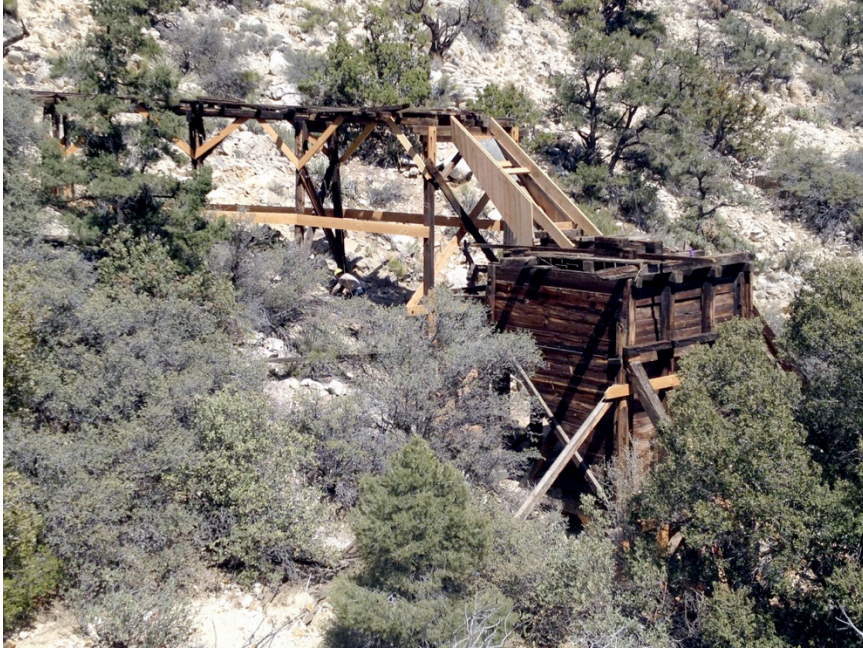
Figure 68: The Live Oak mine structure after completion of repair work
