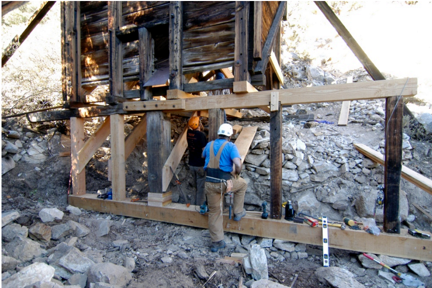
Figure 47: All four of the braces connecting the hopper girders to the subframe were in poor condition and were replaced in kind.
