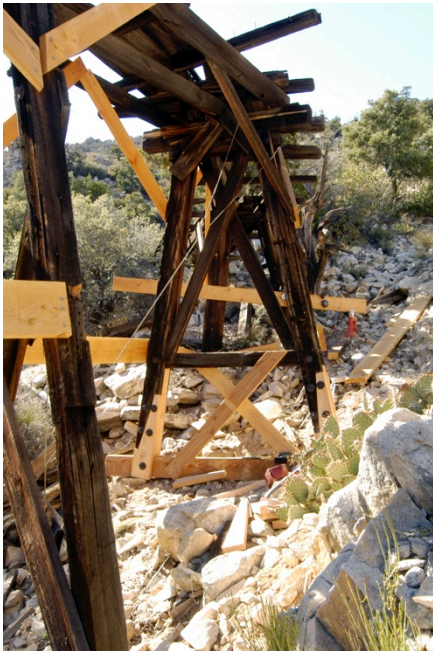
Figure 63: The lower set of cross bracing in bent 3 was decayed and was also replaced in kind.
