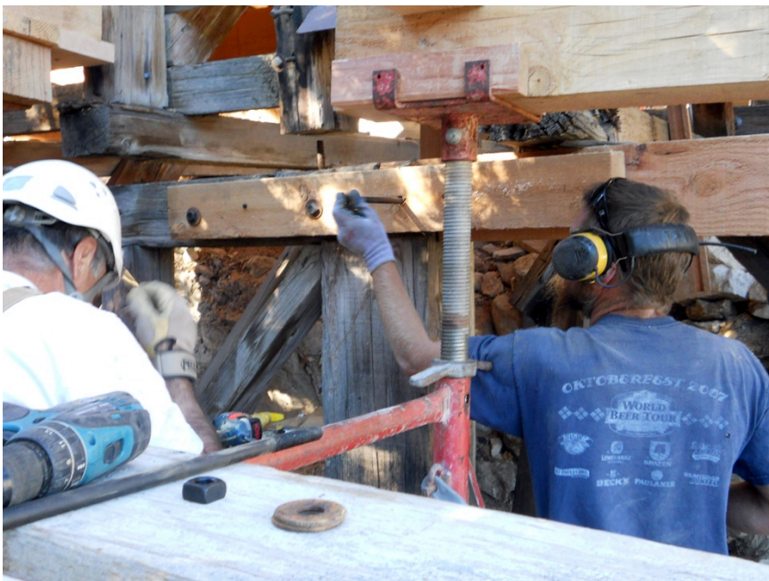
Figure 33: Hardware is installed through the cap beam and the brace on the far side.
