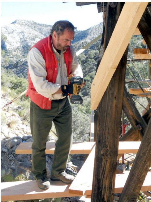
Figure 59: Attaching a replacement diagonal brace between bent 3 and the stringers above. Bracing was attached using corrosion-resistant structural screws.
