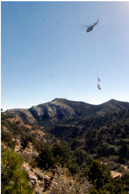
Figure 67: The remoteness of the site and the difficulty of the terrain necessitated the use of a helicopter to transport bulky equipment, timber, and supplies.
