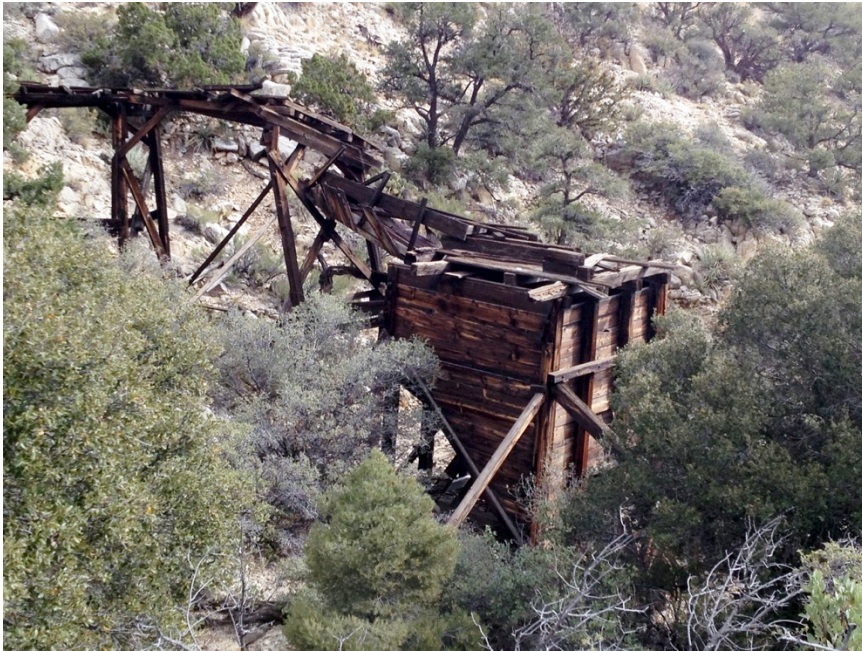
Figure 24: The Live Oak mine structure in 2014, prior to repair work. View from the southwest.
