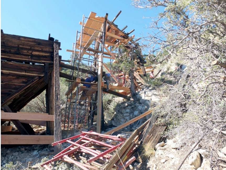
Figure 50: Staging provided access to both sides of the bent and to the intermediary sill located halfway up the structure.
