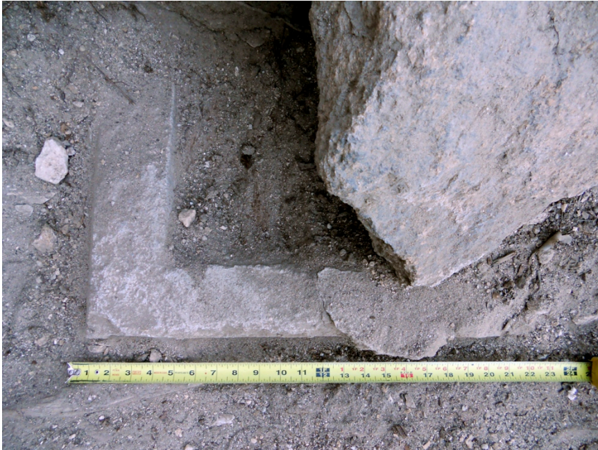
Figure 39: Two small concrete footers were uncovered during the removal of the decayed sill, and may have been used to provide additional support to the sill. The footers were left in place. See Appendix B, sheet XXX for approximate locations of the footers.
