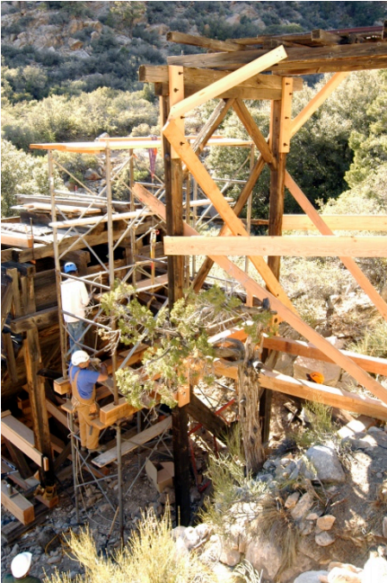
Figure 55: Three diagonal braces and all of the vertical braces connecting the cap beam and the upper posts and the intermediary sill and the lower posts were damaged and were replaced in kind.
