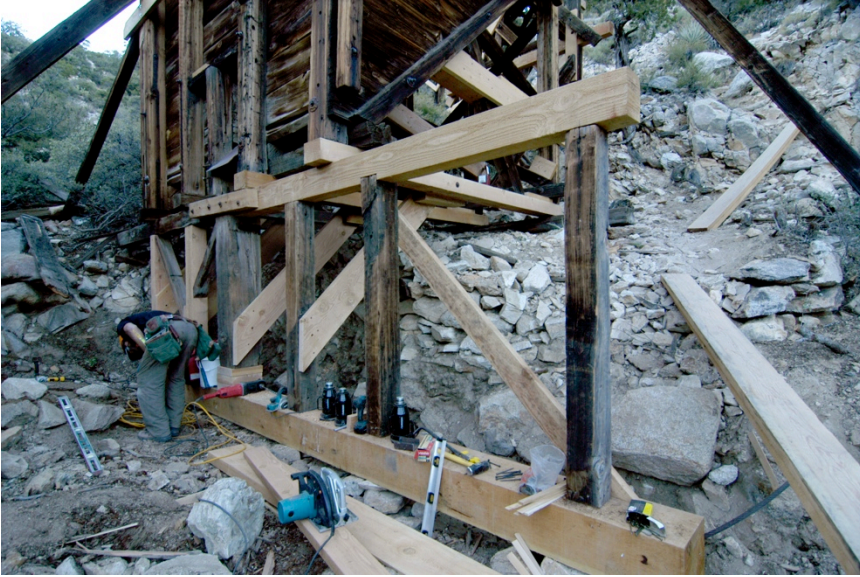
Figure 48: Much of the smaller diagonal bracing (at front) in the subframe was also decayed or damaged. Members were either reattached or replaced in kind.
