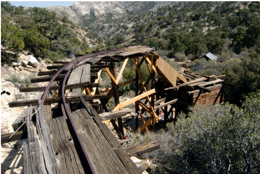
Figure 65: The reinstated ore chute viewed from the northwest.
