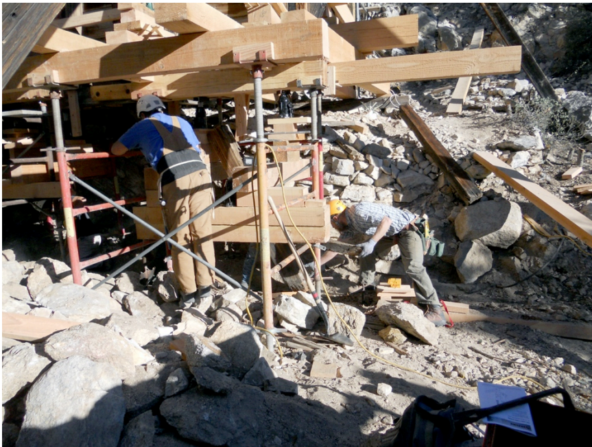
Figure 37: The ore bin subframe sill was largely lost to decay, and was replaced in kind. Here, remnants of the sill are removed.
