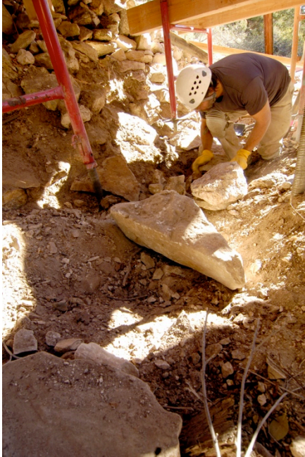
Figure 40: A dry stacked stone foundation was constructed under the subframe prior to the installation of the replacement sill. The stone will facilitate drainage and help to slow deterioration.
