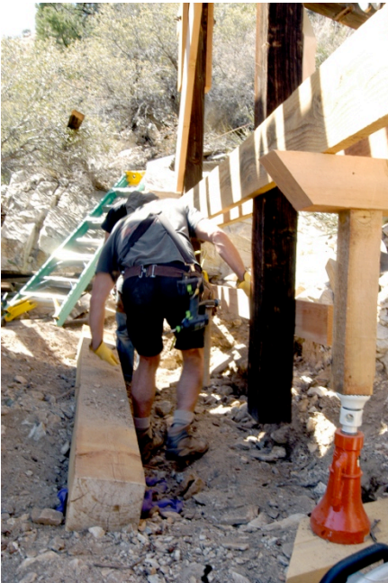
Figure 57: During the second repair visit, the sill for bent 1, which had been largely lost to decay, was replaced in kind.
