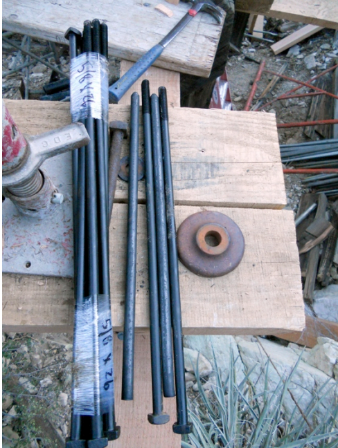
Figure 34: Hardware for the repairs was a combination of existing pieces and custom-made reproductions
