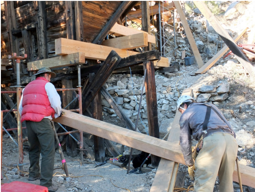
Figure 27: Setting up structural staging and cribbing in front of the ore bin. This framework supported the structure during repair work and provided access to different parts of the structure.
