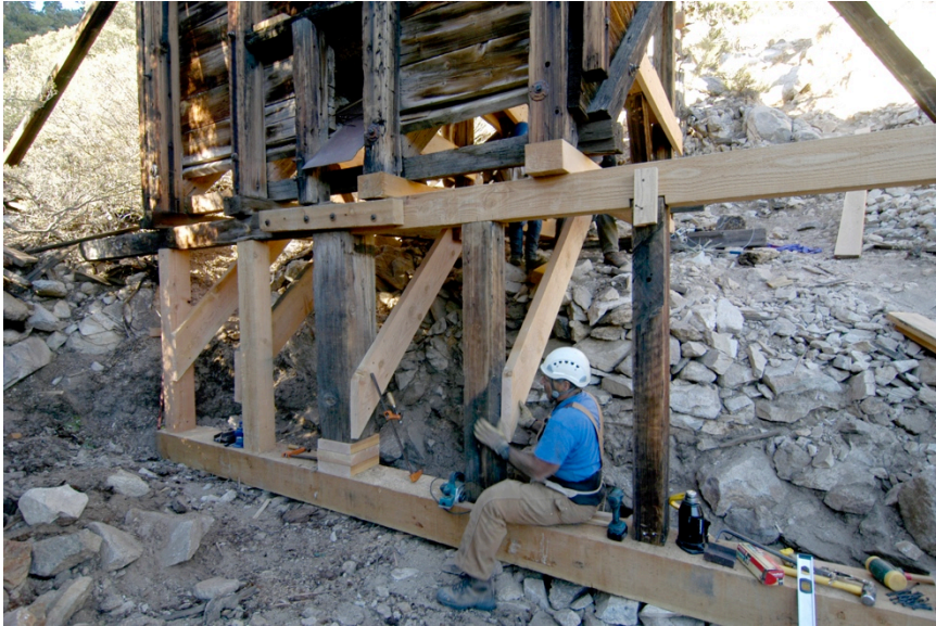
Figure 6: Replacing the braces between the hopper girders and the ore bin subframe. The two easternmost hopper girders were deteriorated along their length, and were replaced in kind (ends visible above the subframe).
