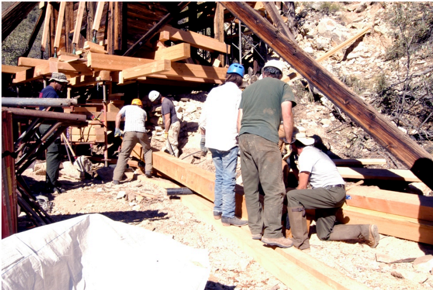
Figure 41: Installing the replacement sill. The replacement was moved into position under the subframe using a dimensional lumber roadway and ABS plastic pipe rollers,.
