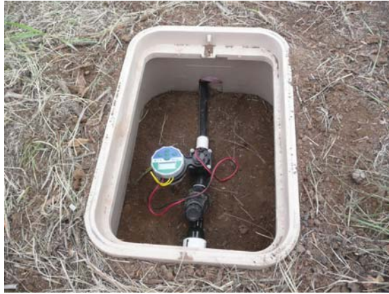
Irrigation valve box
