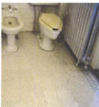
Poorly repaired floor
