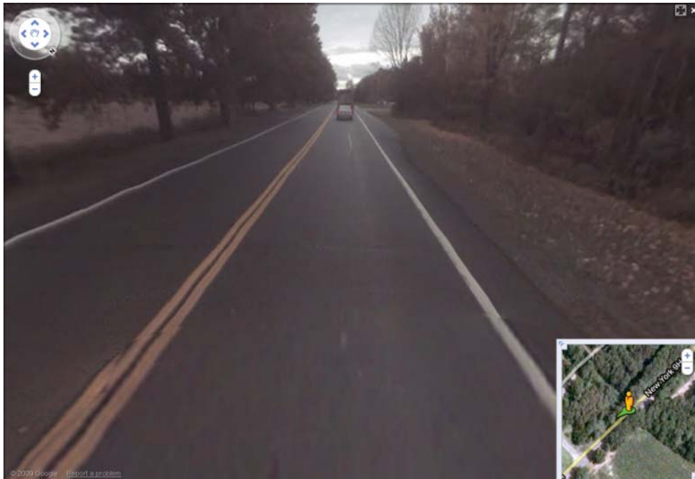
Figure 38 SR 9H approach north of the park showing shoulder width change Source: Google Maps, 2010
