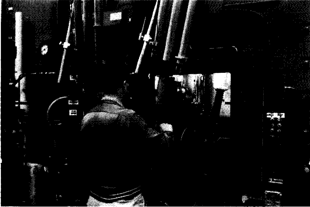
Above, a worker operates the state-of-the-art hydraulic manipulators at the face of a hot cell in the 325 Radiochemistry Building in the 1950s. Below, a HAPO-1-A Cask arrives at the entrance to the rear face of the three large new hot cells in the building in 1961. The cask contained radioactive material being used in pioneering "isotope campaigns" at the Hanford Works.
