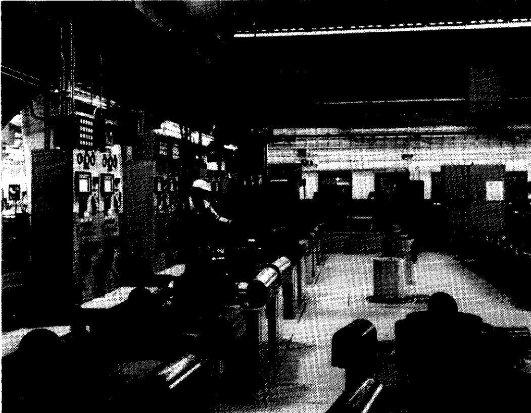
The autoclave inspection area in the 333 Fuels Manufacturing Building, 1984.
