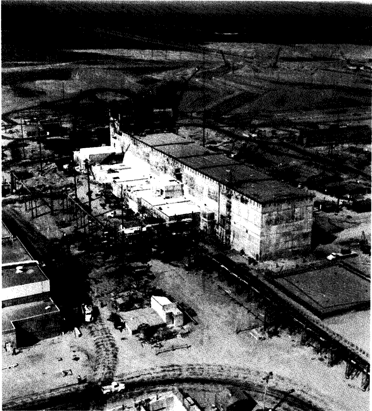
The REDOX Plant under construction in Hanford's 200 West Area in 1951. The unique chemical process used in the REDOX facility was developed in the 3706 Building and first tested in the 321 Building.
