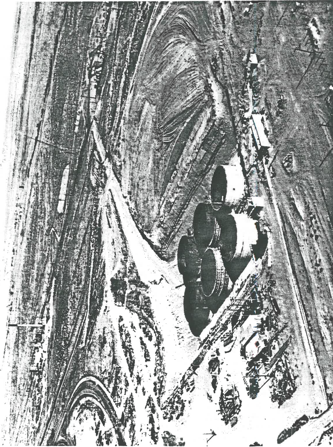
Figure 11. 241-A Tank Farm, for the storage of high-level wastes from the PUREX Plant, under construction, July 1954.
