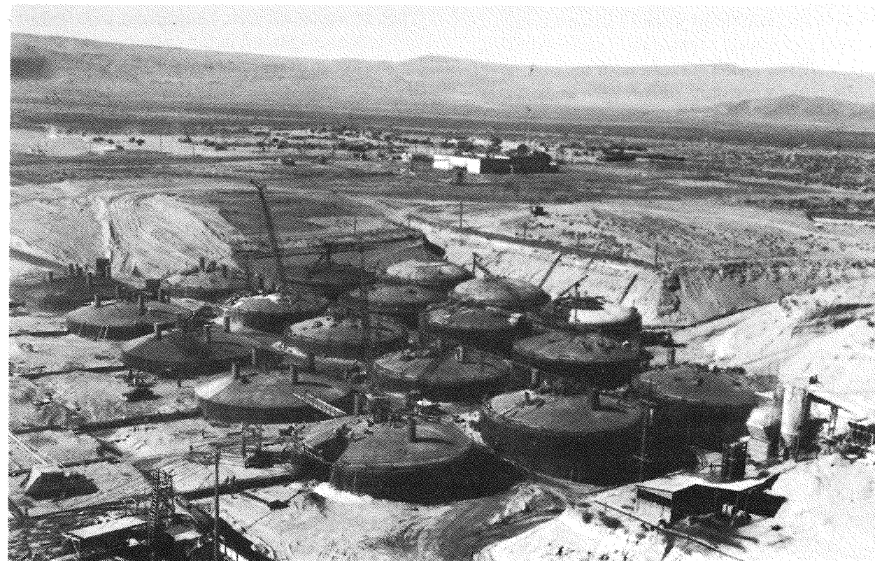
The 18 single-shell tanks of the 241-TX Tank Farm take shape, July 1948.
