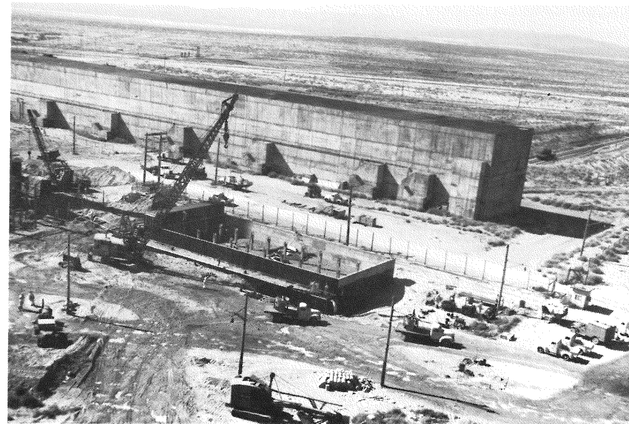
Sand filter bed being emplaced at T Plant in 1948.
