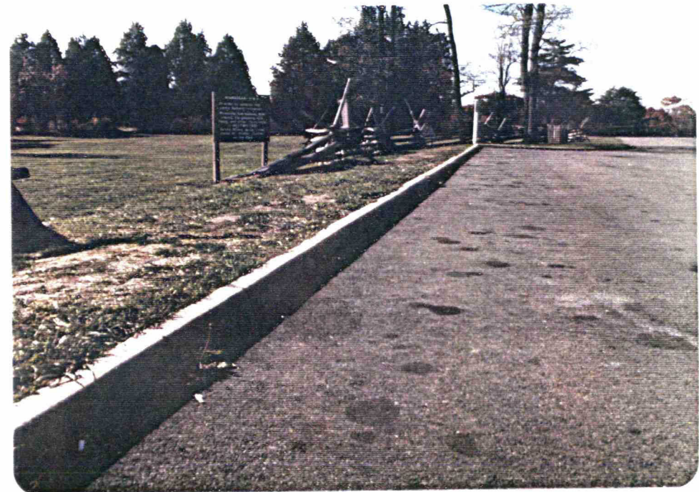
Curb along Rte. 13 Turnout
