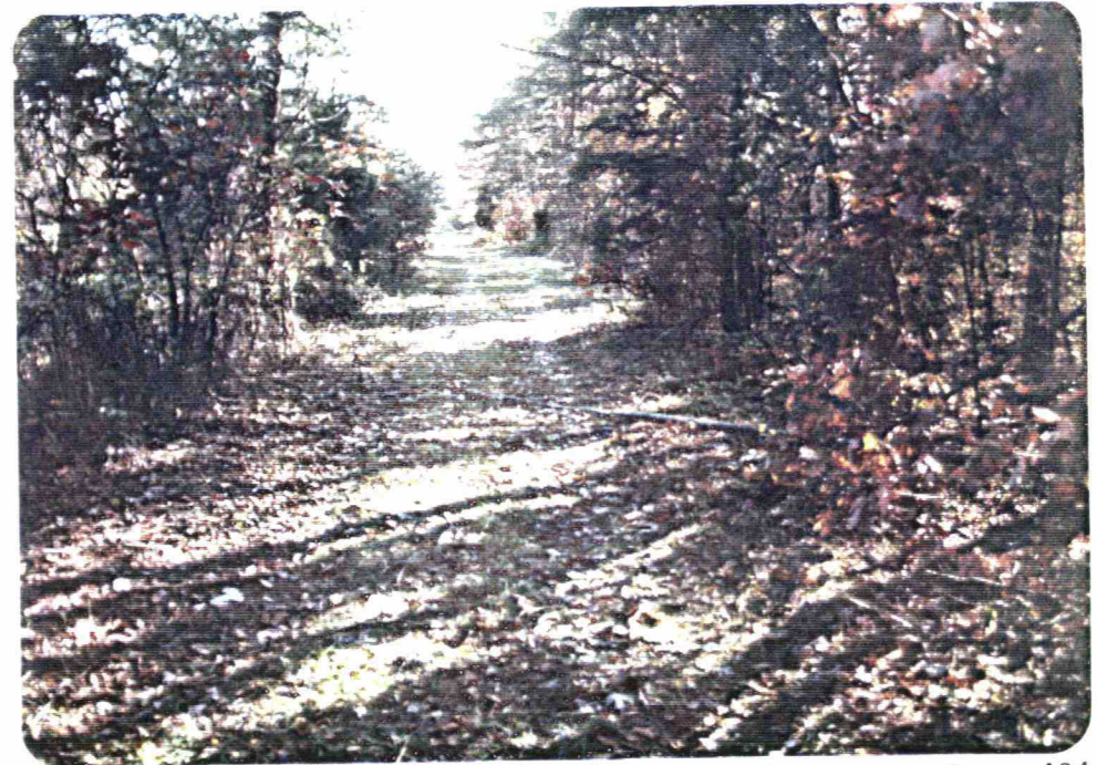
Trees and Other Vegetation Encroaching upon Rte. 404
