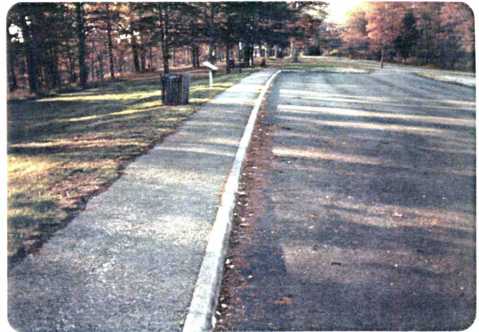
Bituminous Sidewalk along Rte. 14
