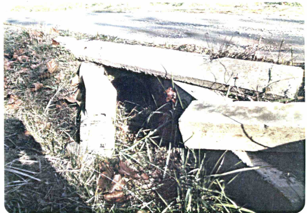
Culvert Outlet at MP 0.17 on Rte. 406
