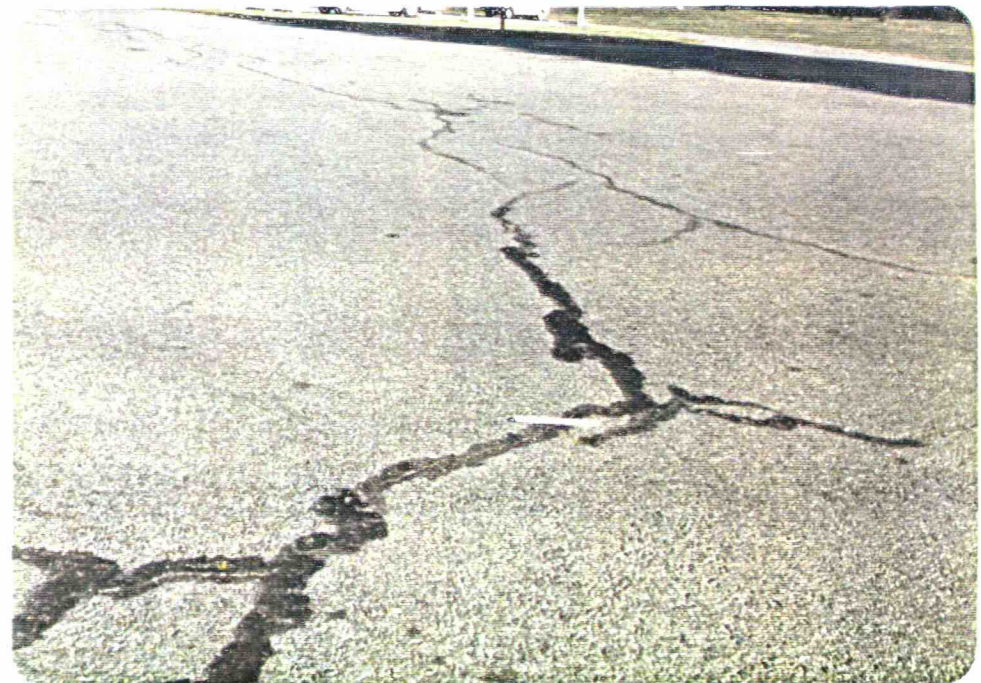
Sealed Cracks on Rte. 10
