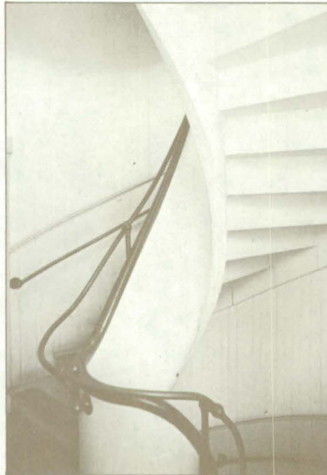
Stairway at the mills.
