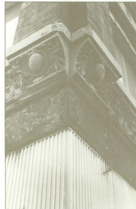
Aluminum meets brownstone: Prior to the renovation of the Fairburn Building.
