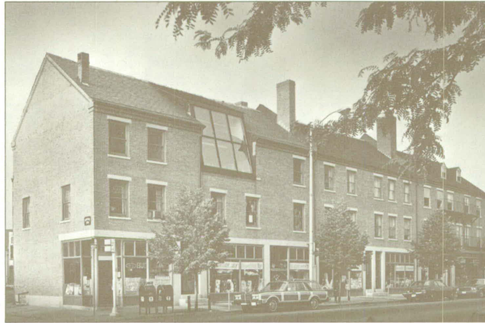
The Bank Block, ca. 1826, rehabilitated in 1976.
