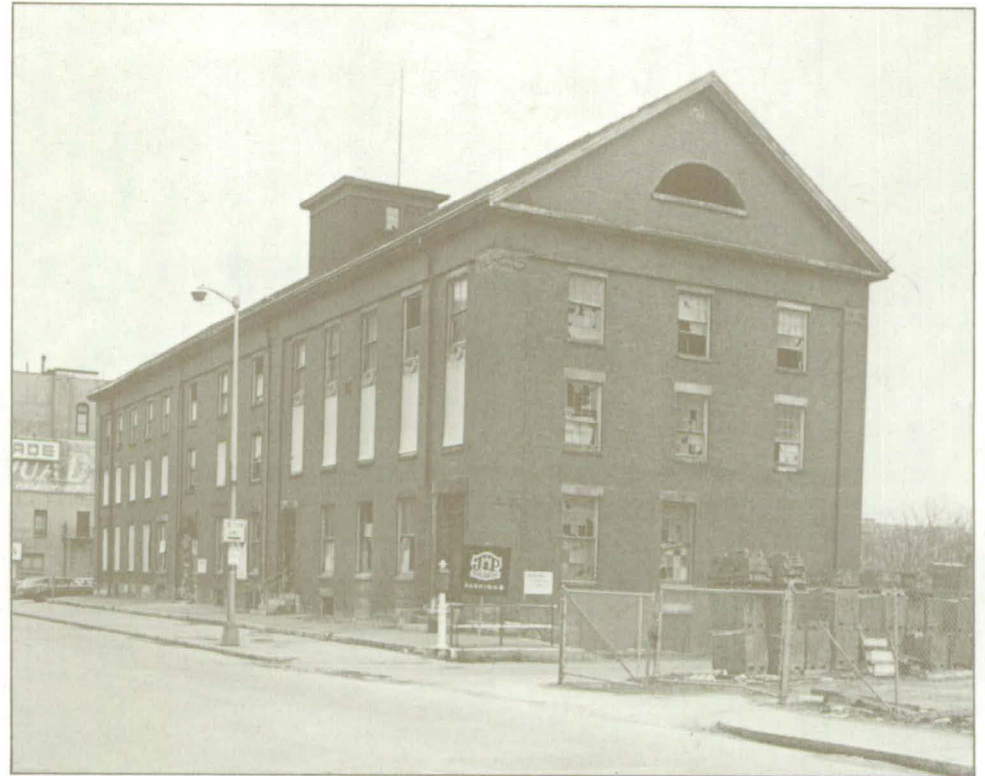
A low interest loan from the LDFC will help make this renovation possible.
