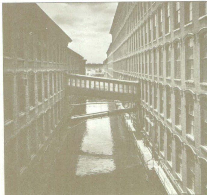
Surviving mill buildings are among Lowell's most important architectural assets. It is imperative that their historic character be preserved.
