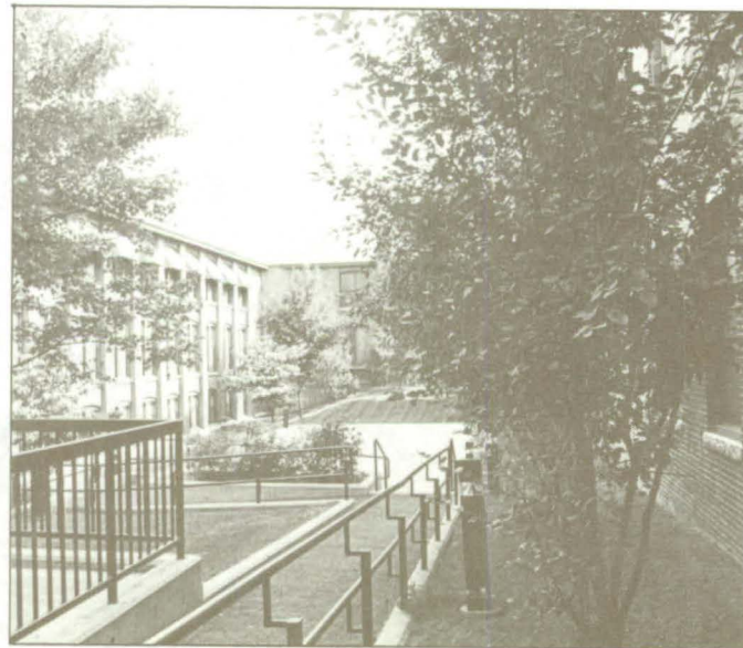
The millyard of the Pilling Shoe Mill was recycled to maintain its historical integrity while providing an outdoor area for elderly residents.
