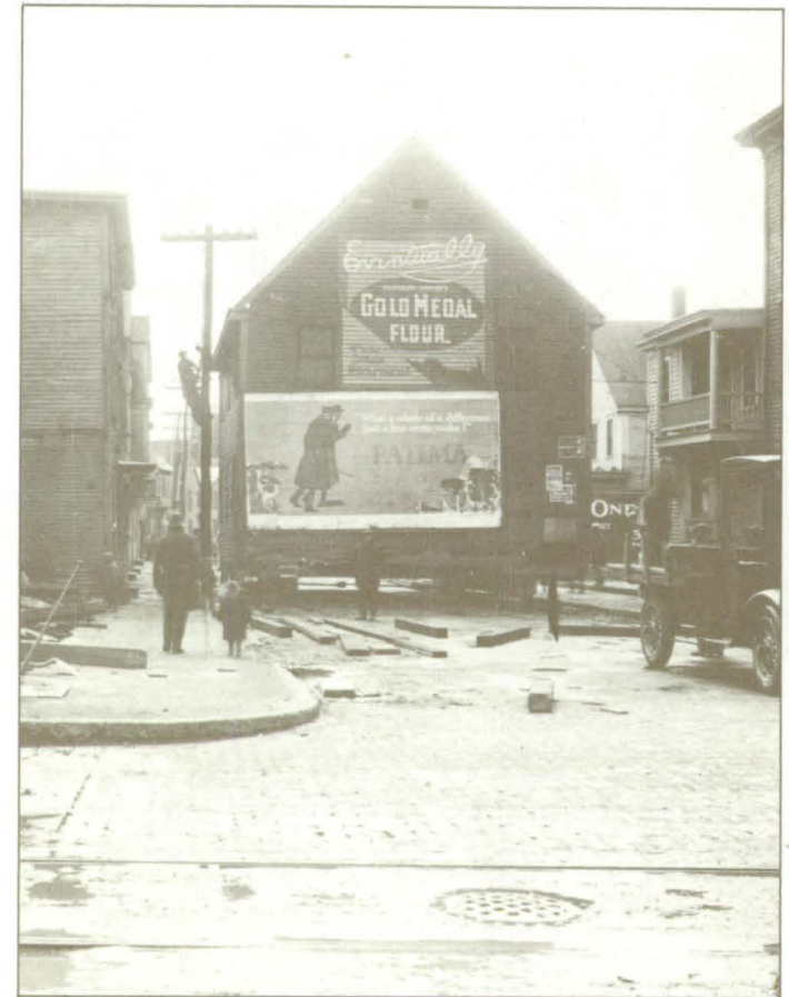
Relocating buildings is an old American practice and also occurred in Lowell. As a last resort to demolition, relocation may need to be considered.
