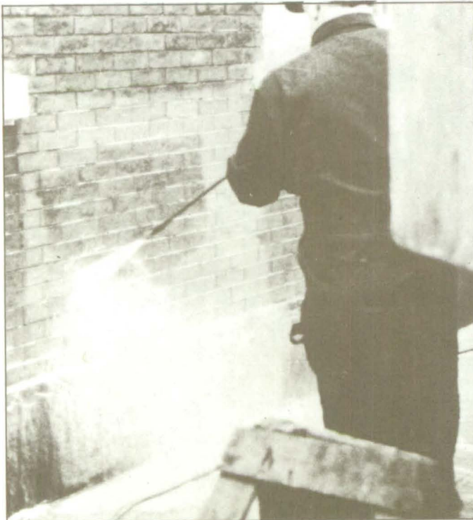
A cleaning test patch of the soiled masonry of the Gas Light Building will help determine the proper method for cleaning. Here the previously applied dilute acidic chemical is being pressure rinsed.
