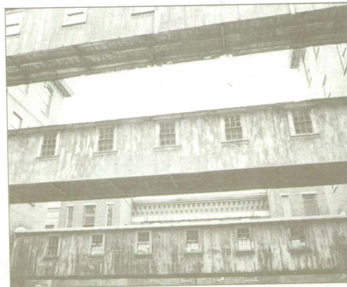
Enclosed millyard bridges were commonly employed to move materials between buildings.
