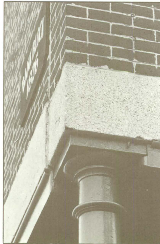
Three prolific building materials of the 19th century, pressed brick, granite and cast iron are juxtaposed in a typical manner on the Bank Block. The conservation of historic building materials is the basis of preserving Lowell's architectural heritage.
