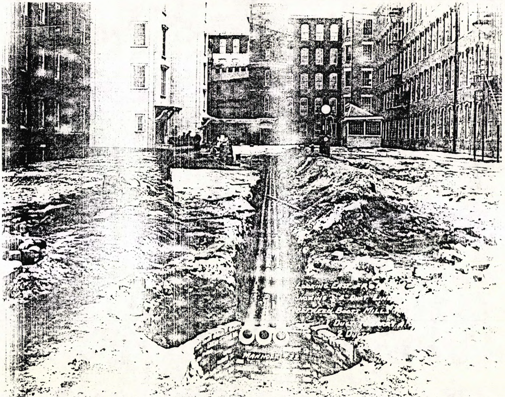
30. Mill yard between Boott Mills Number 1 and 2 and Number 6, Dec. 1933 Note fire stair at west end of Number 6, accessory structure at elevator
