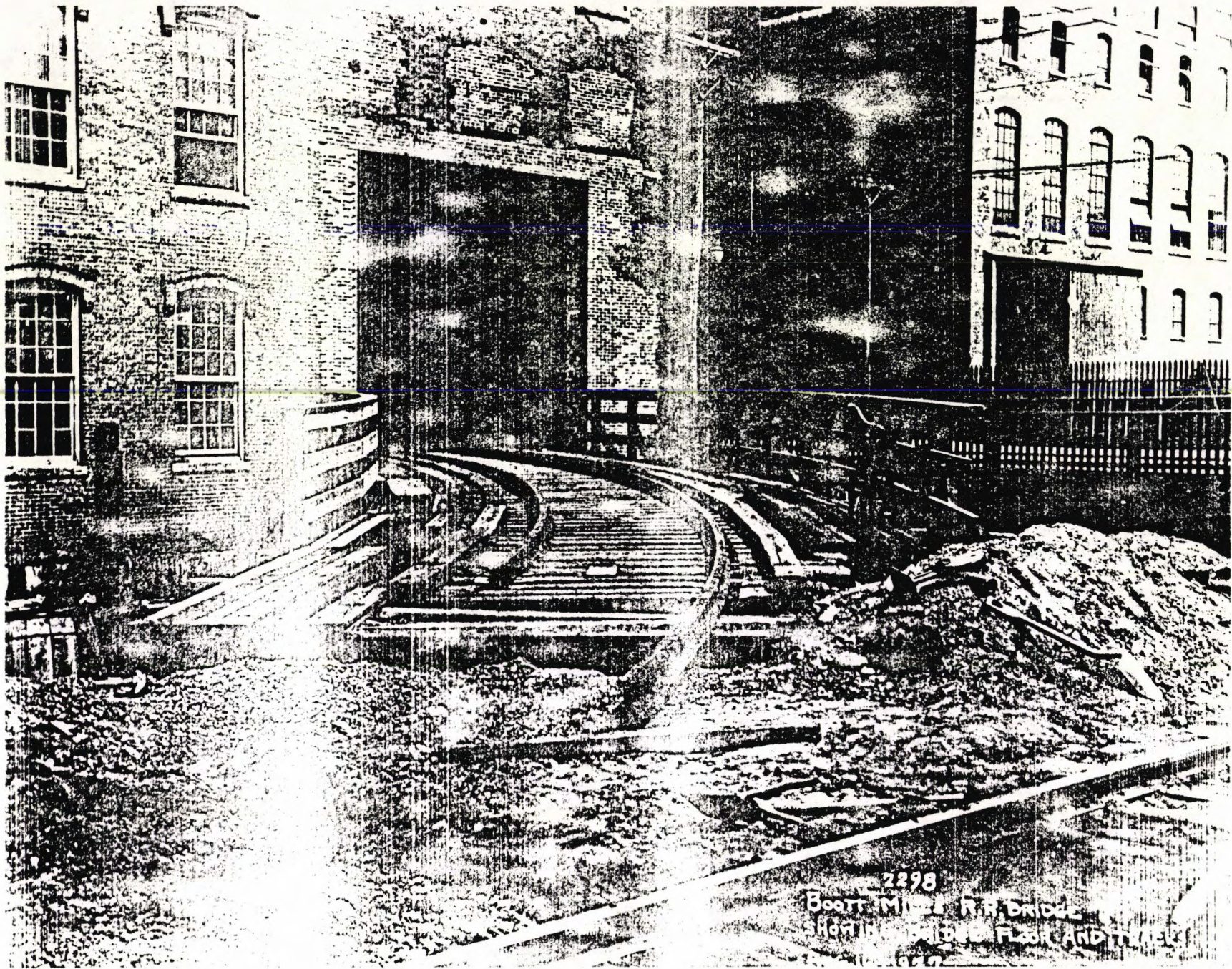
27. "Boott Mills Railroad Bridge Showing Bridge Floor and Tracks, Aug 1927."
