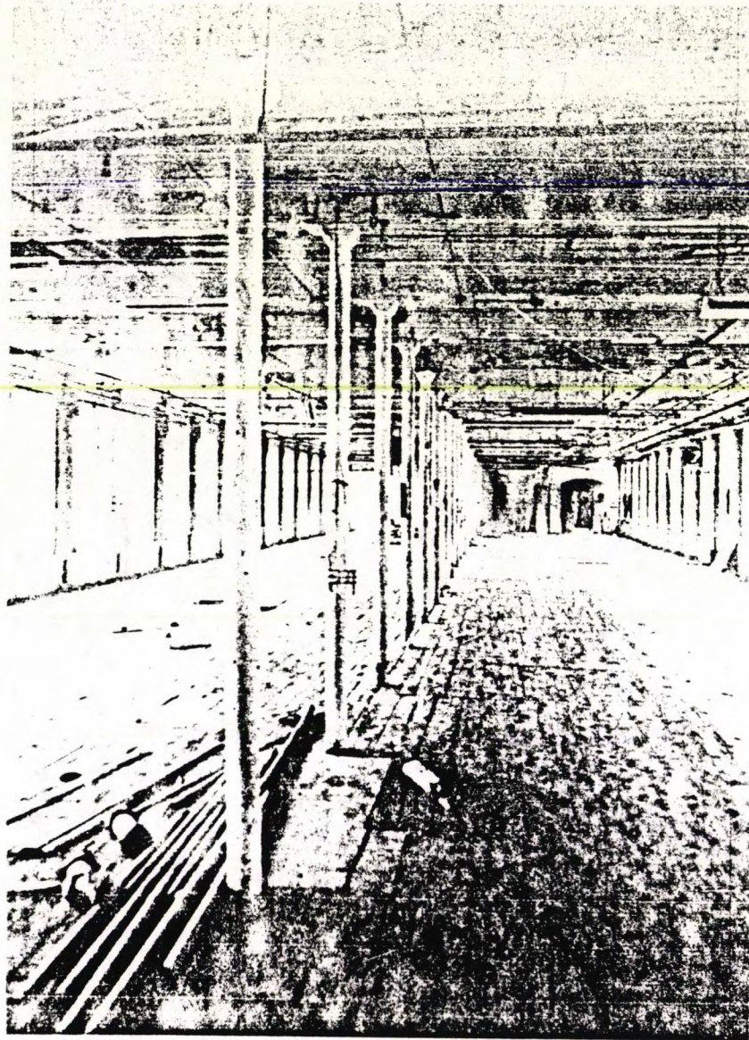
20. Cast iron columns at first floor of Boott Mill Number 6, June 1985
