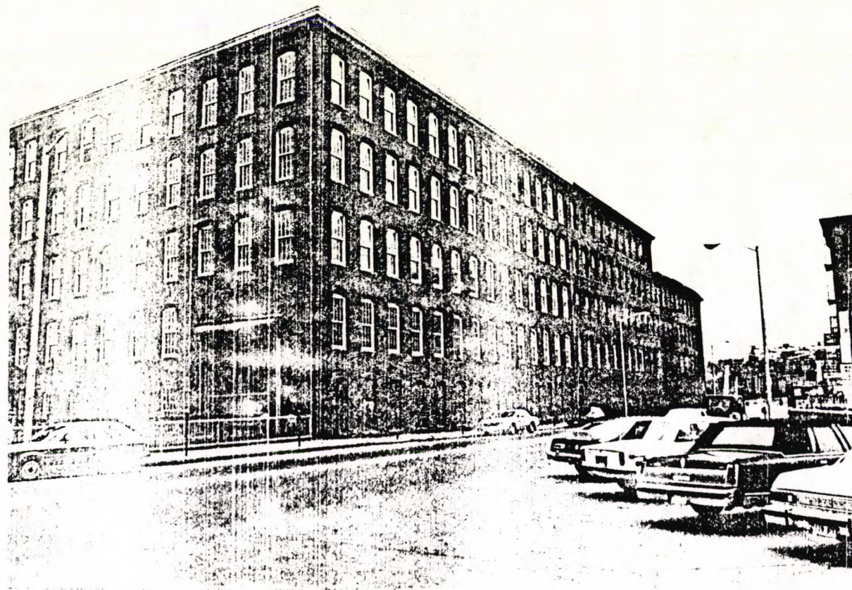
16. Bridge Street facade of Number 6 with blind arcade, June 1985
