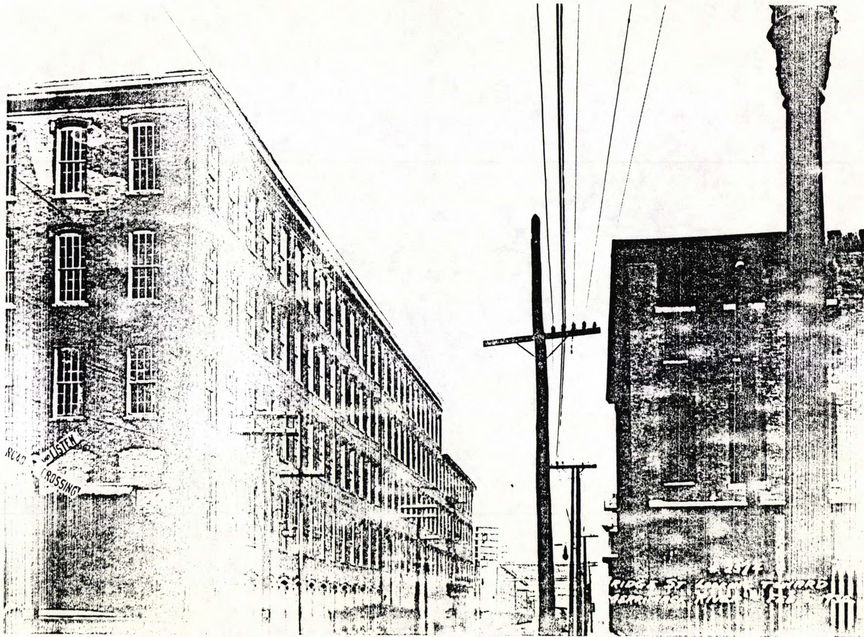
15. "Bridge Street Looking Toward Merrimack River, February 5, 1930" Note blind arcade of Bridge Street elevation of Mill Number 6
