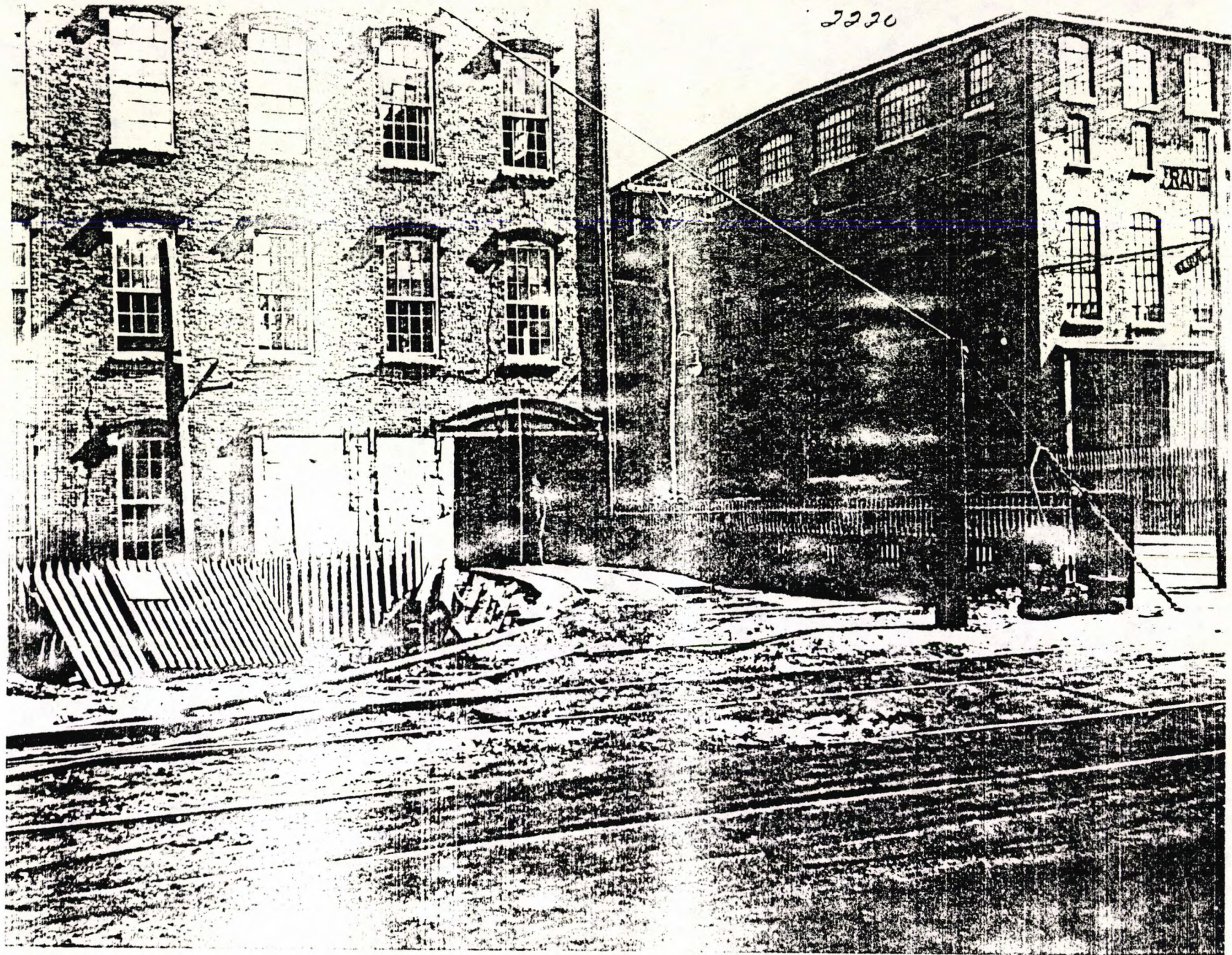
18. Side Track and Bridge to Coal Pocket of Boott Mill, Sept. 3, 1926" showing original design of Coal Pocket and sliding door
