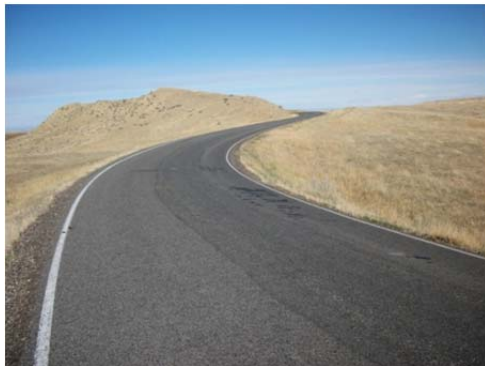
Tour Road. Source: URS Corporation
