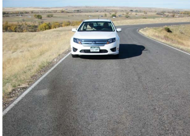
Narrow Tour Road Is Difficult for Two-way Traffic. Source: URS Corporation
