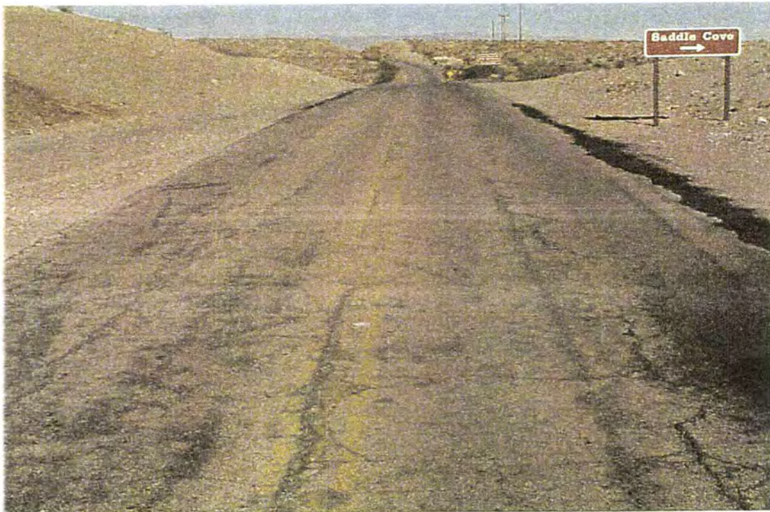
Photo #1635 - MP 5.32 - Pavement Change
