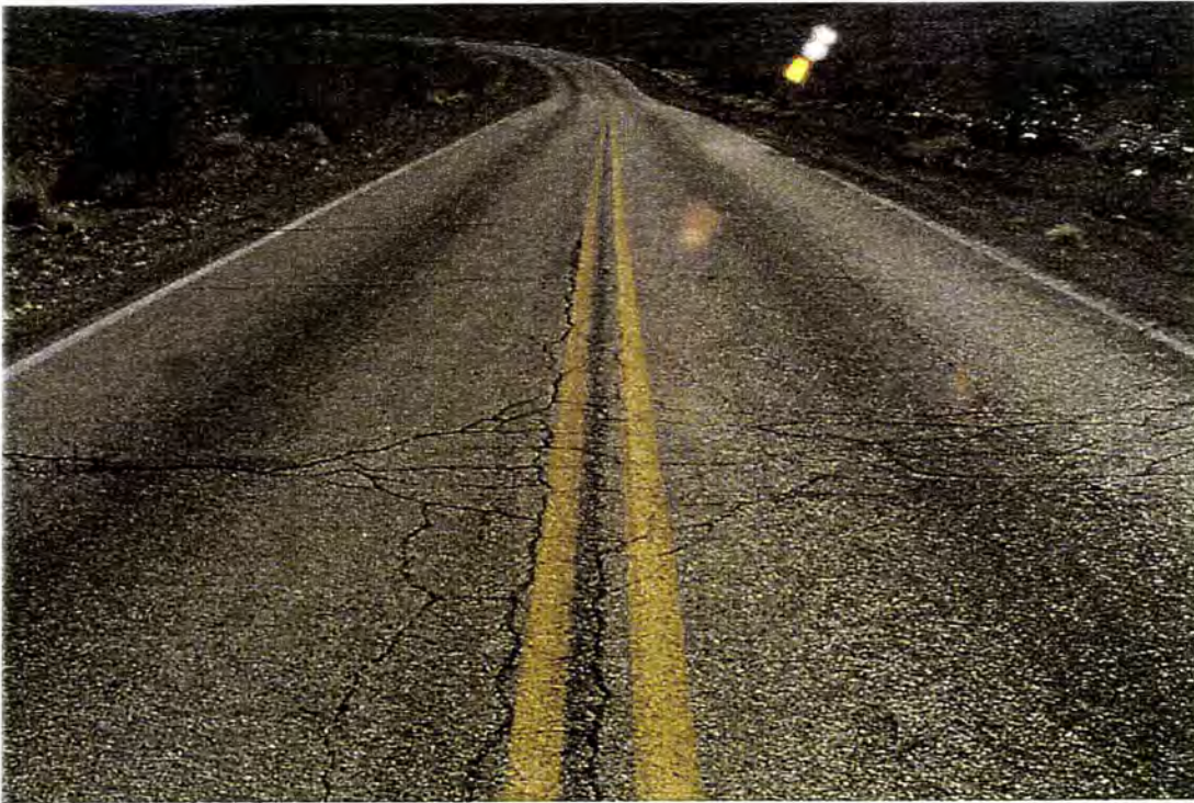
Photo #1676 - MP 12.50 - Reflective Cracking
