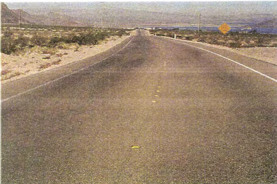
Photo #1633 - MP 0.70 - Typical Pavement Section
