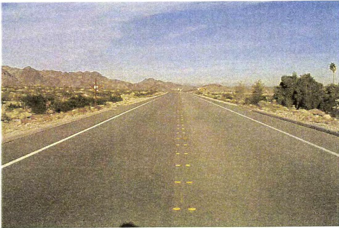
Photo #1634 - MP 2.56 - Typical Pavement Section
