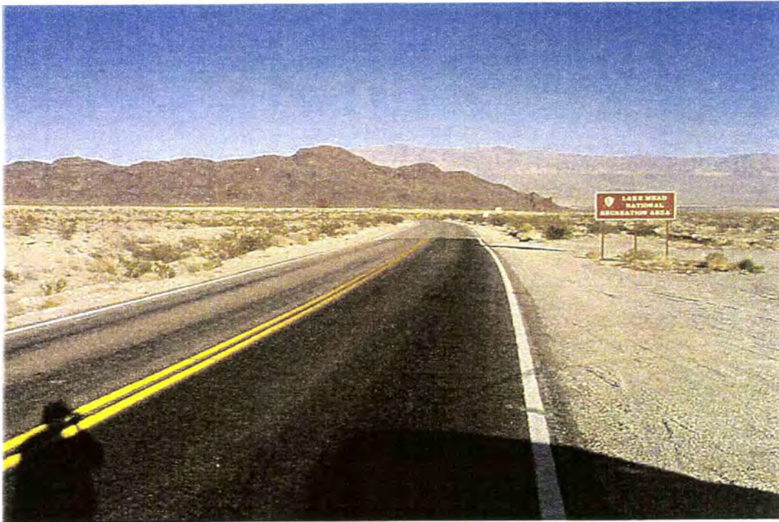
Photo #1687 - MP 0.00 - Begin at West Boundary
