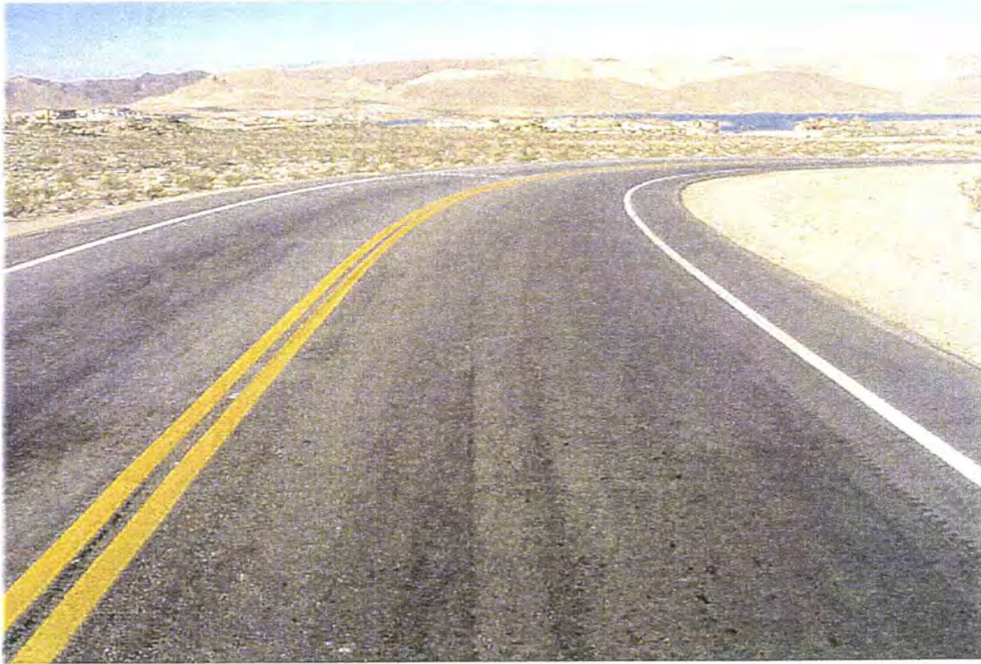
Photo #1618 - MP 0.00 Northshore Road - Typical Pavement Section
