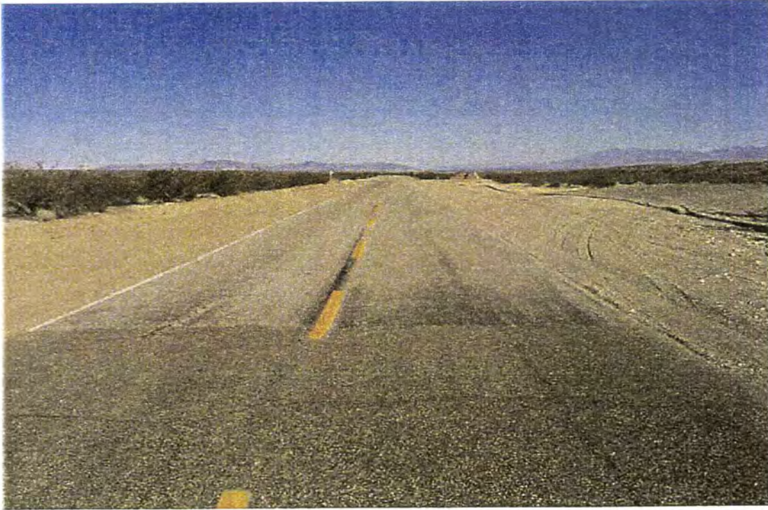
Photo # 1674 - MP 0.00 - Begin at South Boundary
