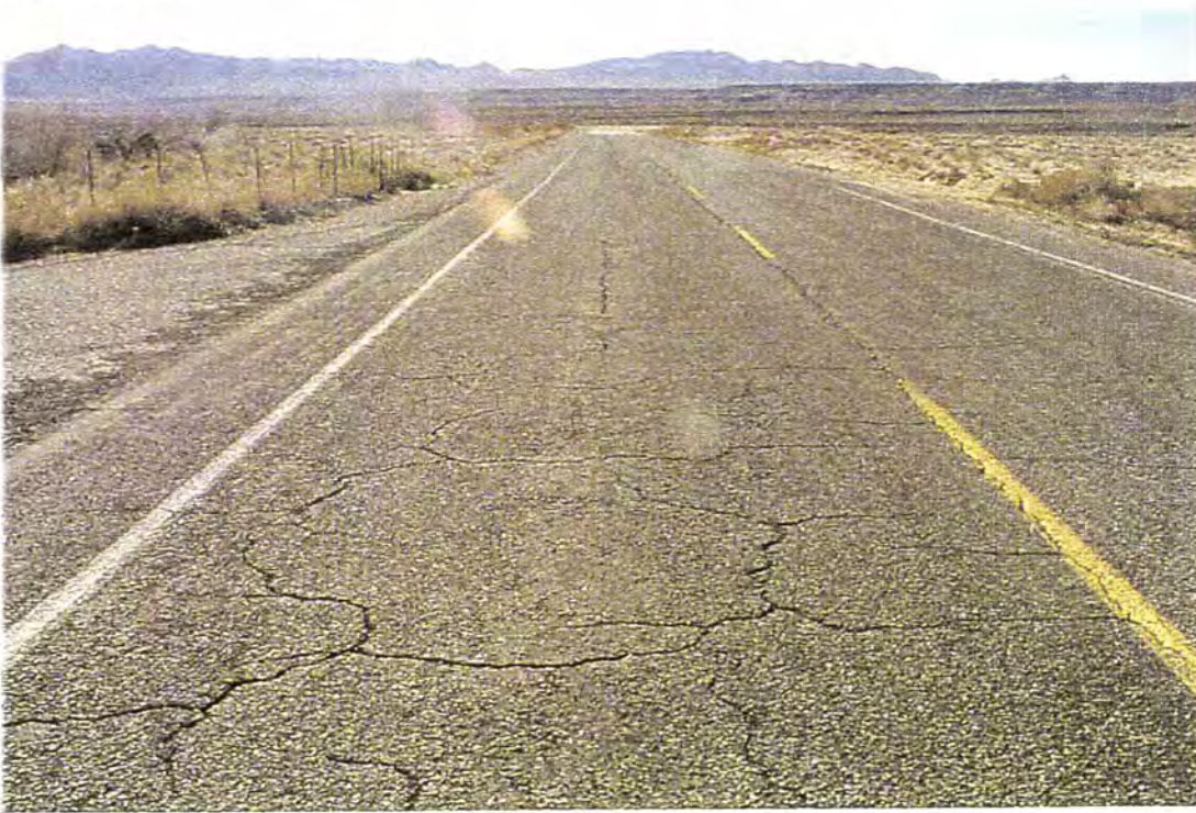
Photo #1625 - MP 39.50 - Pavement Change
