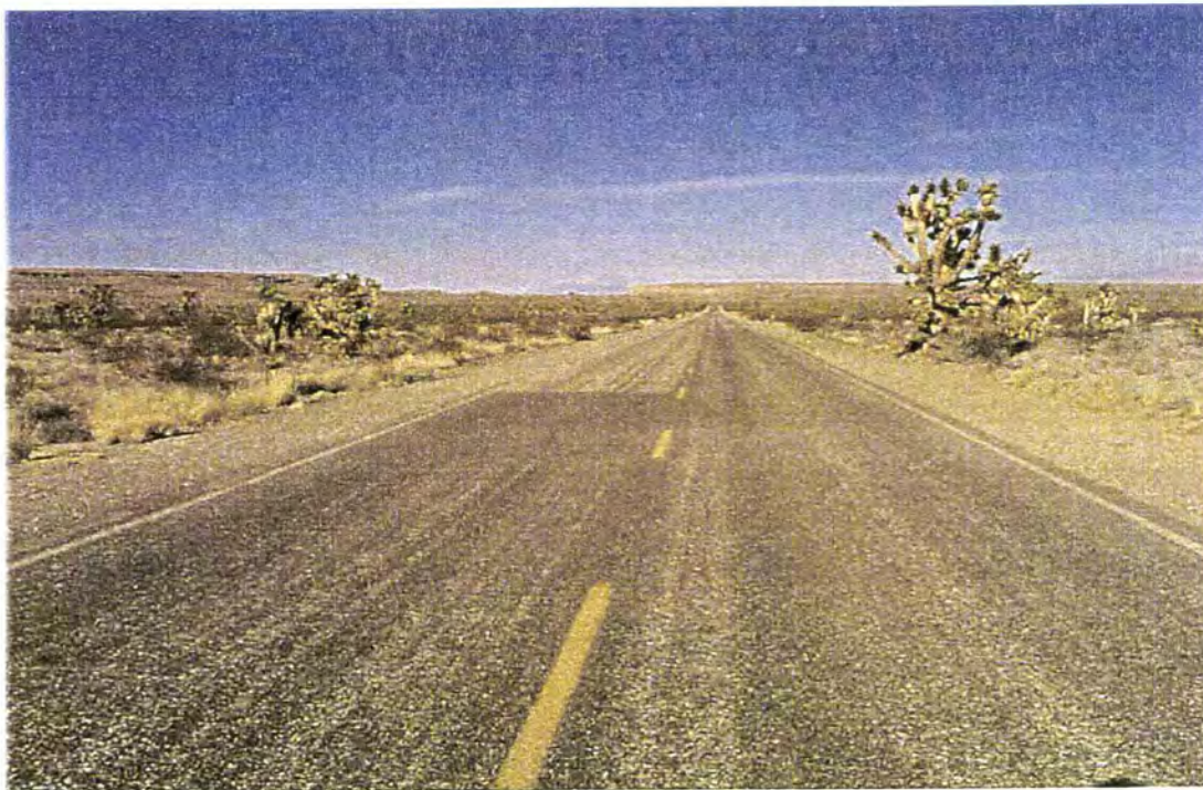
Photo #1665 - MP 6.16 - Pavement Change
