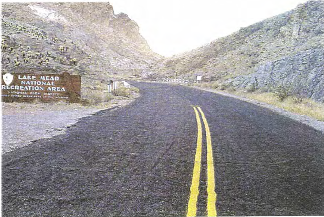
Photo #1690 - MP 0.16 - Typical Pavement Section
