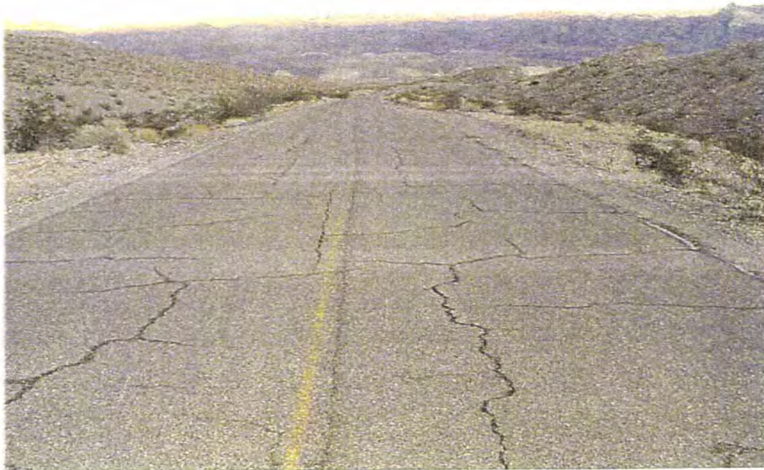
Photo #1691 - MP 1.90 - Typical Pavement Section
