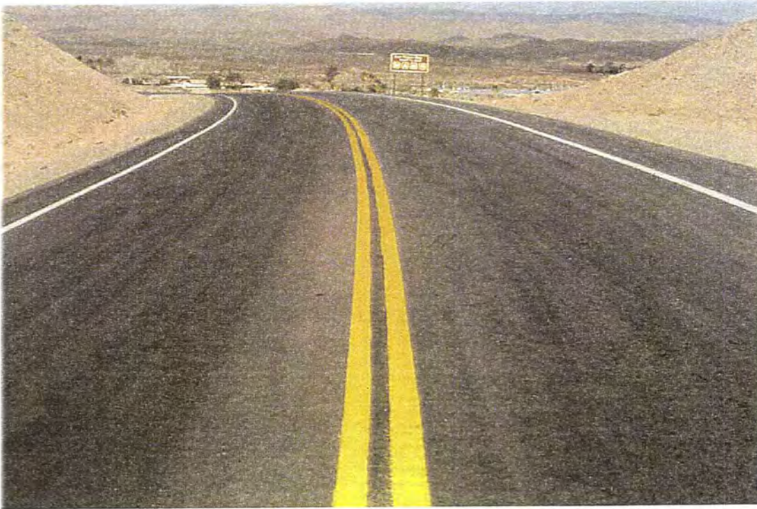
Photo #1636 - MP 9.02 - Pavement Change
