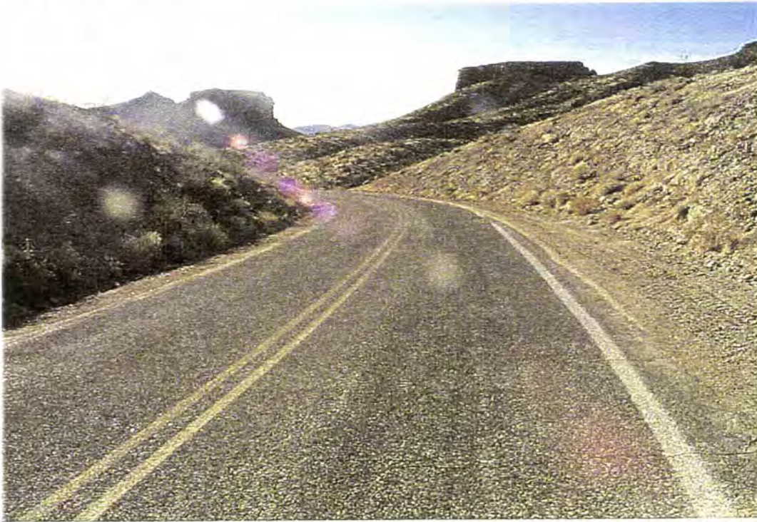
Photo #1667 - MP 0.00 - Begin of Route, Typical Pavement Section
