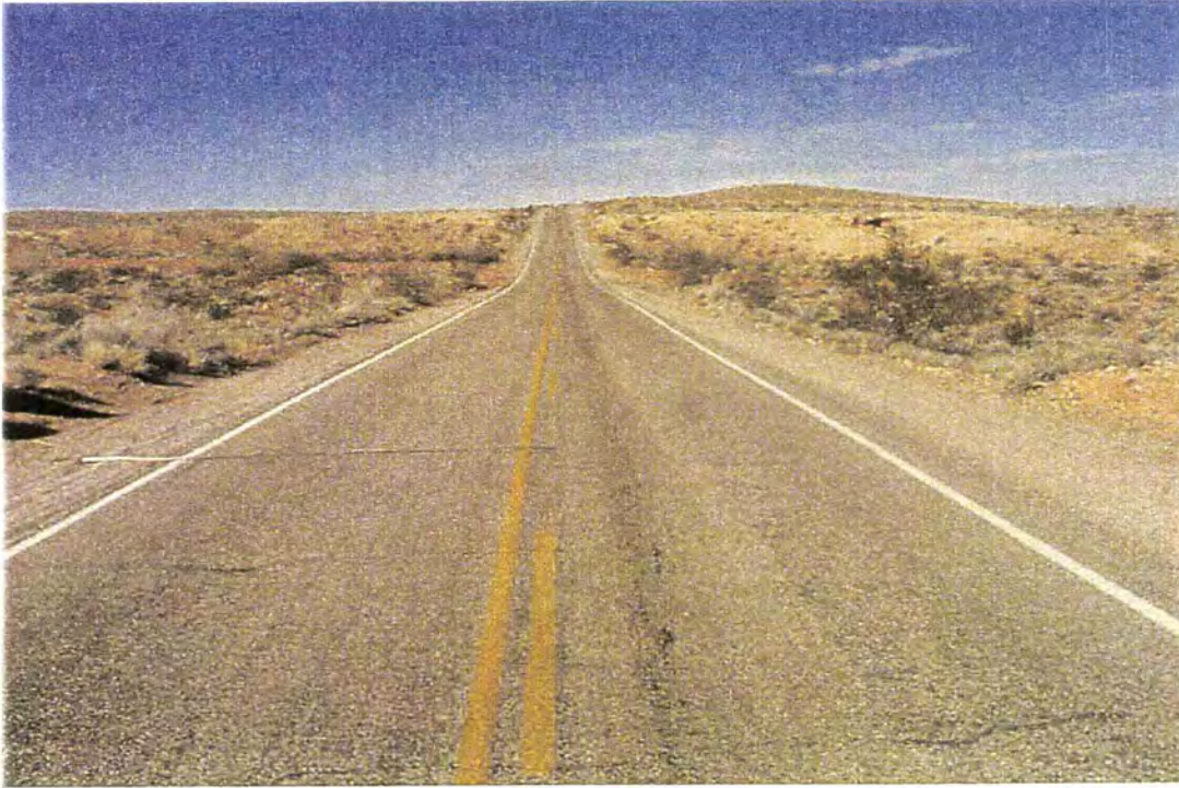
Photo #1627 - MP 46.20 - Typical Pavement Section
