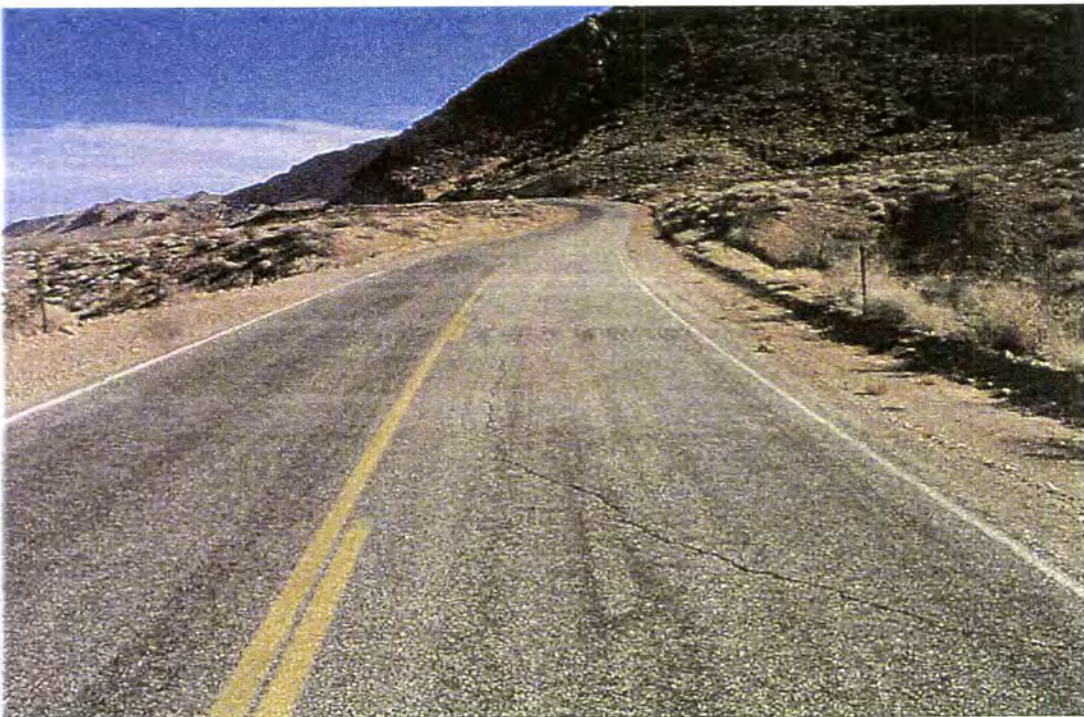
Photo #1623 - MP 21.40 - Parking Area Left (Rte 968)
