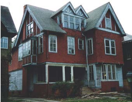
Before and After—The Michigan state tax credit helped to transform Detroit’s Kales House.
