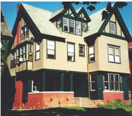
Kales House, Detroit, Courtesy State Historic Preservation Office
