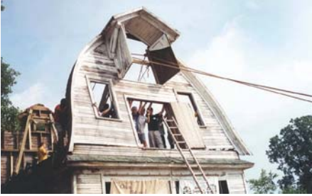
Porritt Barn, Orion Township, Oakland County Courtesy Lori Brown
