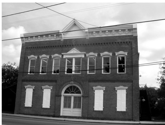
Figure 11-7. Percy Lobdell Building, Thibodaux. (author)
