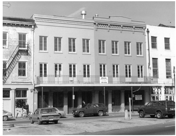
Figure 8-3. 419 Decatur façade, before restoration. (JELA)
