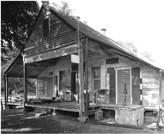
Figure 12-4. Oakland Plantation Store, Cane River. (HABS)
