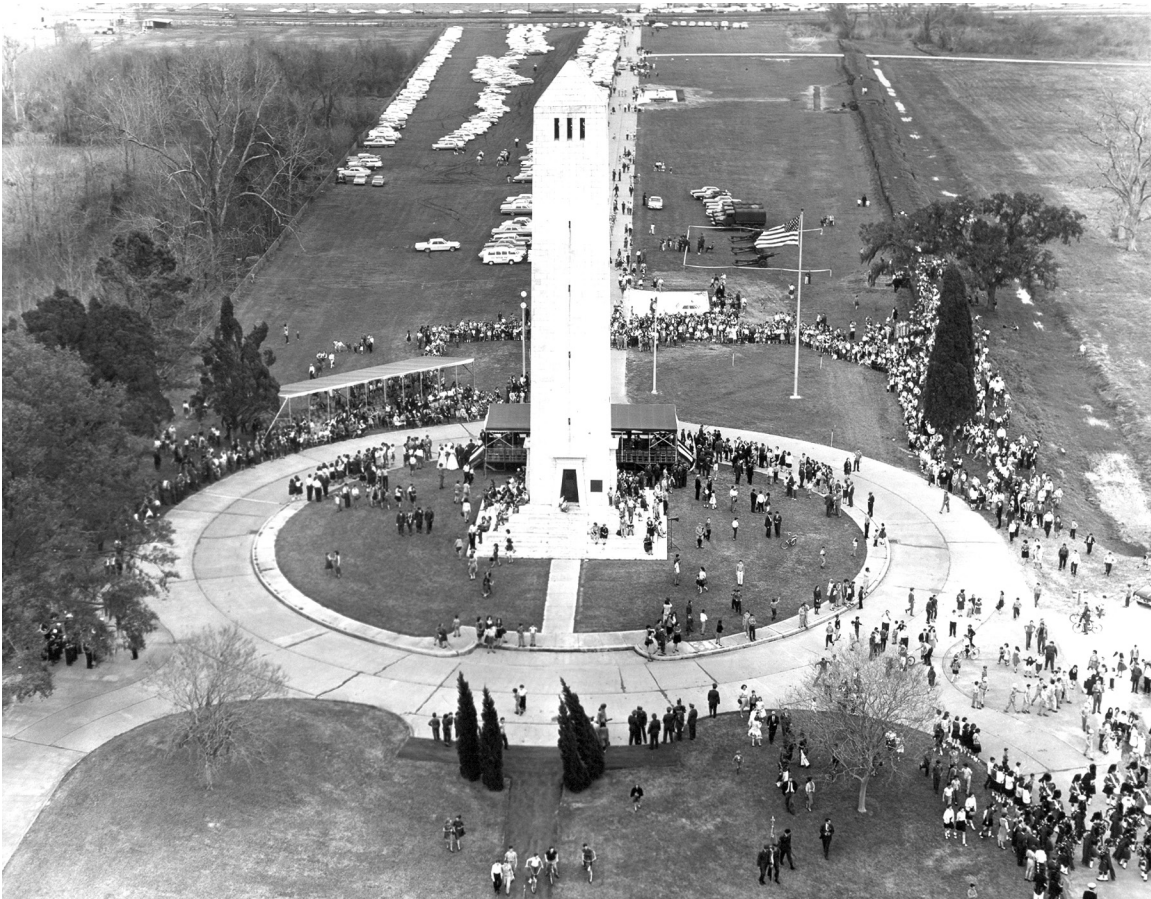
Figure 5-9. Aerial view of sesquicentennial activities, January 1965. (JELA)
