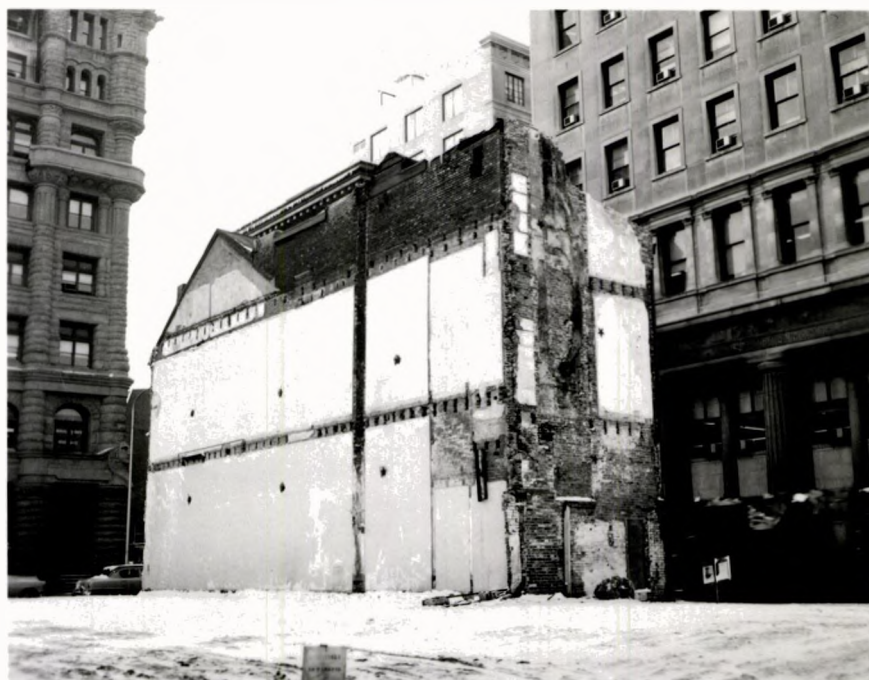
The Todd House, in 1957, after demolition of adjoining properties at Fourth and Walnut Streets. Note the 19th century addition, which completely obscures the original house yard, alleyway and back lot.
