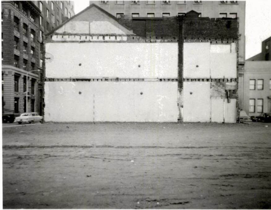
East elevation of the Todd House, after 1957 demolition of adjoining Griffitts and Morris houses. The misleading appearance of the structure is caused by the elongated 19th century addition. The original back lot, alleyway and yard are covered over by this post-1818 addition.
