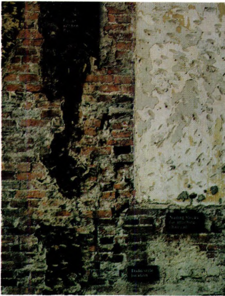
The original party walls at 322 Market were left exposed as an exhibit-in-place.
