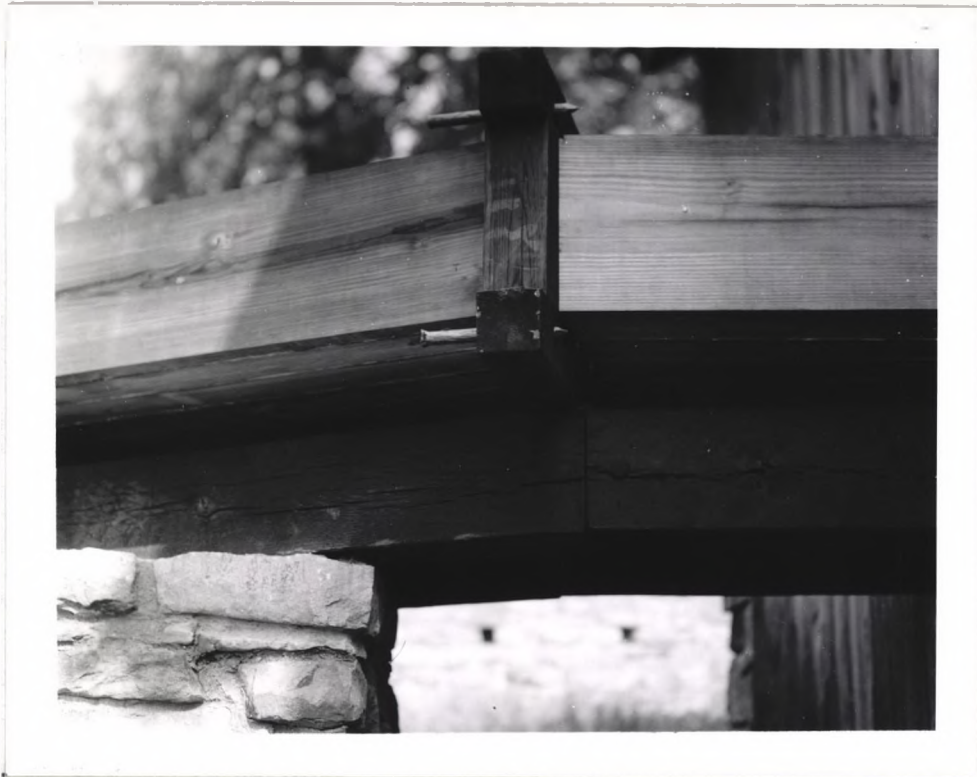
View of Forebay Pier #2 where flume enters wheelhouse on the right. Note that pegs have not been sawed off awaiting final curing of the oak timbers.
