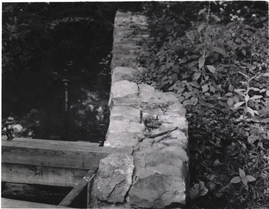
Resetting of Headrace Wall at the gate where water enters the West Headrace Flume.
