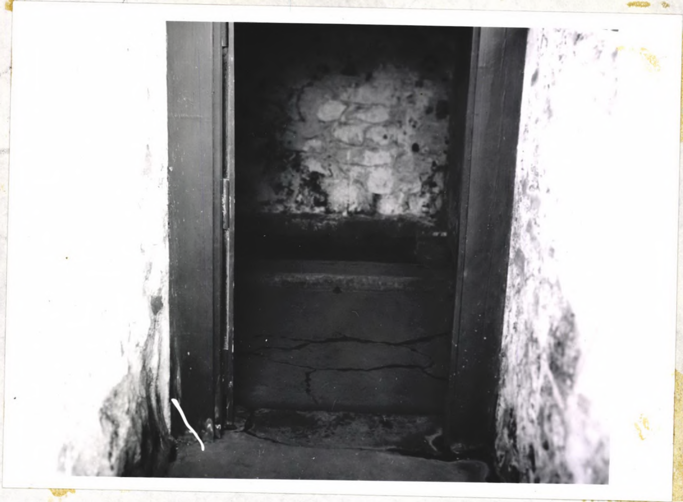
Concrete floor in Spring Section
