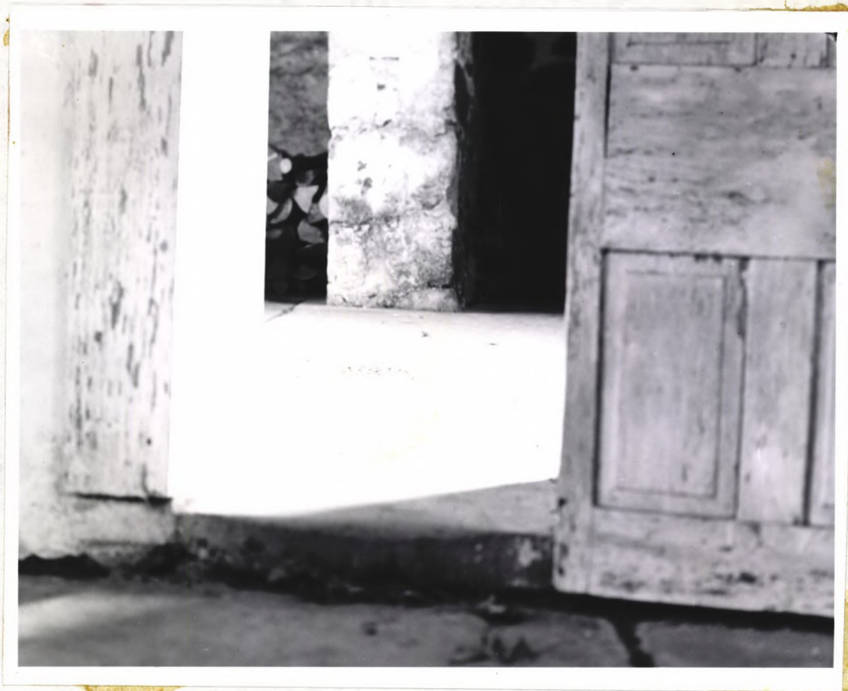
Concrete floor in Lard Kitchen
