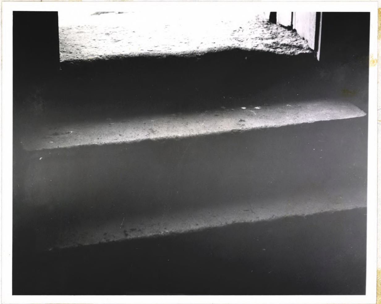
Modern concrete steps out of the Spring House
