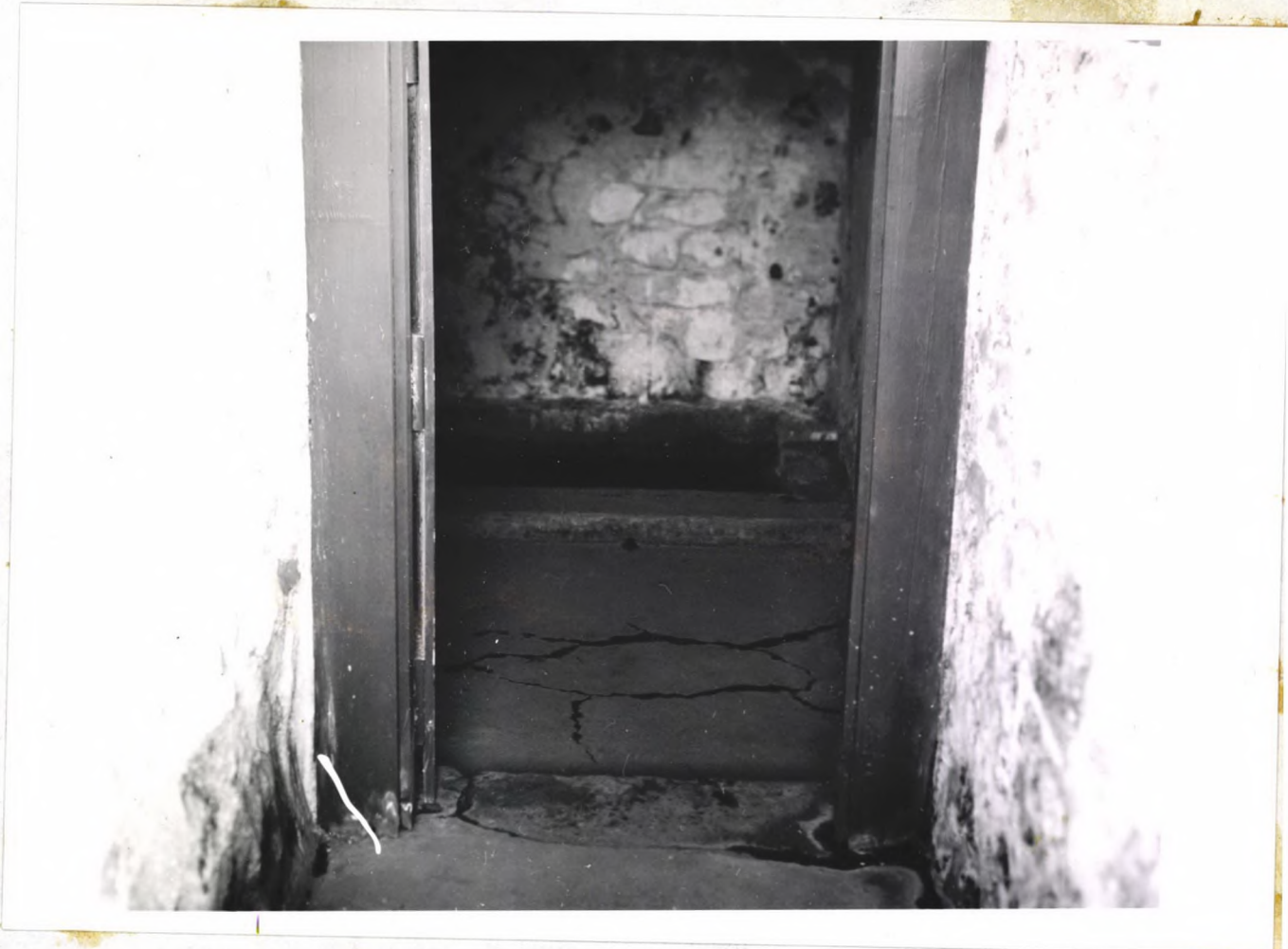
Concrete floor in Spring Section
