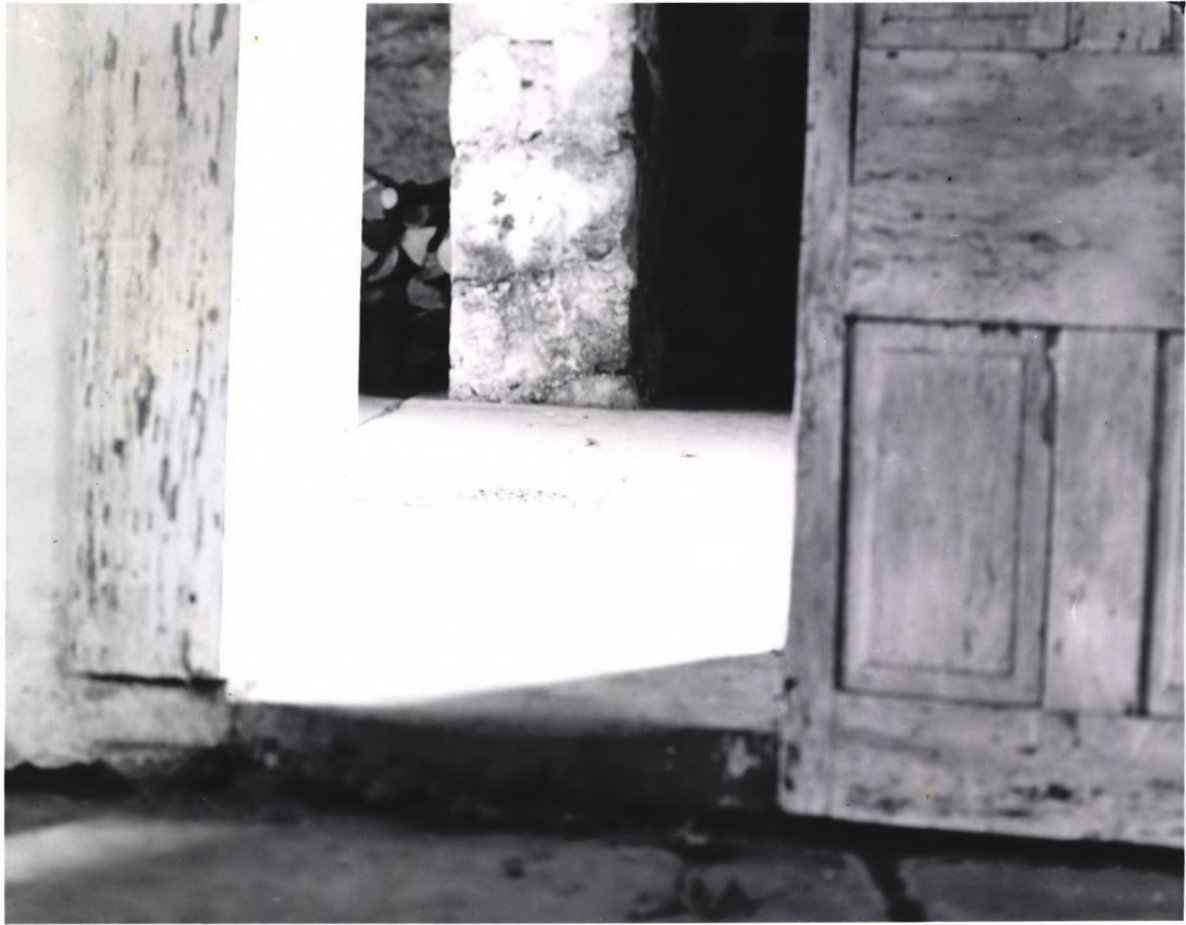
Concrete floor in Lari Kitchen
