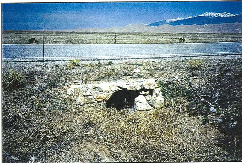
Photo # 03 - Typical culvert inlet with headwall (MP 0.85)
