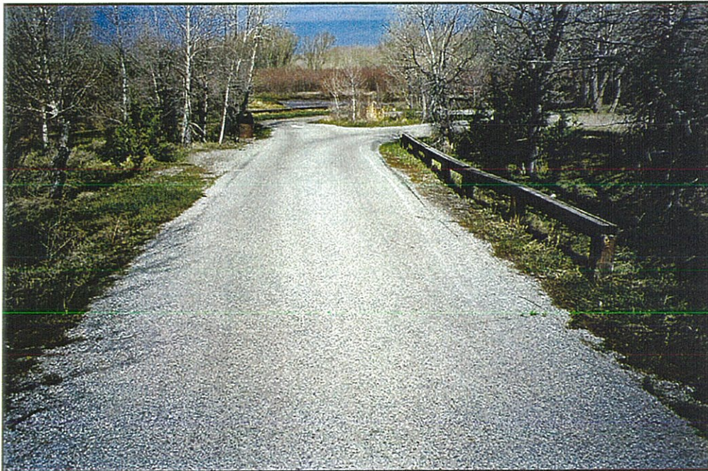
Photo # 18 - Wood guardrail
