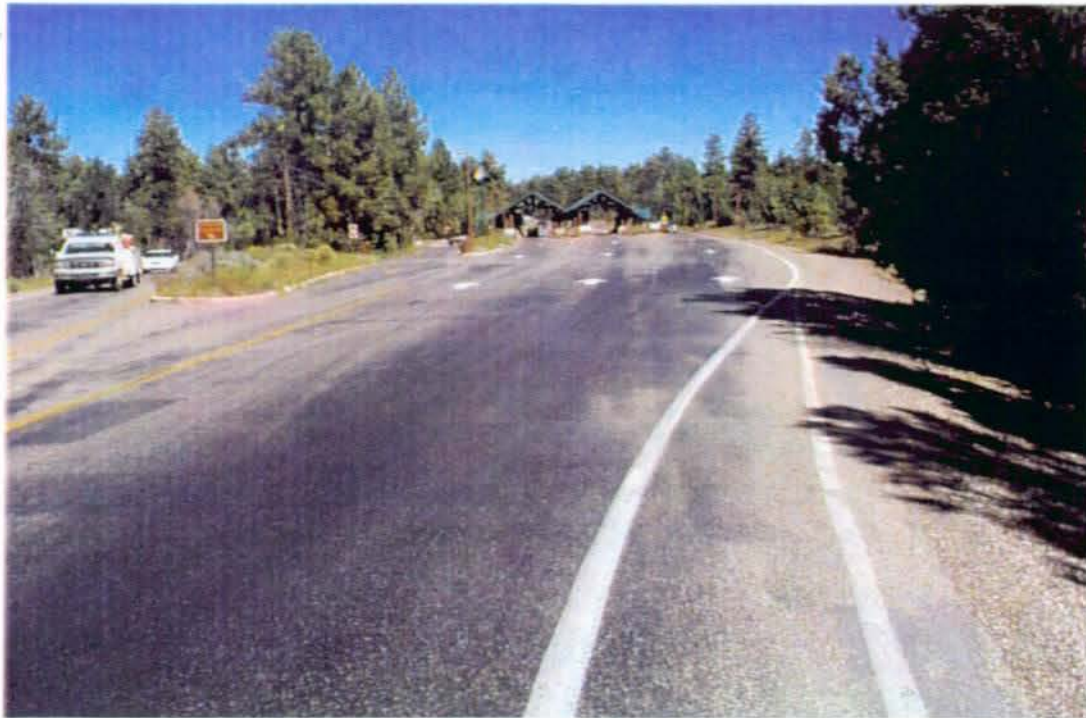
Photo #3680 - MP 0.44 - Begin widening for South Entrance Station.
