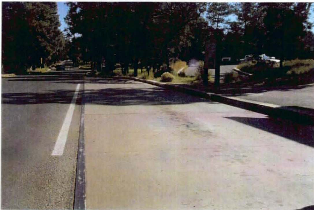
Photo #182 - Center Road Bus Stop.
