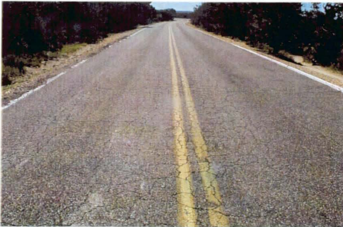
Photo #3685 - MP 3.40 - Typical Pavement Section.
