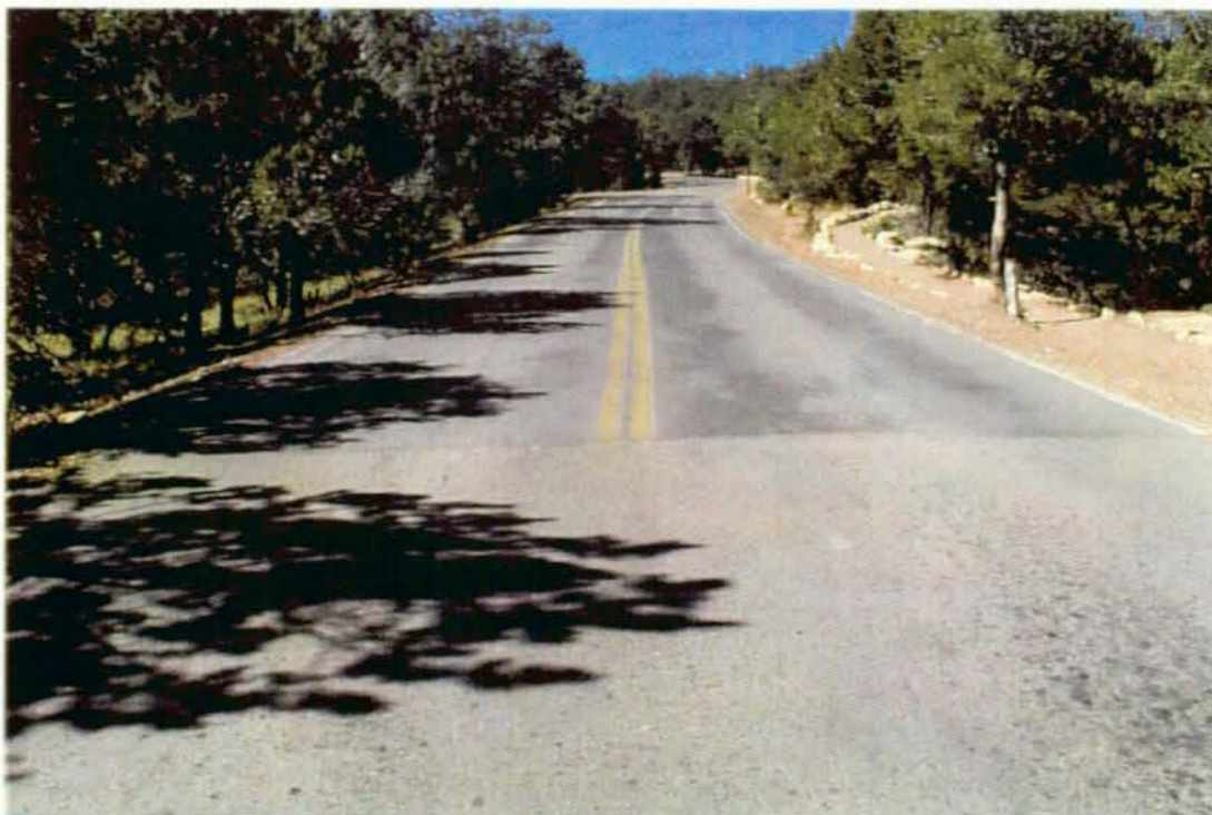
Photo #3683 - MP 0.03 - Typical Pavement Section.
