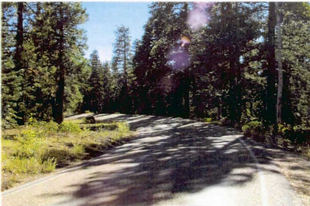
Photo #47 - MP 6.81 - Typical Pavement Section.
