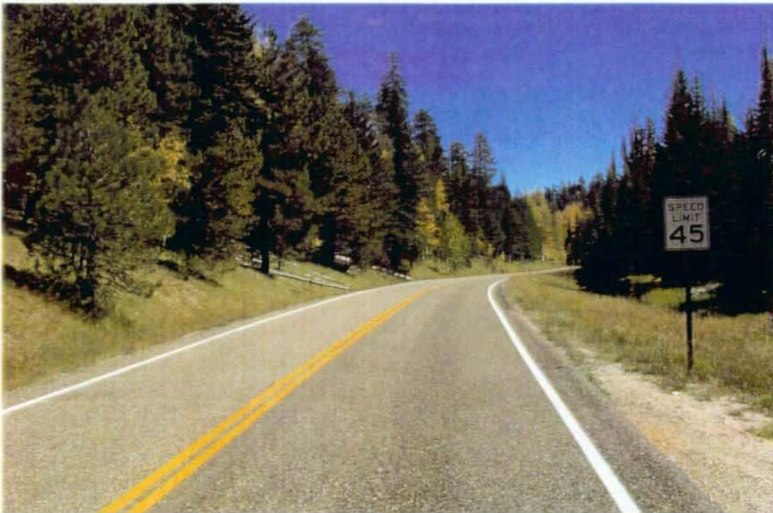
Photo #38 - MP 5.35 - Typical Pavement Section.
