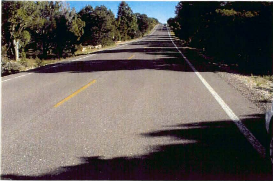
Photo #3710 - MP 13.40 - Typical Pavement Section.
