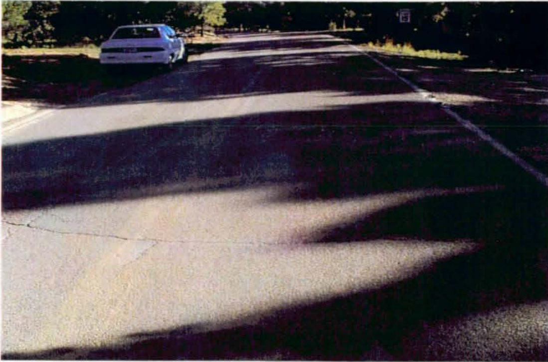
Photo #3695 - MP 0.00 - Begin at Route 409, Typical Pavement Section.
