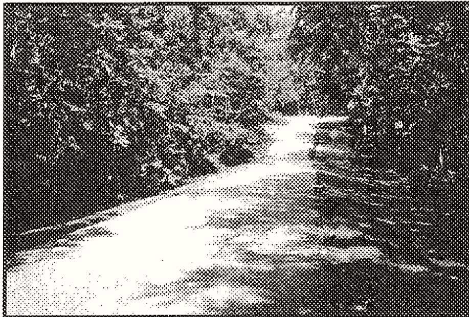
Photo # 43 - MP 0.10 Typical pavement section
