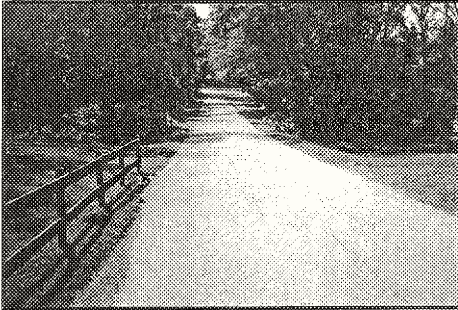
Photo # 06 - MP 0.01 Typical pavement section
