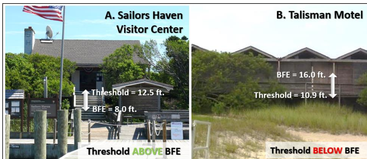
Figure 3. Two FII structures that had revised scores for the flood damage potential (elevated) sensitivity indicator based on the precise threshold elevation data (collected by NPS-RISD) and BFE values. A) Sailors Haven Visitor Center was originally reported as not elevated within the questionnaire, but the threshold elevation data showed that the first floor was, in fact, above BFE. Therefore, this structure was modified to receive a favorable score for the flood damage potential sensitivity indicator. B) Talisman Motel was originally reported as elevated within the questionnaire, but the threshold elevation data showed that the first floor was, in fact, below BFE. Therefore, this structure was modified to receive an unfavorable score for the flood damage potential sensitivity indicator. Threshold elevation and BFE values are relative to the North American Vertical Datum of 1988 (NAVD88).
