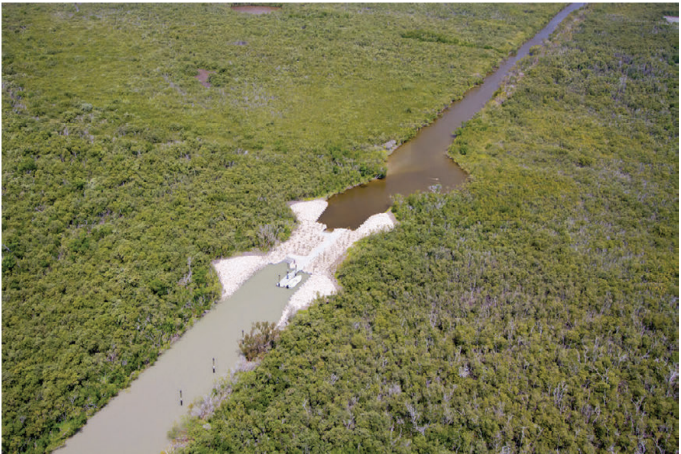
Figure 33. Example of a canal plug.
