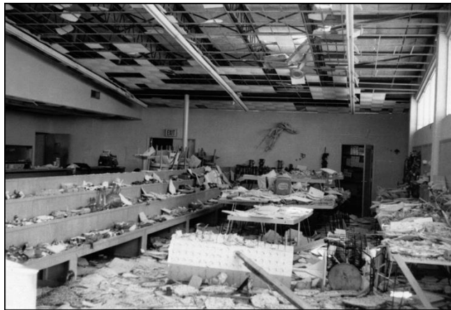
Figure 16–1, damage to concessioner’s shop at Flamingo from Hurricane Donna, 1960
