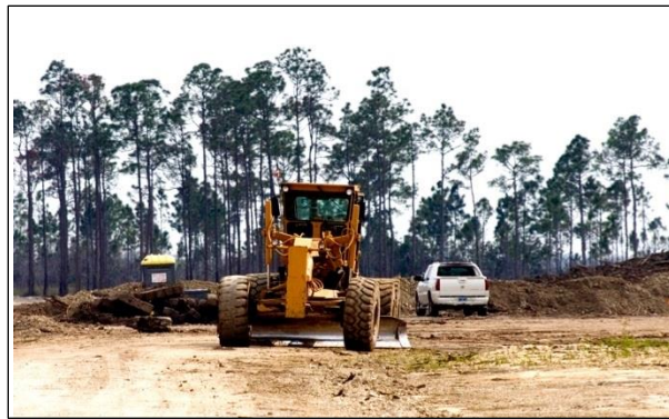
Figure 14–6, removing soil in the Hole-in-the Donut).
