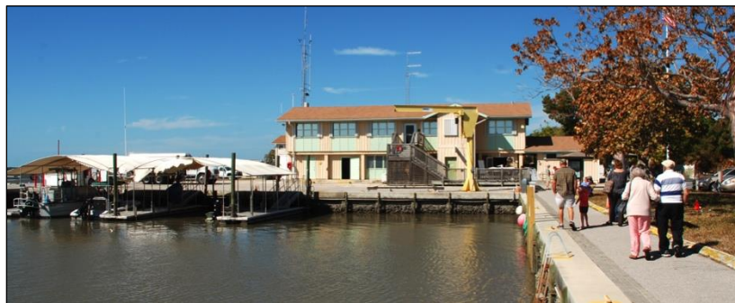
Figure 7–22, Everglades City ranger station and boat basin
