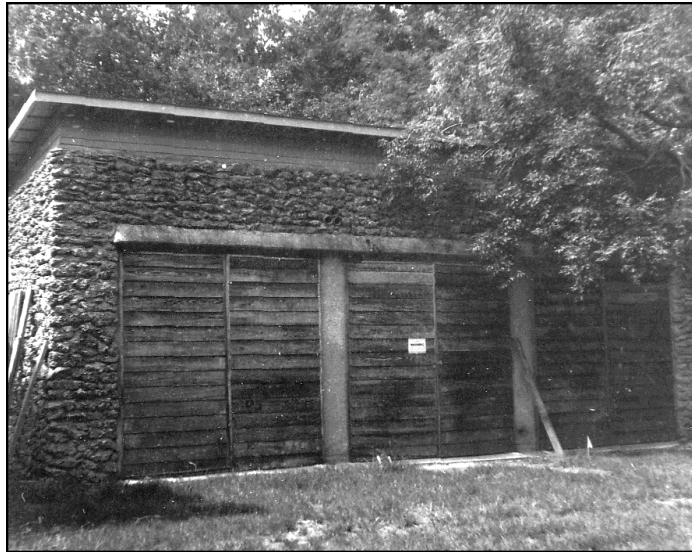
Figure 17-7, CCC-built garage at Royal Palm
