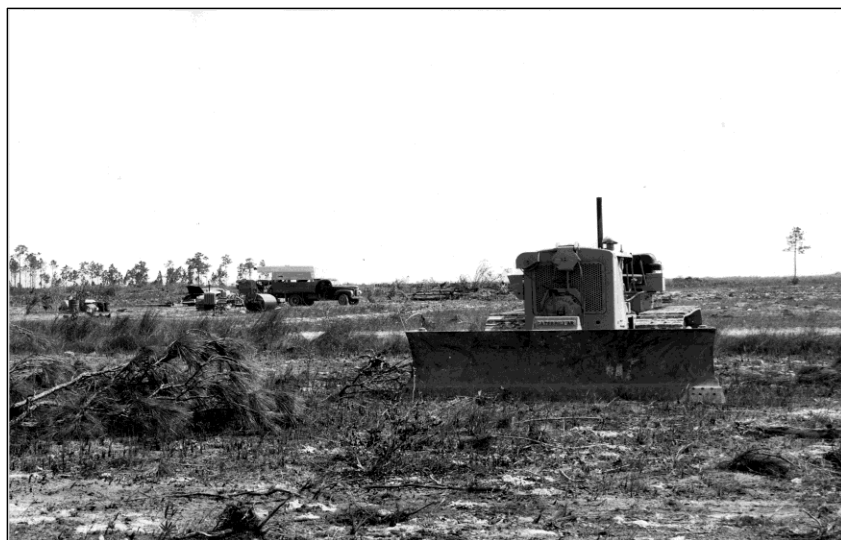
Figure 6–5, bulldozer with scarifying blade for rock plowing, 1955
