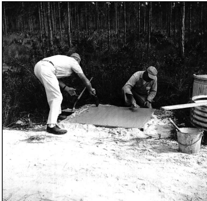
Figure 7-20, laying a concrete pad at Long Pine campground
