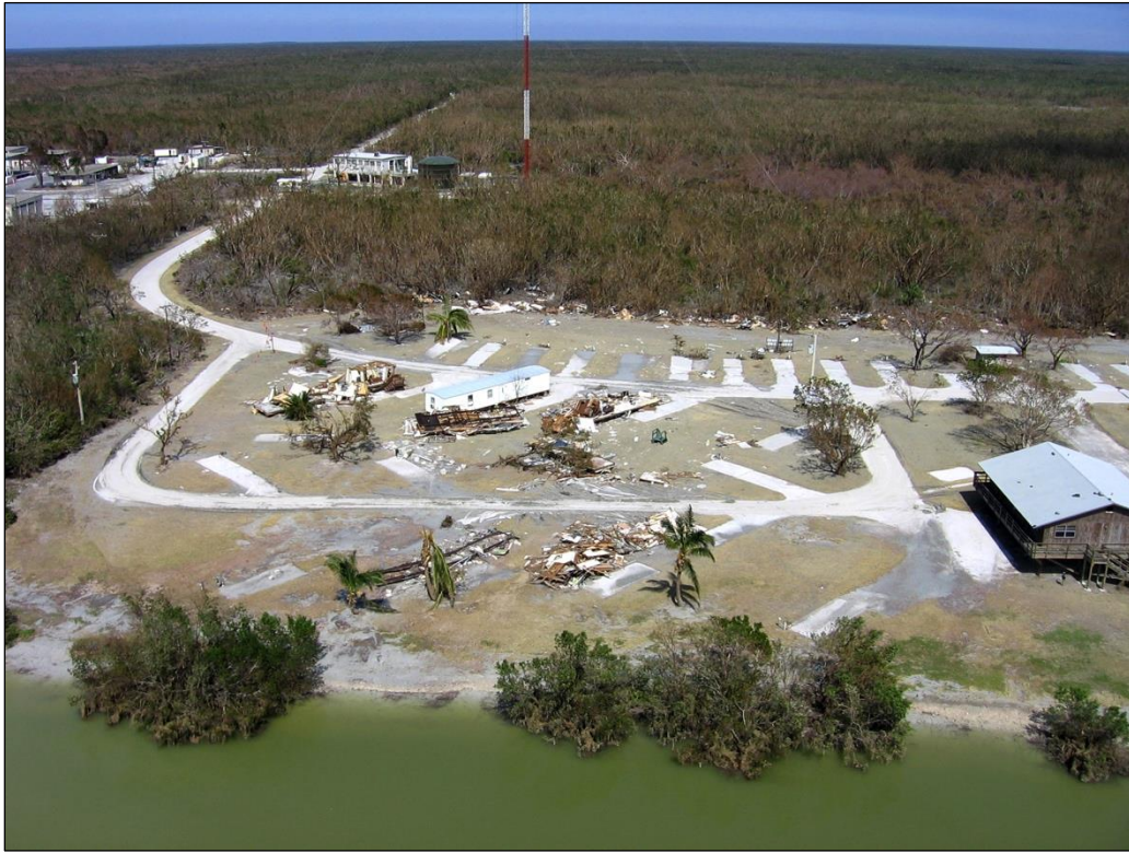
Figure 16-4, Flamingo housing area following Hurricane Wilma, 2005
