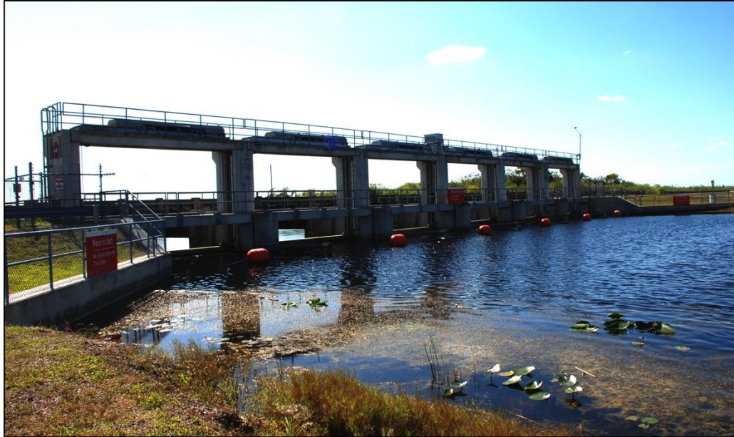
Figure 8–3, one of the S-12 water control gates
