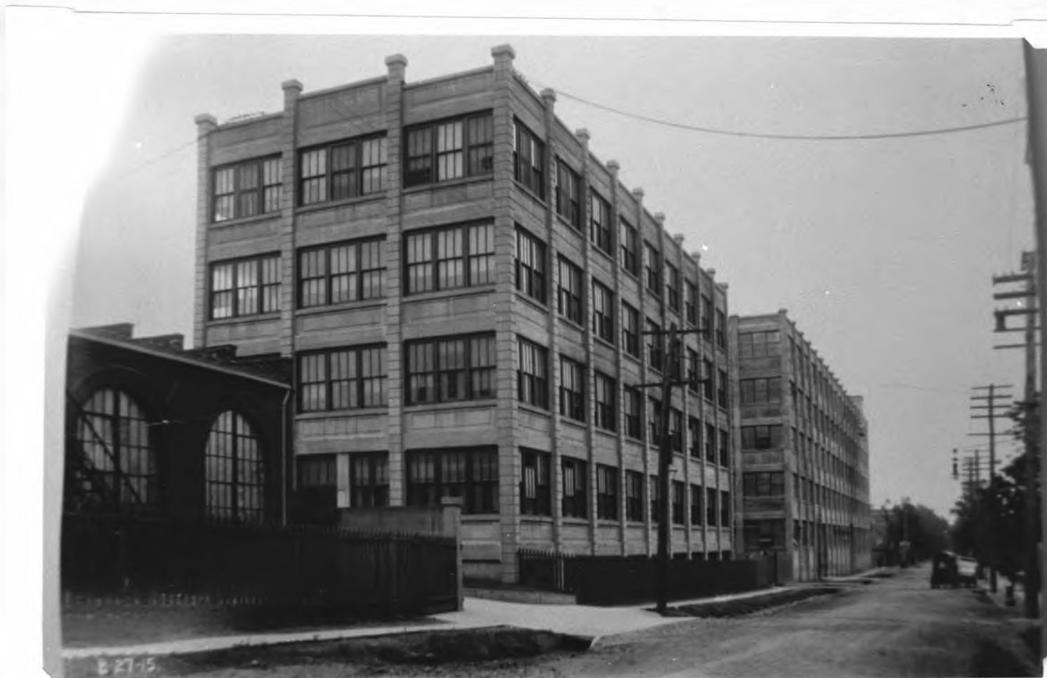
Illustration 8-2 The Administrative Building
