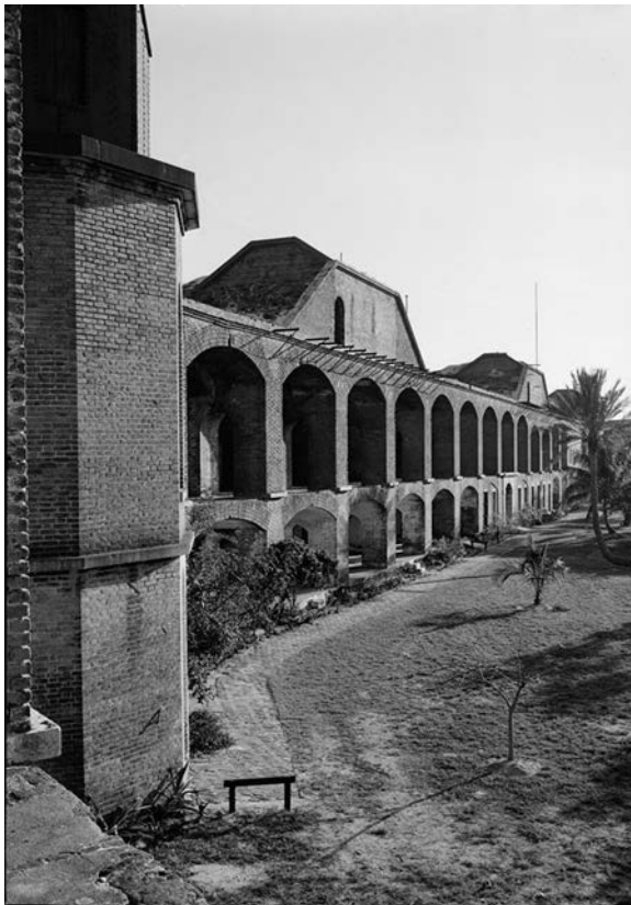
Figure 178. Image of walkway from Bastion 1 to 6, 1962. (HABS 053134)
