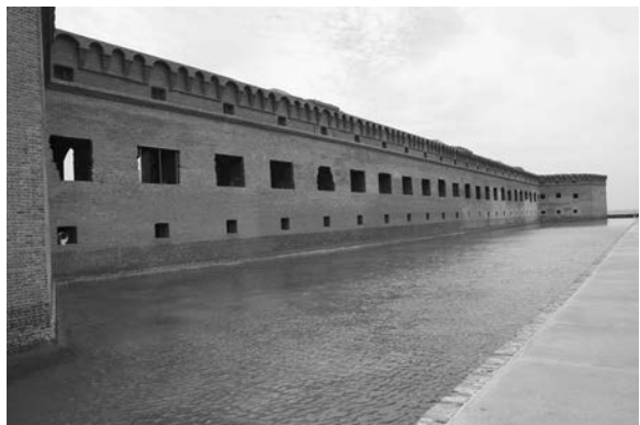
Figure 26. Front 4 wall repair, June 2009. (SERO image)
