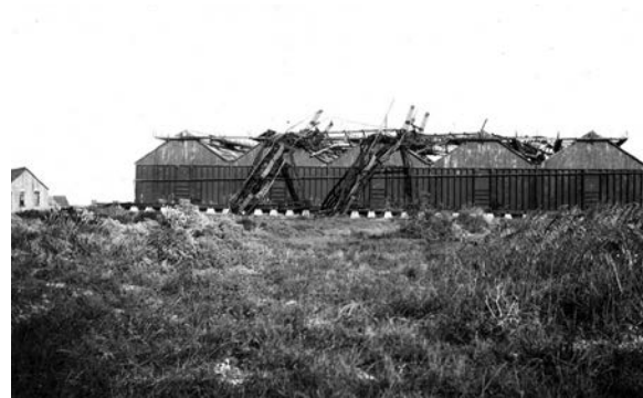
Figure 54. Damage to south coal shed, 1911. (USGS Photographic Library vtw00352)
