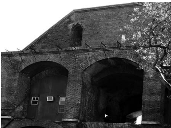
Figure 221. Walkway braces, 2010. (SERO image 1533)
