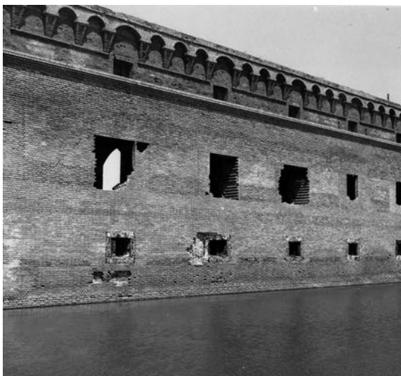
Figure 93. Loss of face brick due to iron exfoliation, 1970. (Alexander Physical Status Report 27)
