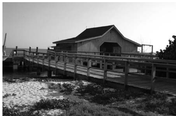
Figure 206. Main dock, 2010. (SERO image 1501)
