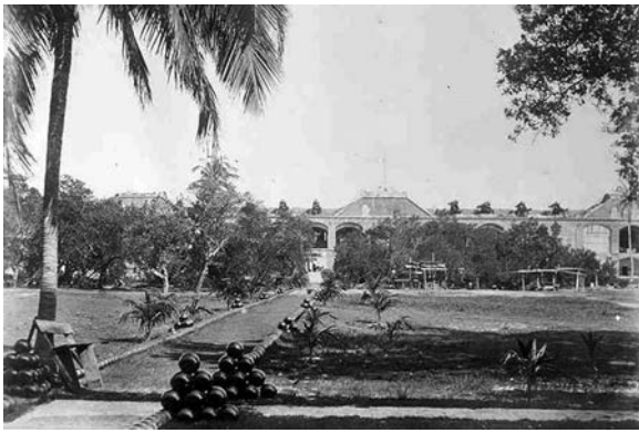
Figure 69. View looking to sally port from officers' quarters, 1898. (EVER 7342)
