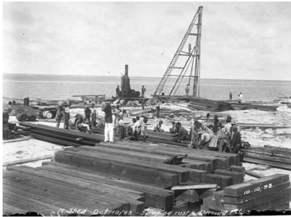
Figure 51. Construction of north coal depot, 1898. (John Meigs Photograph Collection, Dry Tortugas National Park, DRTO 3805)
