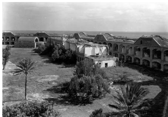
Figure 78. Enlisted men's quarters and Major Smith monument, 1937. (EVER 7123)
