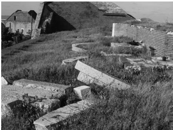
Figure 262. Disrupted granite pieces, Front 4, 2010. (SERO image 1544)
