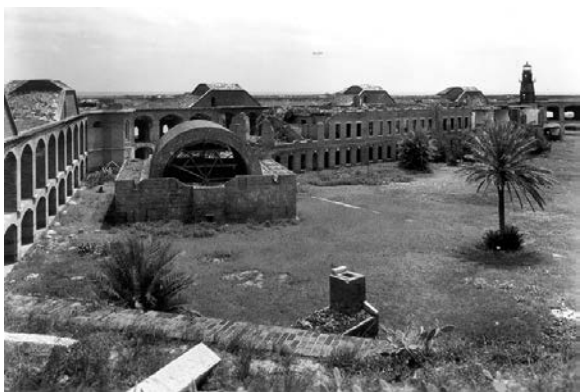
Figure 138. Large powder magazine, 1937. (EVER 7122) repointing and sealing to prevent the mortar from leaching out. 84
