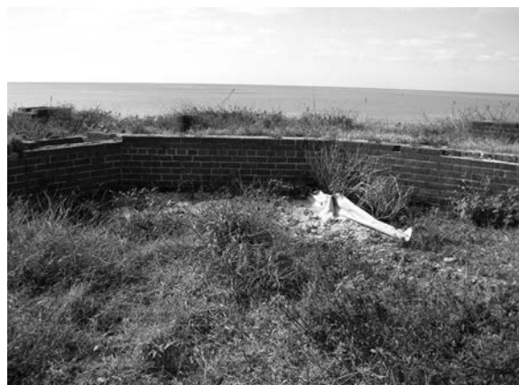
Figure 223. Waterproofing membrane, 2010. (SERO image 1640)
