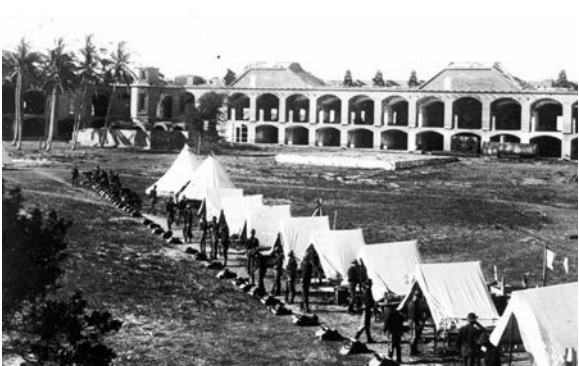
Figure 132. Chapel/office cistern, 1898. (EVER 7345)
