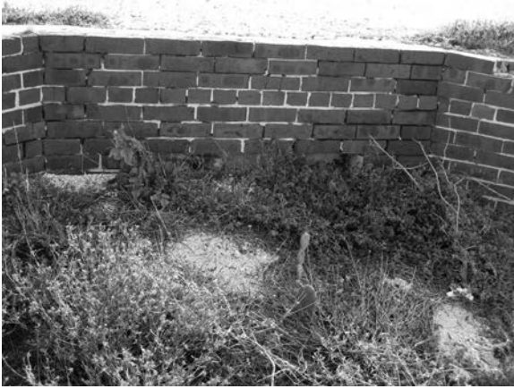
Figure 283. Shot cellar covered with sand and vegetation, 2010. (SERO image 1562)
