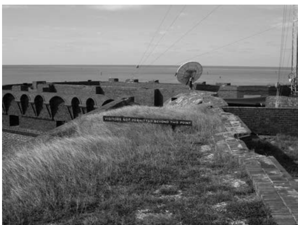
Figure 247. Communications equipment at Bastion 1, 2010. (SERO image 1629)
