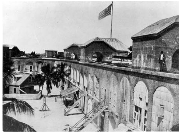
Figure 41. Original lightkeeper's quarters, 1867. (National Archives 77-F-74-79D)
