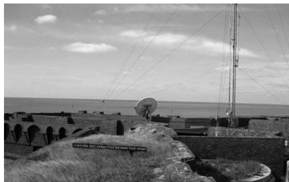
Figure 281. Communications equipment, 2010. (SERO image 1628)
