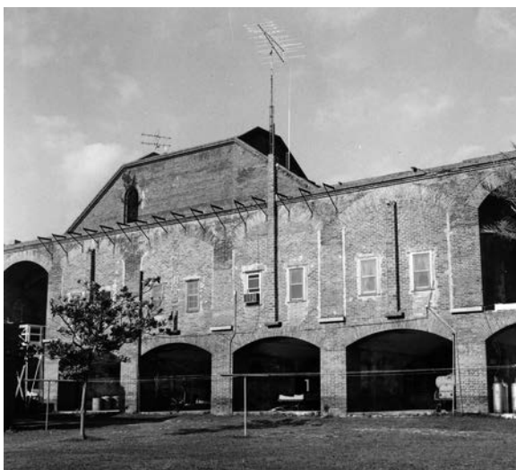
Figure 92. Quarters #3 in upper tier casemates Front 3, maintenance units in bottom, 1970. (Alexander Physical Status Report 80)
