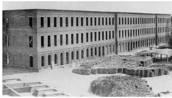
Figure 120. Enlisted men's quarters under construction, 1864. (DRTO 300894)
