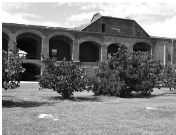
Figure 254. Vegetative screen in front of maintenance units, 2010. (SERO image 1534)
