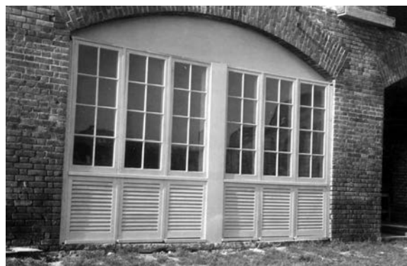
Figure 90. Casemate enclosure, 1945. (DRTO 300906)
