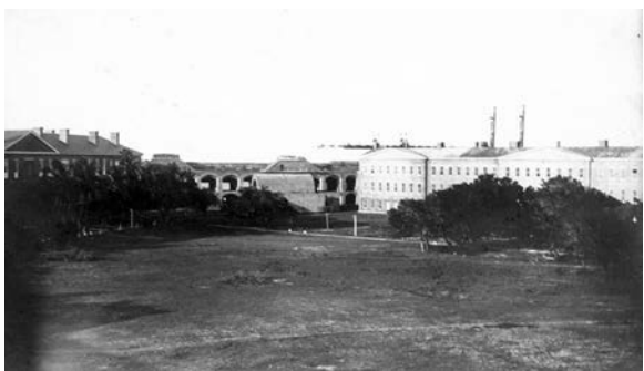
Figure 10. Officers' quarters, large magazine, and enlisted men's quarters, 1909. (Monroe County Library)
