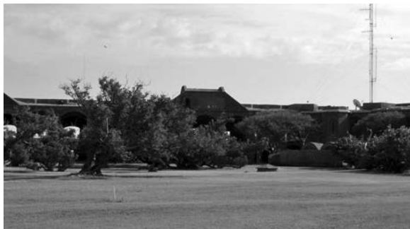
Figure 251. Views up to the terreplein of radio tower, 2010. (SERO image 1487)
