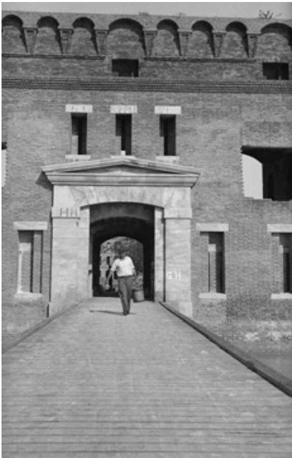
Figure 112. Sally port, 1934. (HABS 053108)
