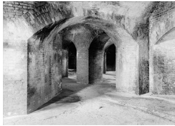
Figure 88. Typical arch construction, 1934. (HABS 053147)
