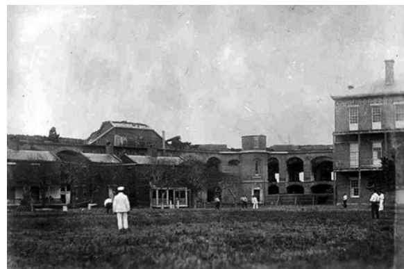
Figure 89. Stair tower with turret, wooden galleries, and cannon, 1901. (DRTO 301203)
