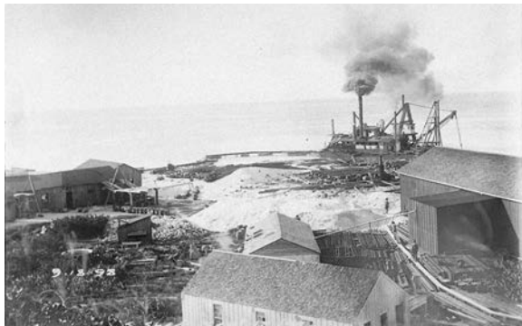
Figure 52. Construction of south coal depot, 1898. (John Meigs Photograph Collection, Dry Tortugas National Park, DRTO 3805)
