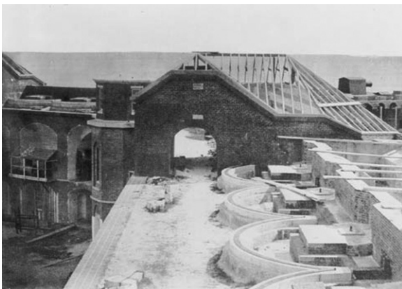
Figure 9. Terreplein under construction, 1863. (DRTO 300646)
