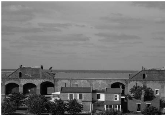
Figure 252. Views of asphalt roof and satellite dish, 2010. (SERO image 1572)
