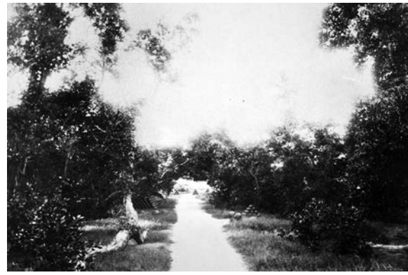
Figure 175. Secondary parade walkway, c. 1898. (John Meigs Photograph Collection, Dry Tortugas National Park, DRTO 3805)
