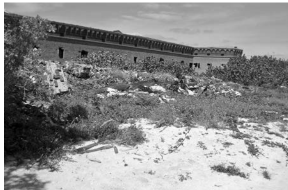
Figure 205. Brick and rubble debris pile, 2010. (SERO image 1658)
