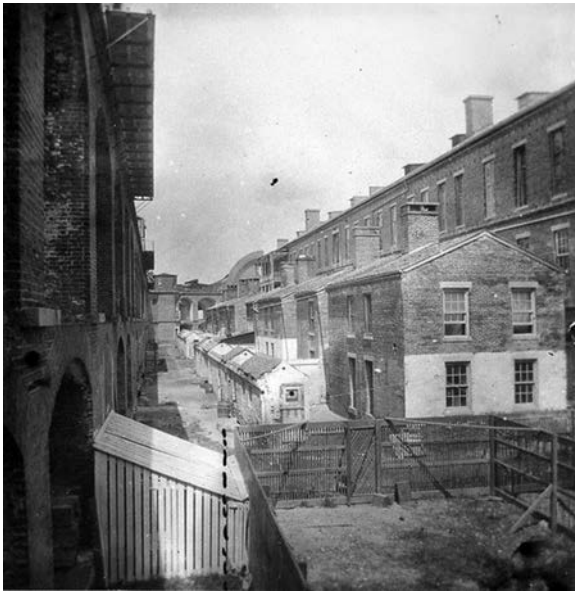
Figure 184. Paling fencing in the work yard of the officers' quarters, c. 1870s.
