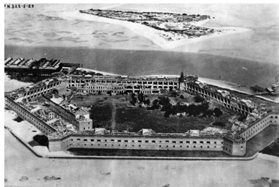
Figure 275. Aerial image of Fort Jefferson, c. 1929. (National Archives RG90)
