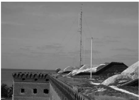
Figure 263. Telecommunications equipment along Front 1, 2010. (SERO image 1606)
