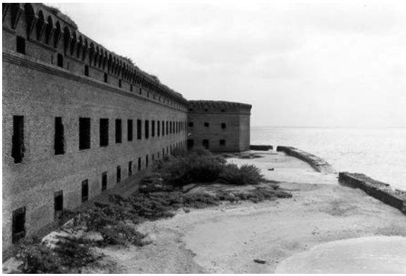
Figure 103. Moat filled with sand, Front 4, 1937. (EVER 7175)
