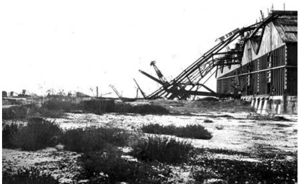
Figure 163. North depot hurricane damage, 1911. (USGS Photographic Library vtww00357)
