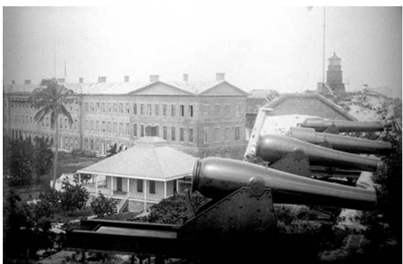
Figure 158. New keeper's quarters, 1898. (John Meigs Photograph Collection, Dry Tortugas National Park, DRT0 3805)
