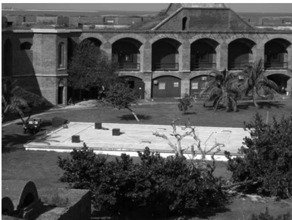
Figure 231. Cistern, 2010. (SERO image 1622)
