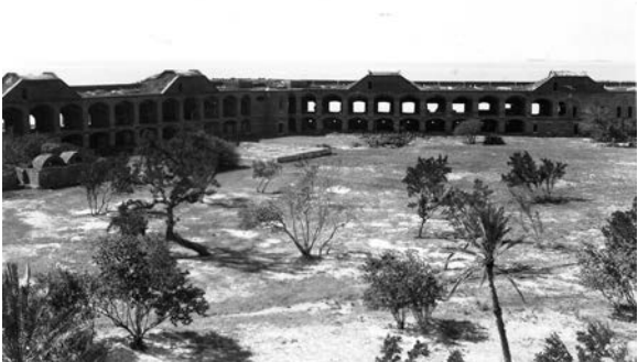
Figure 134. Chapel/office cistern, 1937. (DRTO 301080)
