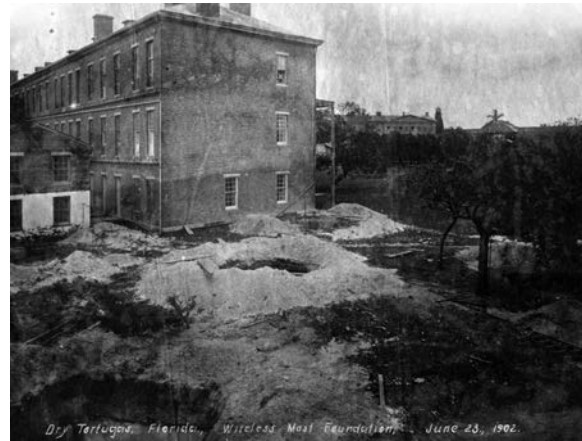
Figure 17. Wireless mast foundation, 1902. (Monroe County Library)
