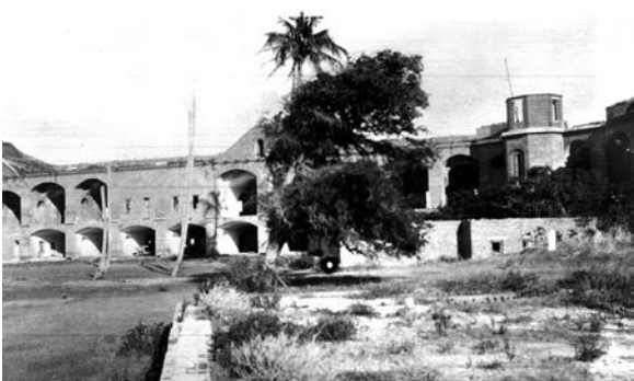
Figure 133. Chapel/office cistern, 1913. (USGS Photographic Library sew01385)
