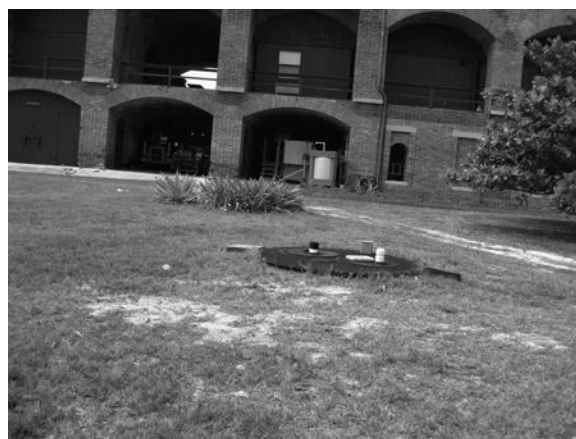
Figure 224. Maintenance area with modular housing units above, 2010. (SERO image 1537)
