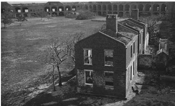
Figure 127. Engineer officers' quarters, 1934. (HABS 053117)
