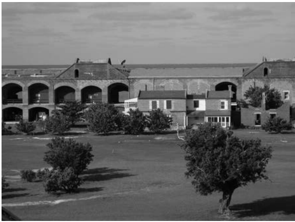
Figure 230. Engineer officers' quarters, 2010. (SERO image 1571)
