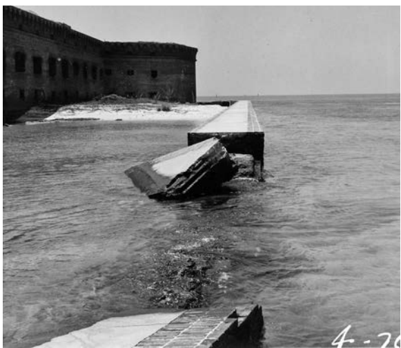
Figure 106. Close-up of section washed out by Hurricane Betsy, 1970. (Alexander Physical Status Report 9)
