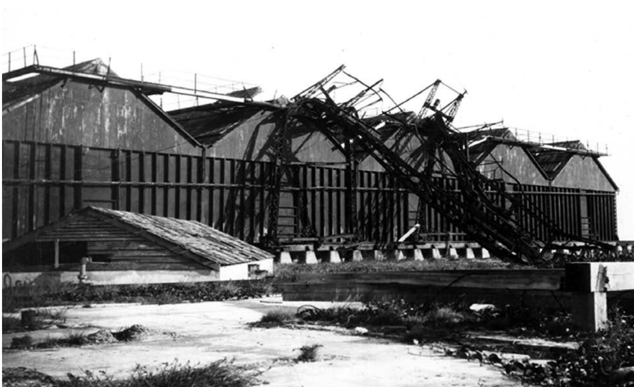
Figure 18. Damage to south coal depot, 1911. (USGS Photographic Library vtw00353)
