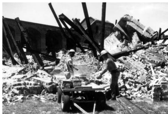
Figure 23. Enlisted men's quarters during demolition, 1962. (DRTO 300792)
