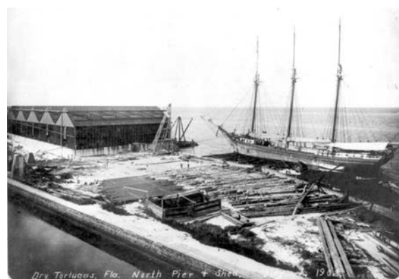
Figure 161. North depot, 1902. (National Archives)
