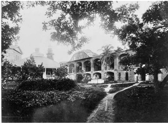
Figure 44. 1876 iron light tower and complex, 1898. (EVER 7349)
