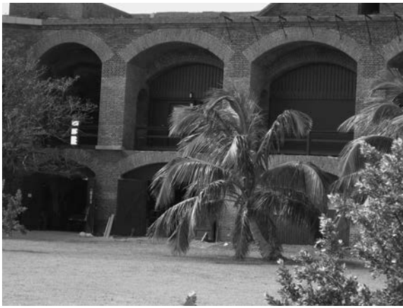
Figure 198. Casemates below used for maintenance, above used for housing, 2010. (SERO image 1535)
