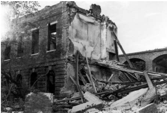
Figure 40. Enlisted men's quarters demolition, 1962. (DRTO 300673)
