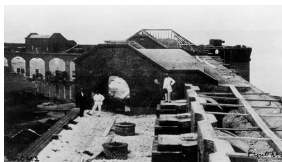
Figure 98. Water collection system on the terreplein, 1863. (DRTO 300685)
