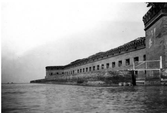
Figure 170. Front 4 showing sluice gate, 1910. (USGS Photographic Library vtw00323)
