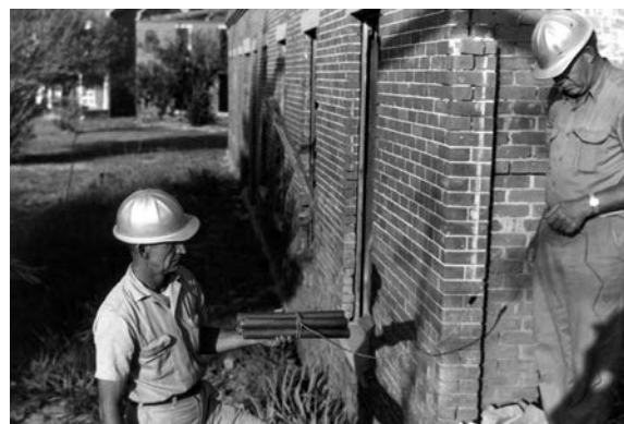
Figure 119. Demolition of officers' quarters, 1962. (DRTO 300765)
