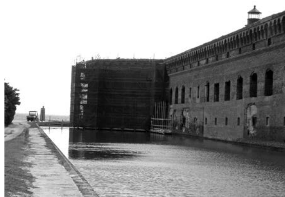
Figure 216. Phase II stabilization, 2010. (SERO image 1514)
