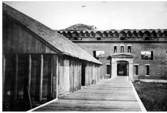
Figure 146. Frame building on wharf, 1908. (USGS Photographic Library vtw00292)
