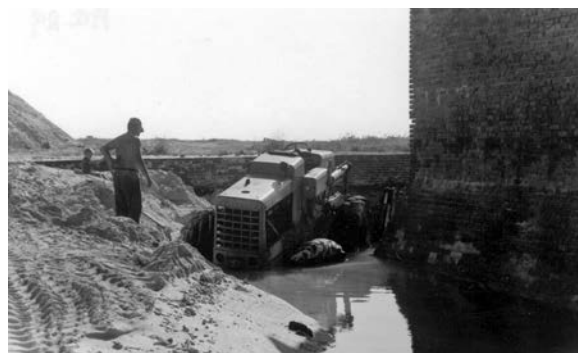
Figure 172. Moat dredging, 1965. (DRTO 300923)
