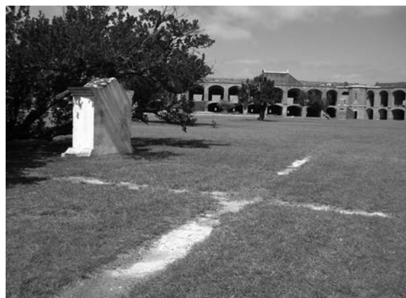
Figure 235. Major Smith Monument with concrete coping, 2010. (SERO image 1527)
