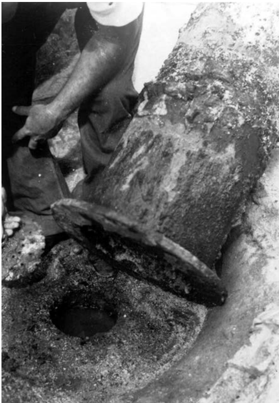
Figure 99. Cistern pipe, Bastion 1, 1938. (DRTO 300954)
