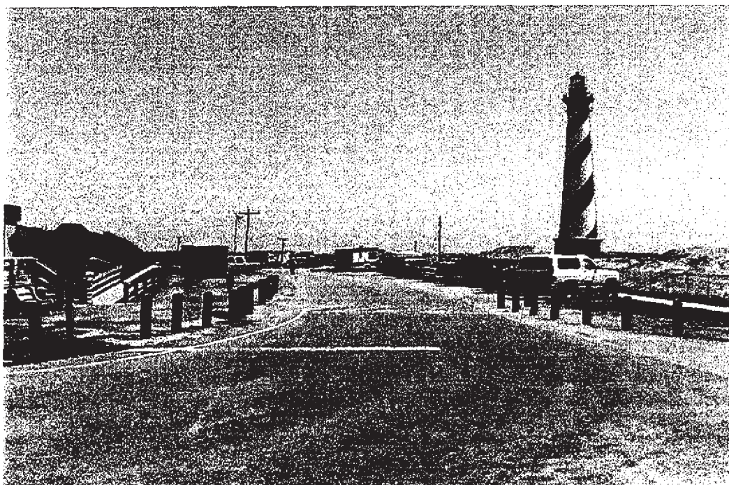
Photo #3 - MP 0.83 - Intersection with Rte 916 on right.
