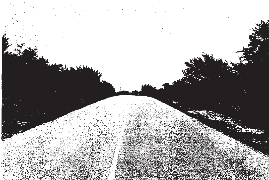
Photo #6 - MP 0.00 - Beginning of route—typical pavement section.
