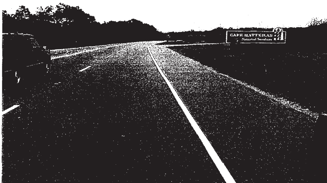
Photo #2909 - MP 0.00 Whalebone intersection—begin with four lanes
