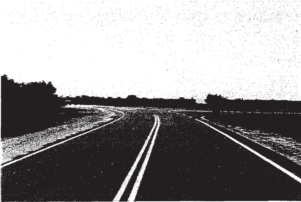
Photo #4 - MP 2.36 - Intersection with Rte 225 on right.
