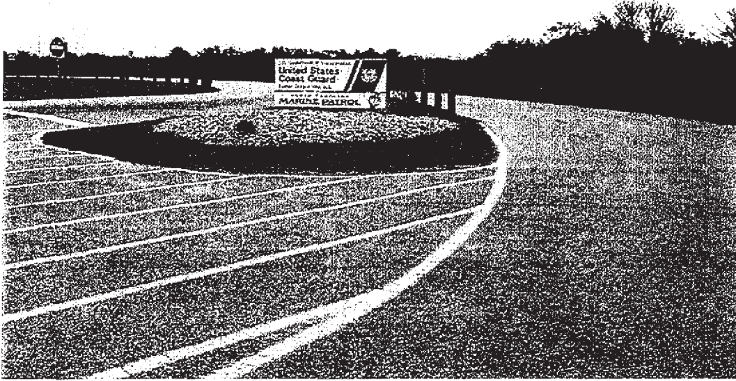
Photo #2919 - MP 0.00 - Begin route to USCS Station—typical pavement section
