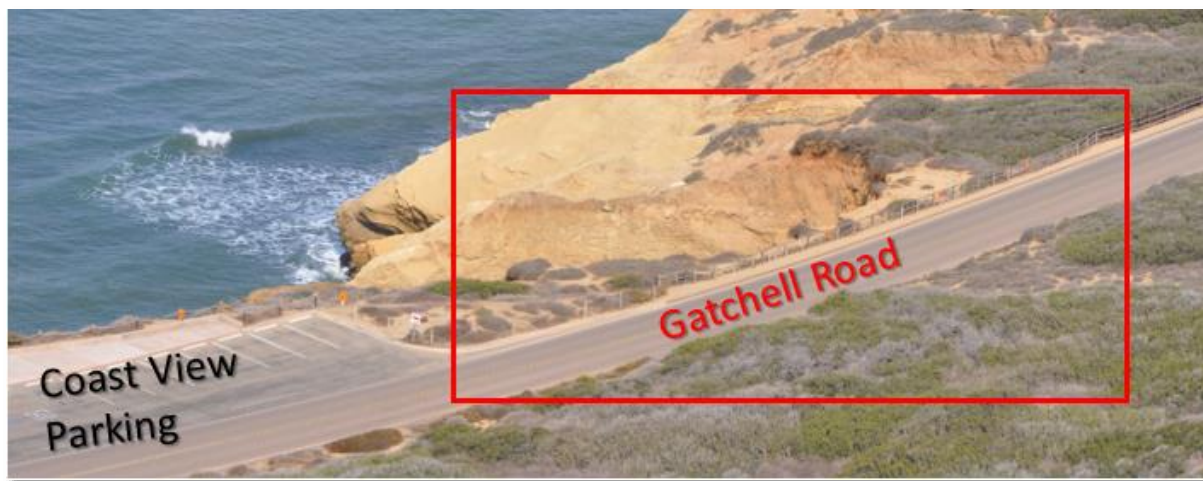
Figure 2. Cliff retreat adjacent to Gatchell Road. Notice the cliff edge roughly 6 feet from the road (red box).
