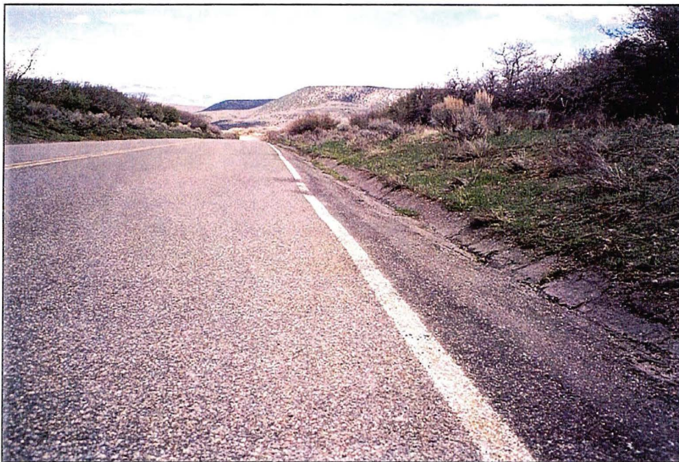
Photo # 02 - Section 1, Pavement buckling (MP 0.49)
