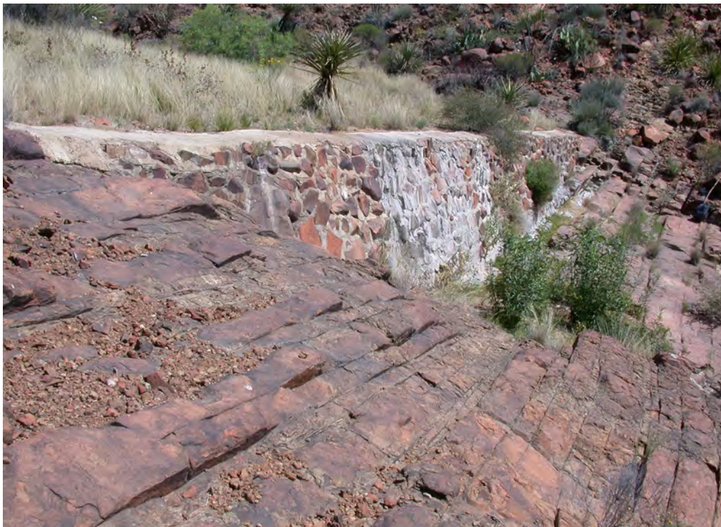
Figure 6-III.29 Portland cement-mortared stone dam at BIBE1642 (41BS1575) in the McKinney Hills. Photo by D. Keller.
