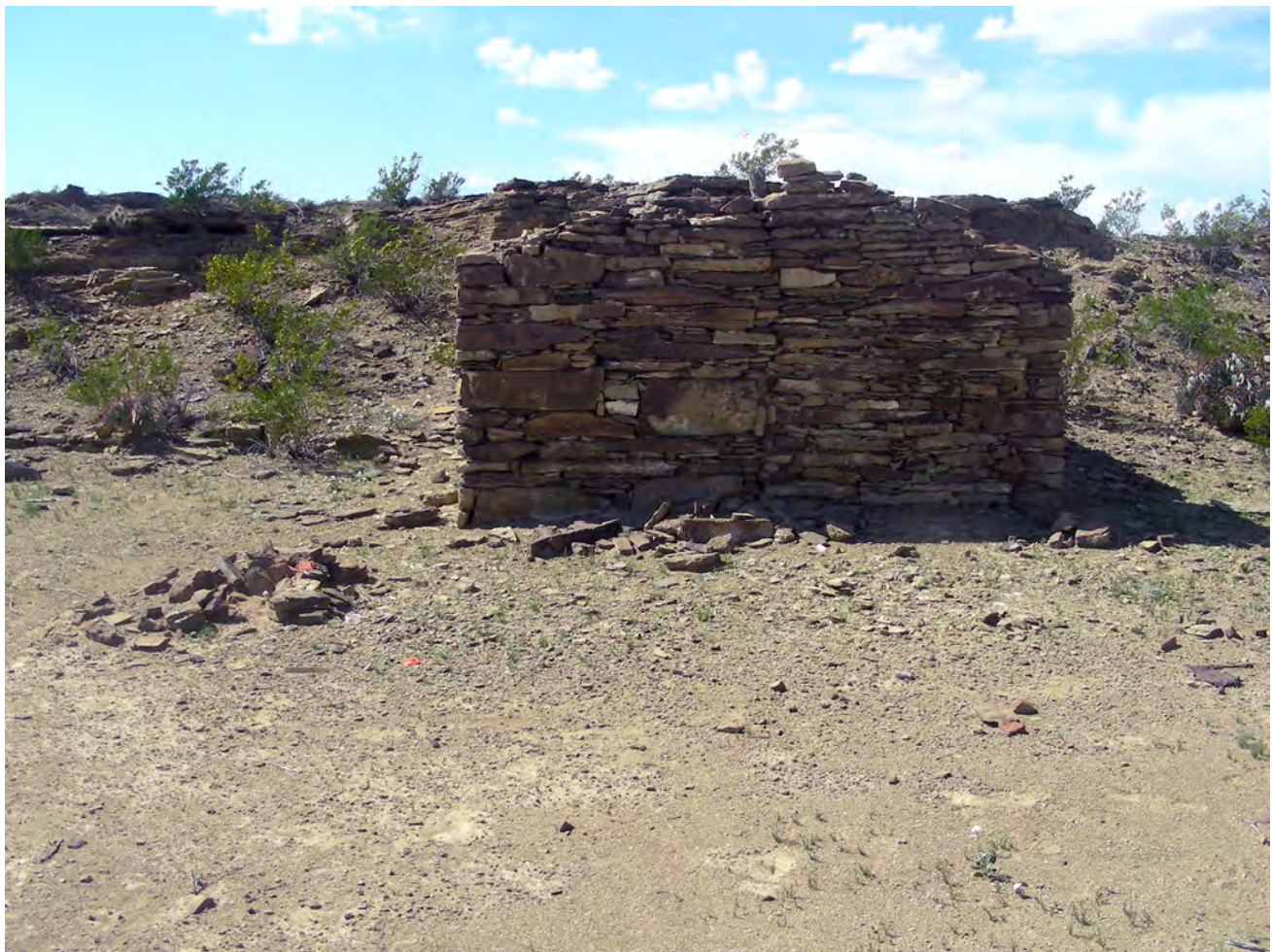
Figure 6-III.10 Mud mortared stone structure at San Vicente (north), BIBE2044 (41BS2261). Photo by B. Dailey.
