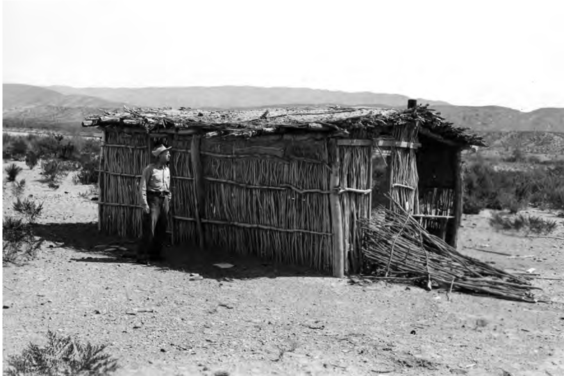
Figure 6-III.20 Historic (1945) photo of jacal structure at Hannold's lechuguilla rope factory; note the use of ocotillo uprights and the remains of daub (earth plaster) along the top of the walls. Courtesy of National Park Service, BBNP.
