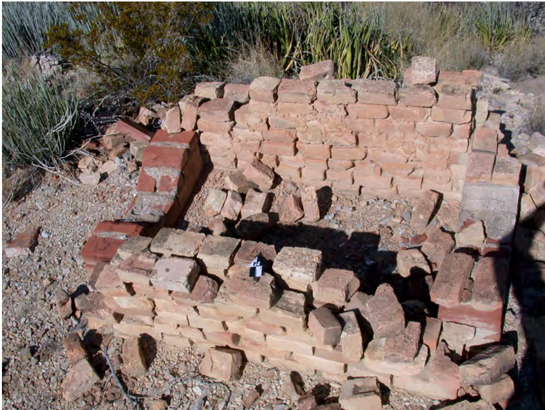
Figure 6-III.35 Foundation for small rotary furnace at BIBE1838 (41BS1764). Photo by B. Dailey.
