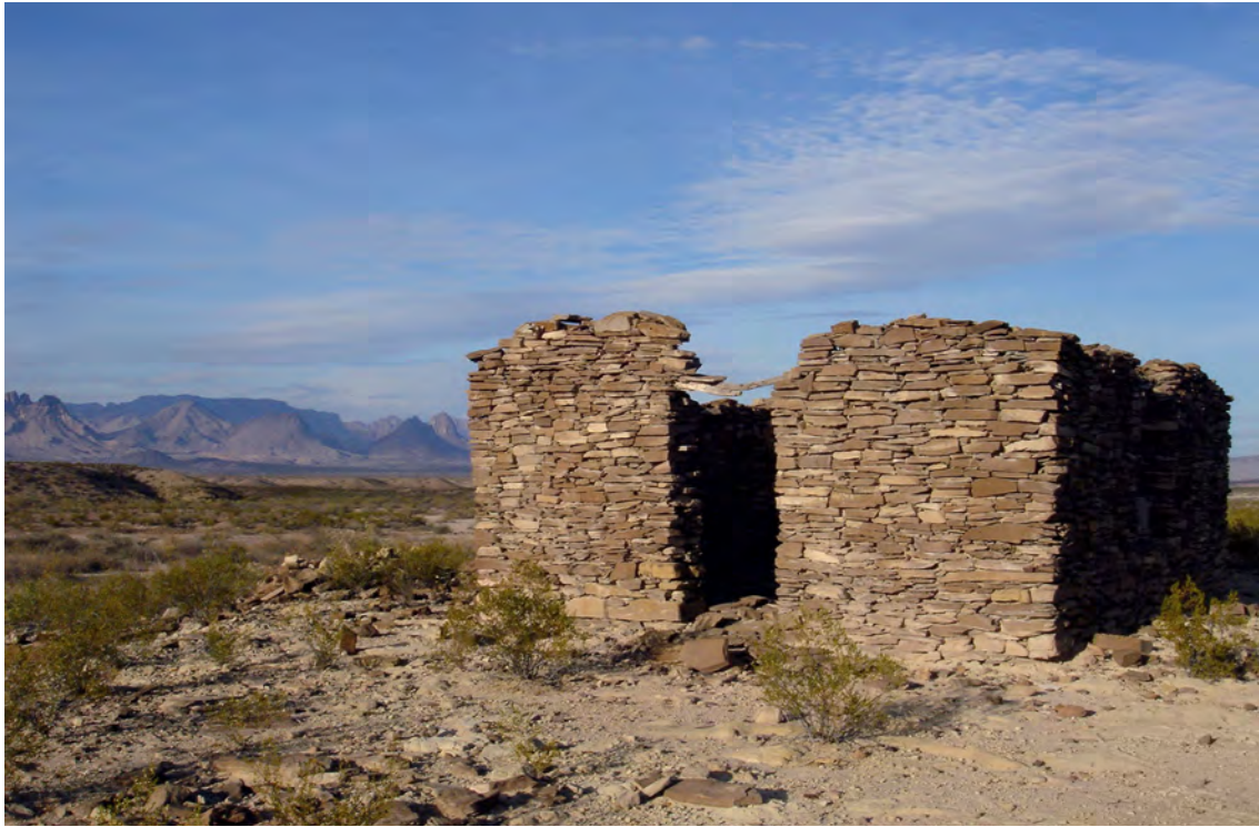
Figure 6-III.19 Mud mortared stone structure at Woodson's (BIBE1594/no trinomial). Photo by J. Bush.
